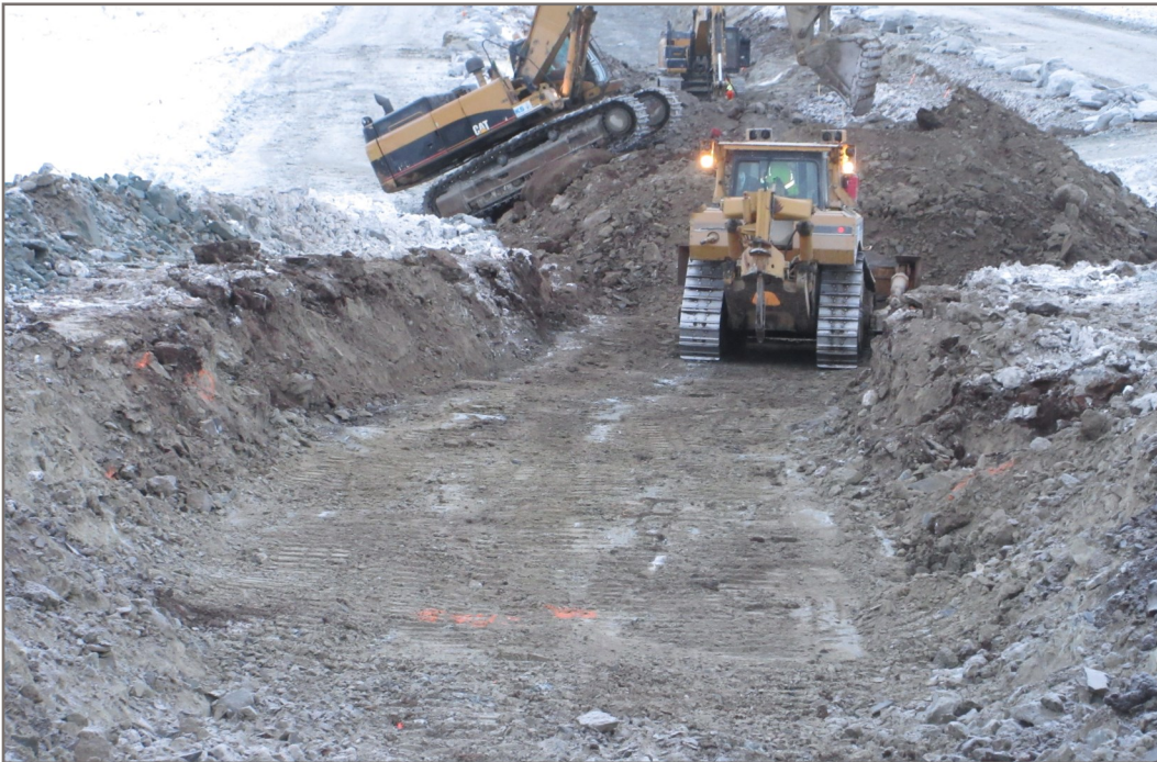
Photo 4: Key trench excavation activities View from Station 0+550 facing down chainage
