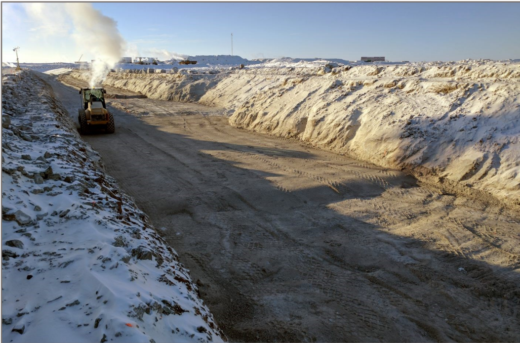
Photo 8: Compacting Type F material placed between Stations 0+450 and 0+475
