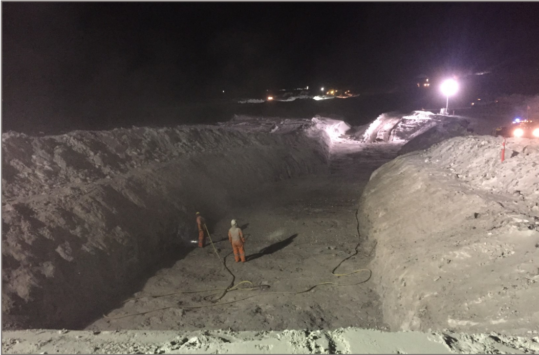
Photo 5: Key trench bottom and slopes final dental cleaning prior to Type F placement View from Station 0+585 facing down chainage
