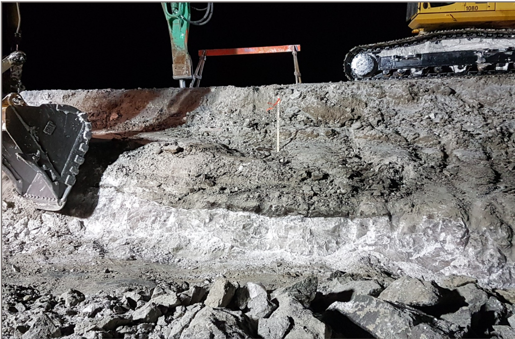
Photo 6: Key trench excavation—massive ground ice on the upstream slope being excavated Between Station 0+492 and 0+507
