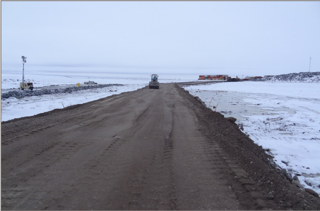
Photo 3: Compacting a lift of Type H material on up stream working platform View from Station 1+280 facing down chainage
