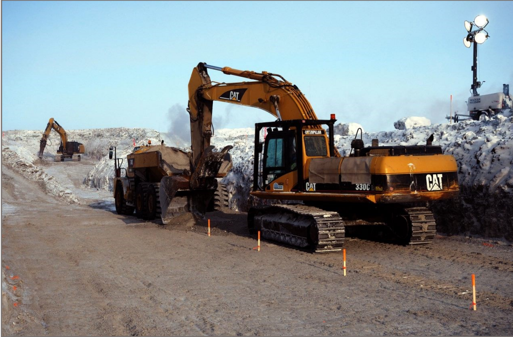
Photo 7: Placing Type F material along key trench bottom around Station 0+470
