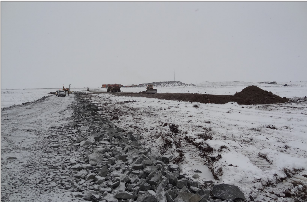
Photo 2: Placing Type H material along the upstream working platform, Type A material on downstream side View from Station 1+300 facing down chainage
