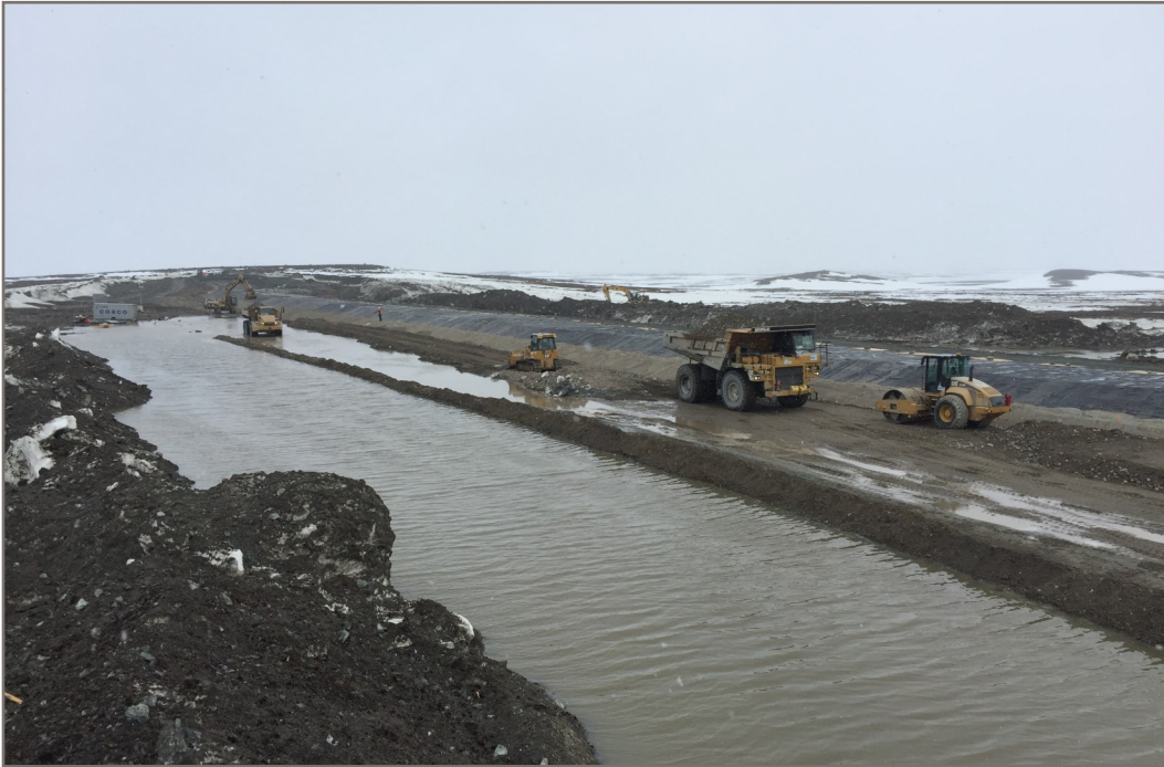
Photo 17: Type H material placement and compaction activities View from Station 1+300 facing up chainage
