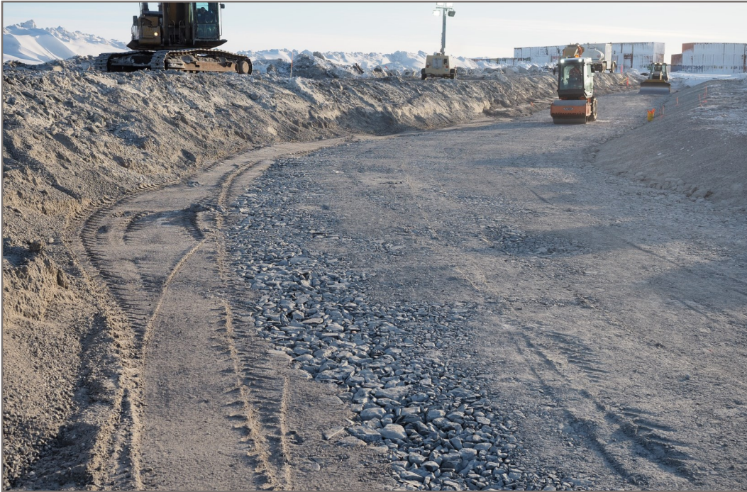
Photo 13: Placing and compacting a lift of transition material in the key trench View from Station 0+200 facing down chainage
