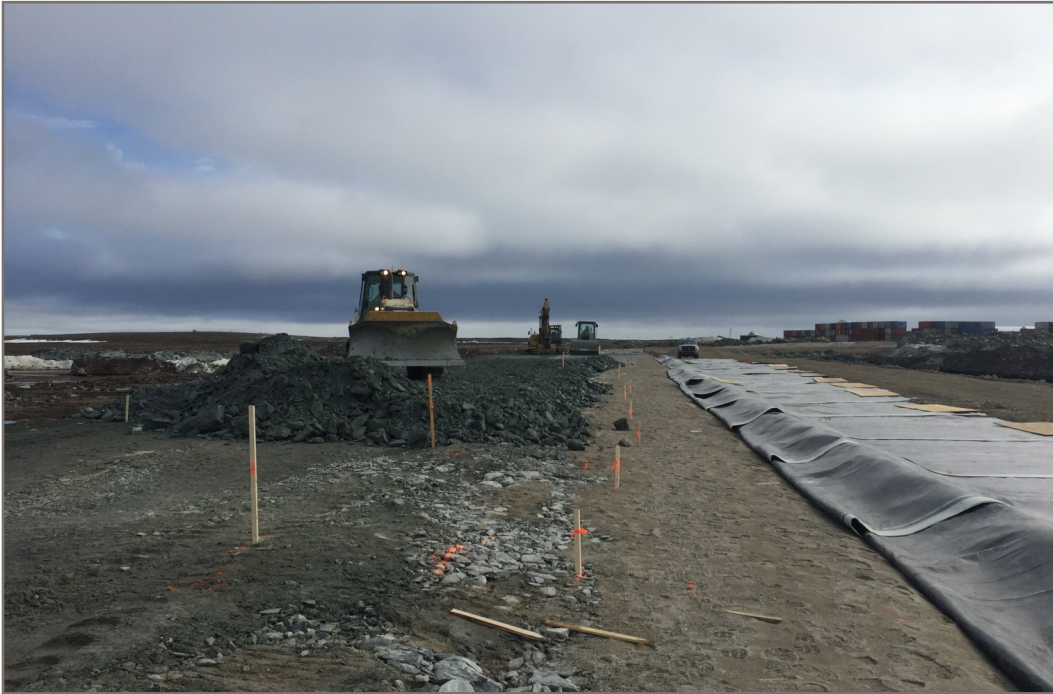
Photo 15: Placing and compacting a lift of Type A downstream shell View from Station 1+360 facing down chainage
