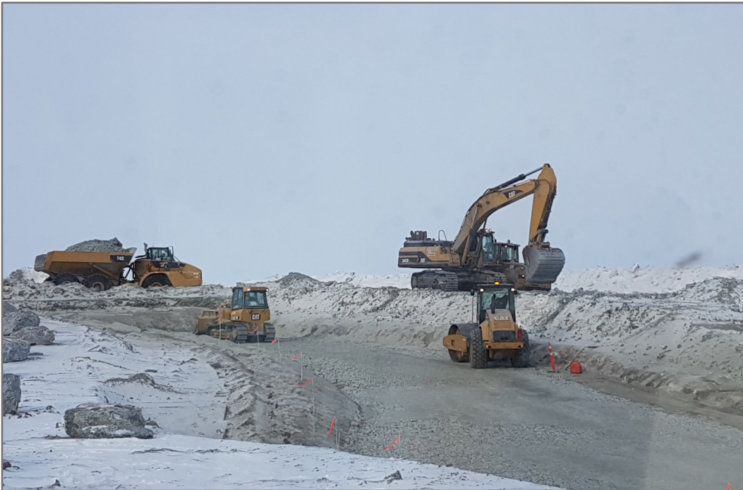
Photo 14: Placing transition material and compacting downstream 20 mm minus fillet zone View from Station 0+545 facing up chainage
