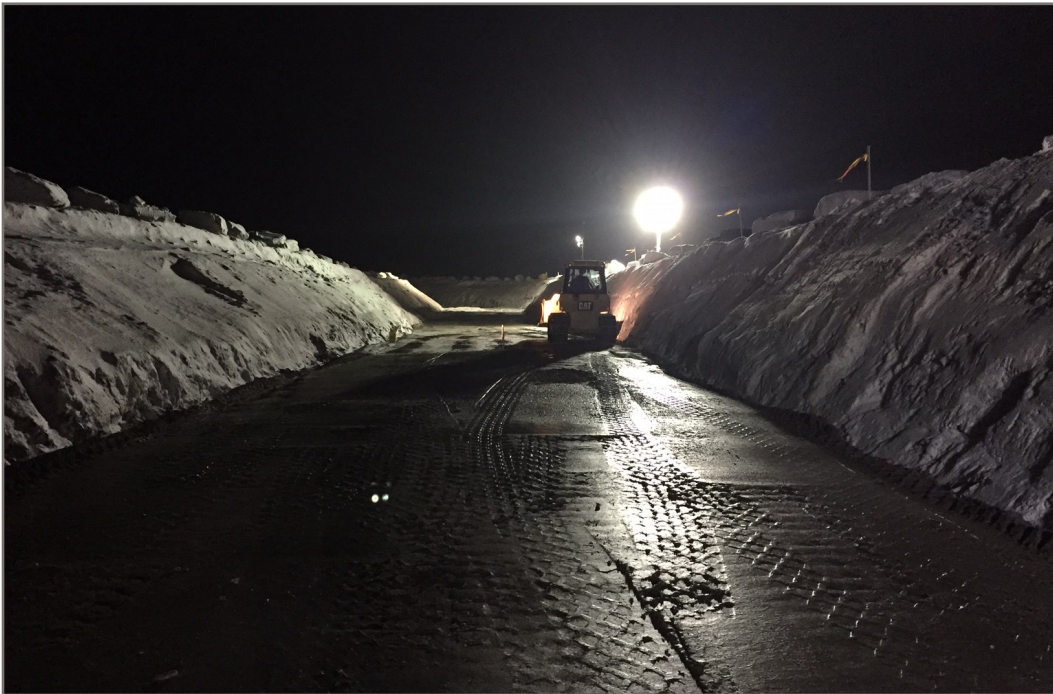
Photo 12: Compacting a lift of Type K material placed on key trench base View from Station 0+250 facing down chainage
