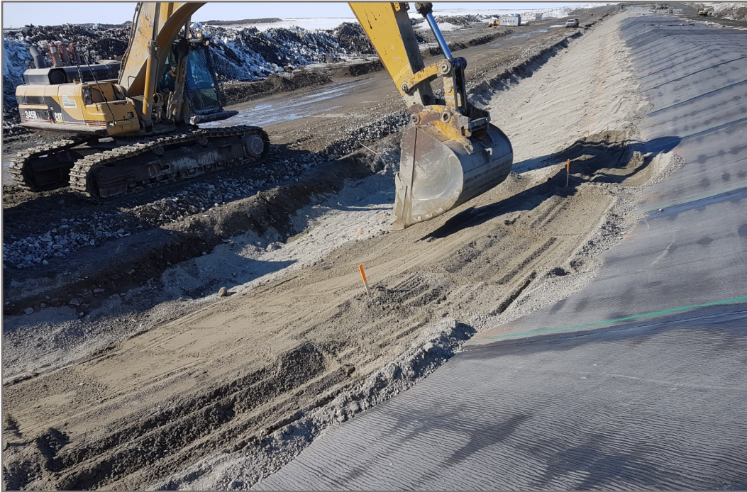
Photo 9: Placing Type F material on top liner from hinge point to Elevation 64.7 View from Station 1+210 facing up chainage
