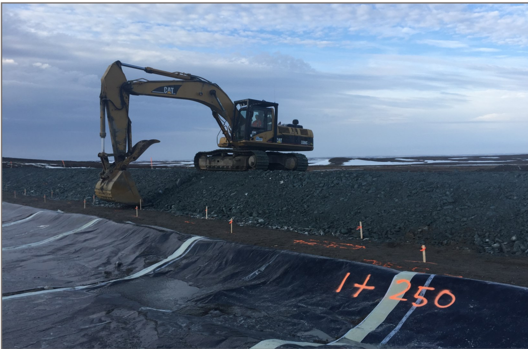
Photo 16: Sloping Type A downstream shell from Elevation 66 m to final elevation (~67 m) View from Station 1+250 facing up chainage
