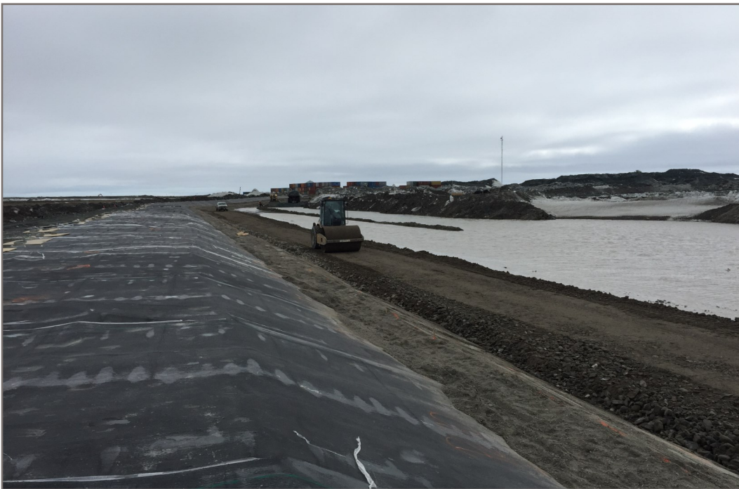
Photo 18: Compacting a lift of Type H material View of from Station 1+250 facing down chainage
