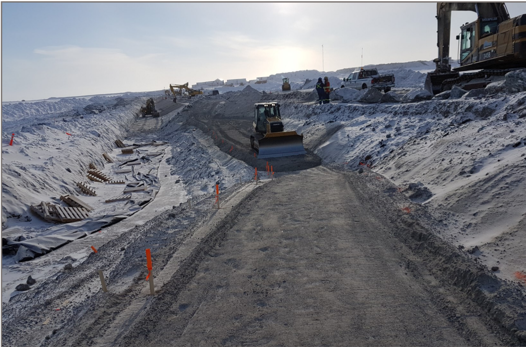
Photo 10: Upstream fillet zone construction - Placing a lift of Type C material View from Station 1+570 facing down chainage
