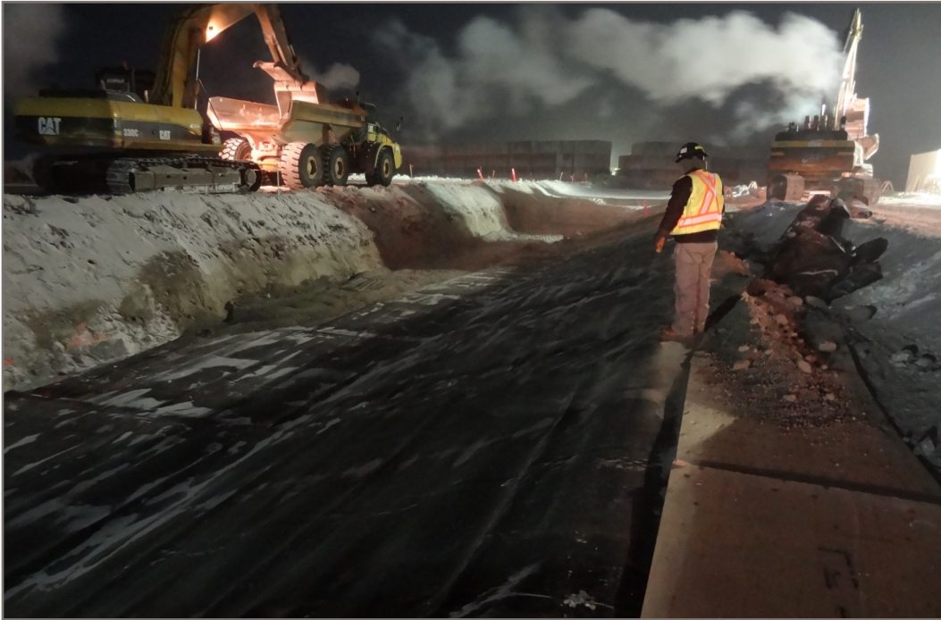
Photo 11: Placing Type F downstream fillet material on liner View from Station 0+050 facing down chainage
