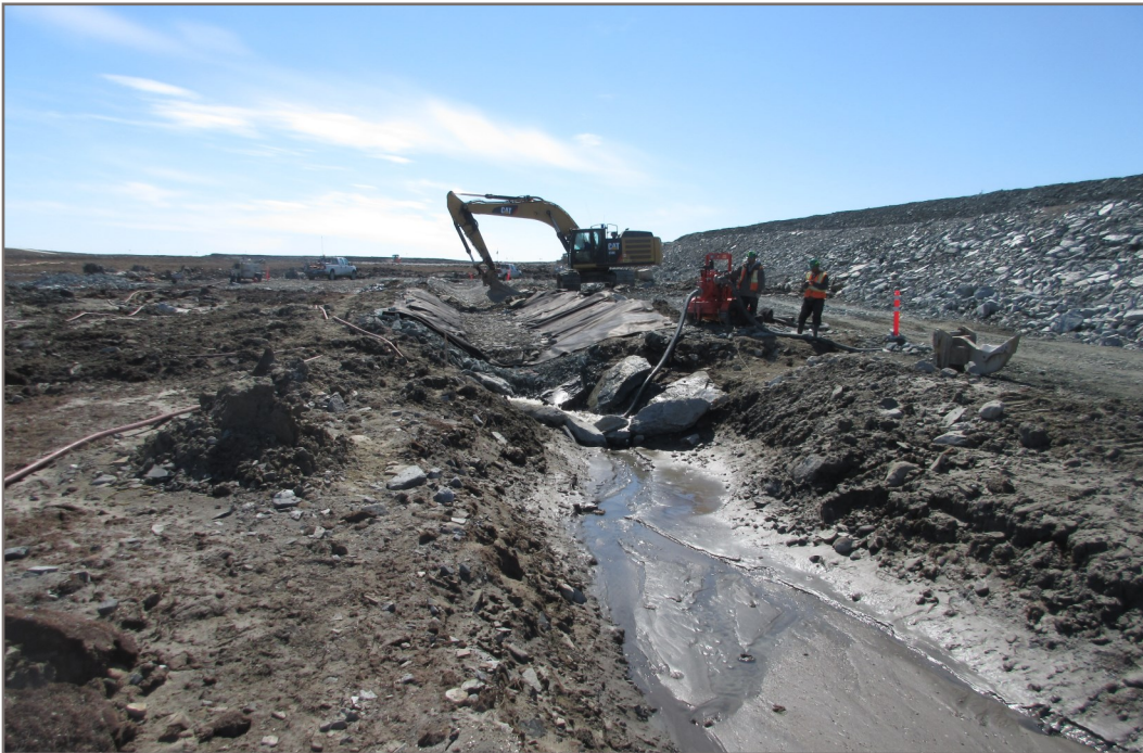
Photo 26: Placing transition material (150 mm minus) on geotextile along North channel View from Station 4+180 facing up chainage
