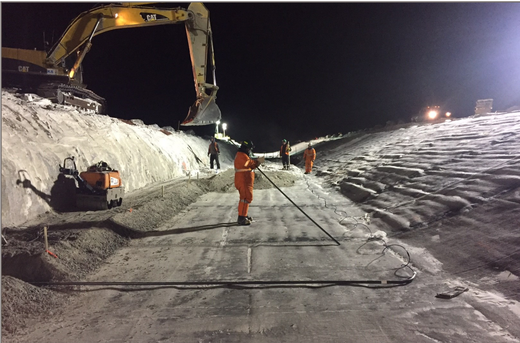
Photo 30: Installing HGTC-4 , cable being inserted in 25 mm ID PVC pipe lying on liner between Station 0+420 and 0+470
