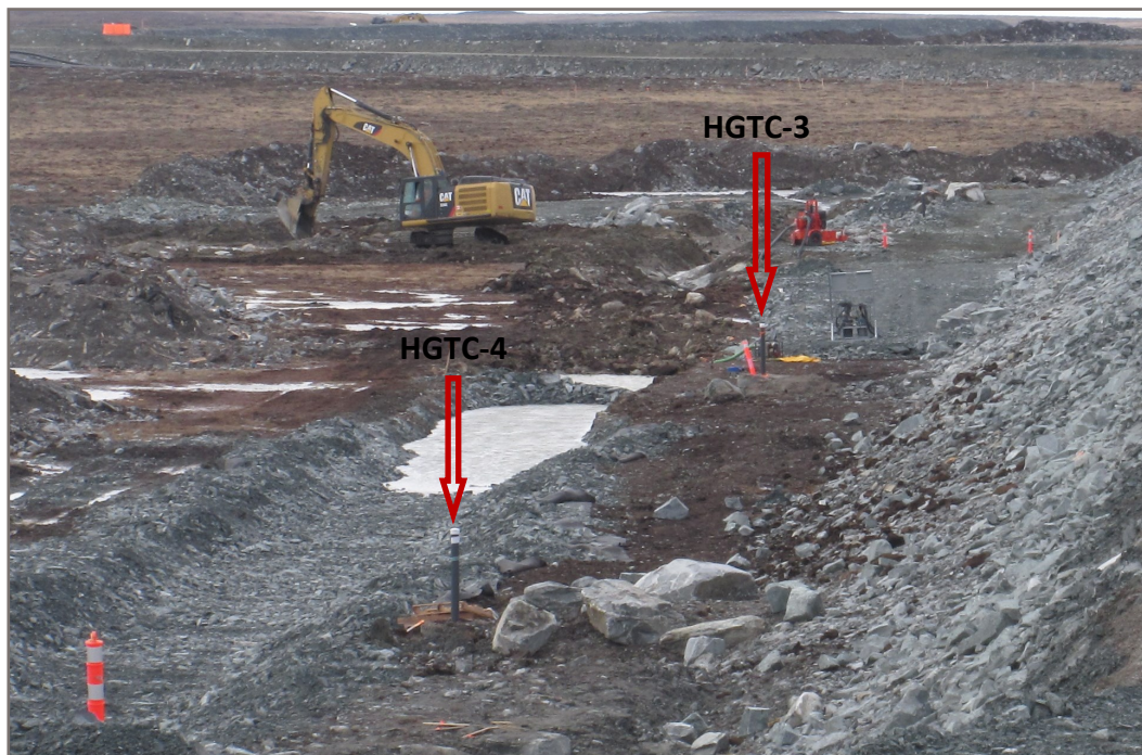
Photo 32: Arrows pointing at terminals for HGTC-3 and HGTC-4
