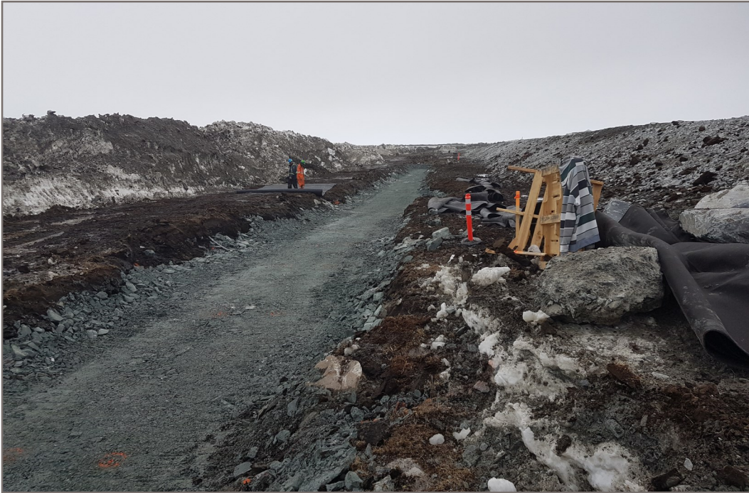
Photo 25: Compacted Type A material along North water collection channel alignment View from Station 4+060 facing up chainage
