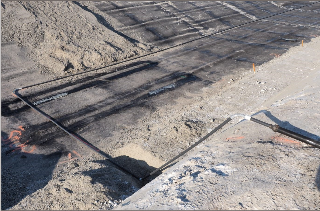
Photo 31: HGTC-2 is in the 25 mm I.D. PVC pipe shown– terminal out of the key trench downstream side at Station 0+290
