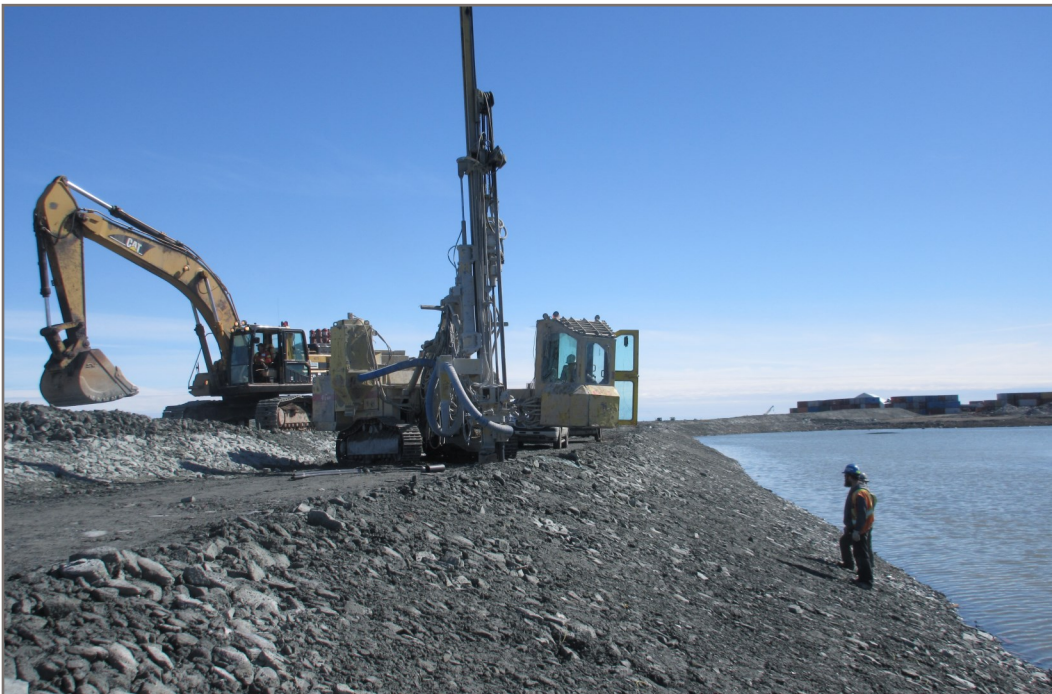
Photo 34: Drilling to install VGTC-3
