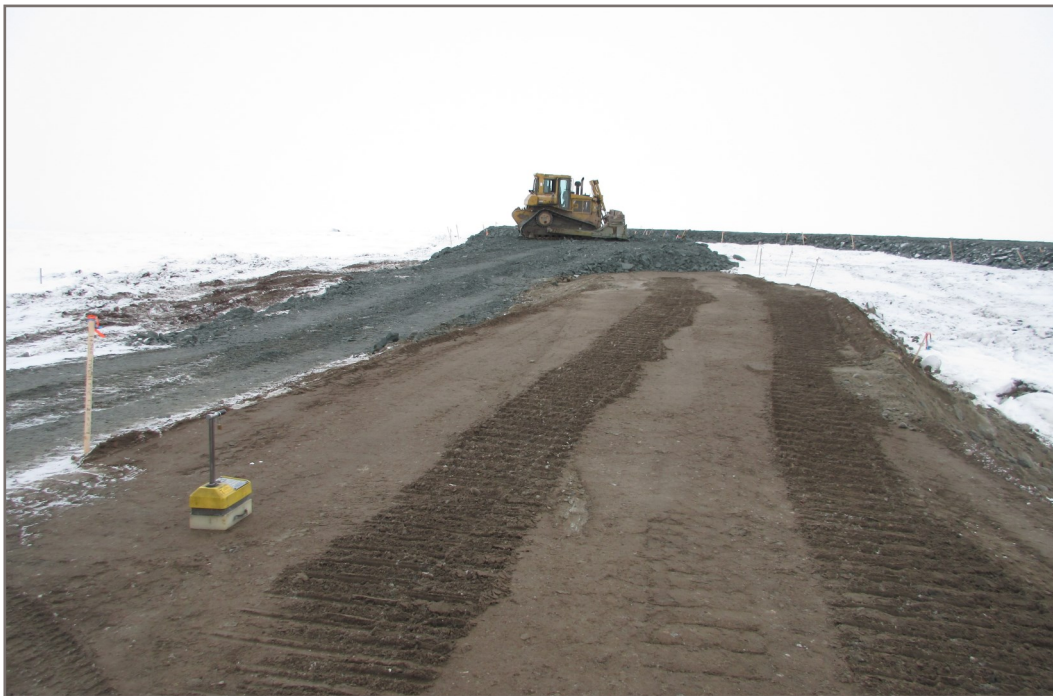
Photo 38: Compaction test on a lift of Type H material around Station 1+565
