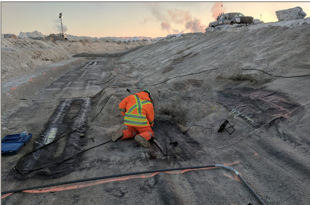
Photo 55: Finalizing Patches R4, R5 and R6
