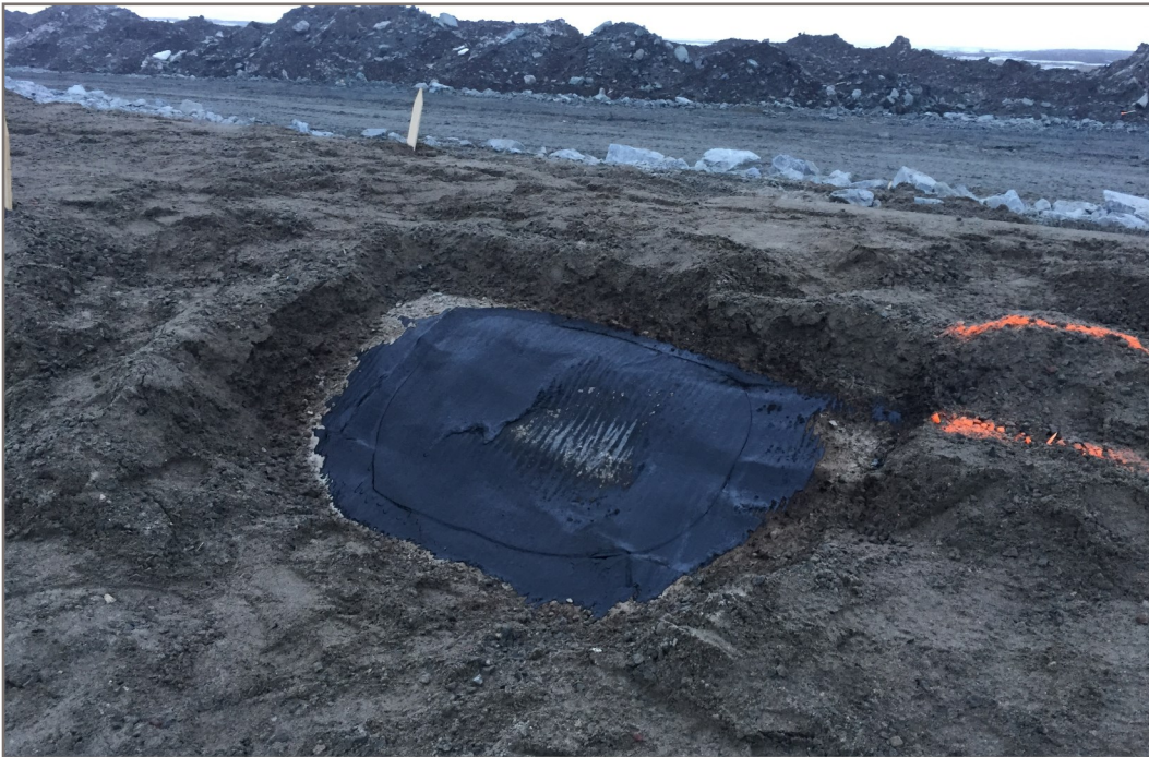
Photo 51: Patch completed on punctured Top Liner at Station 1+040
