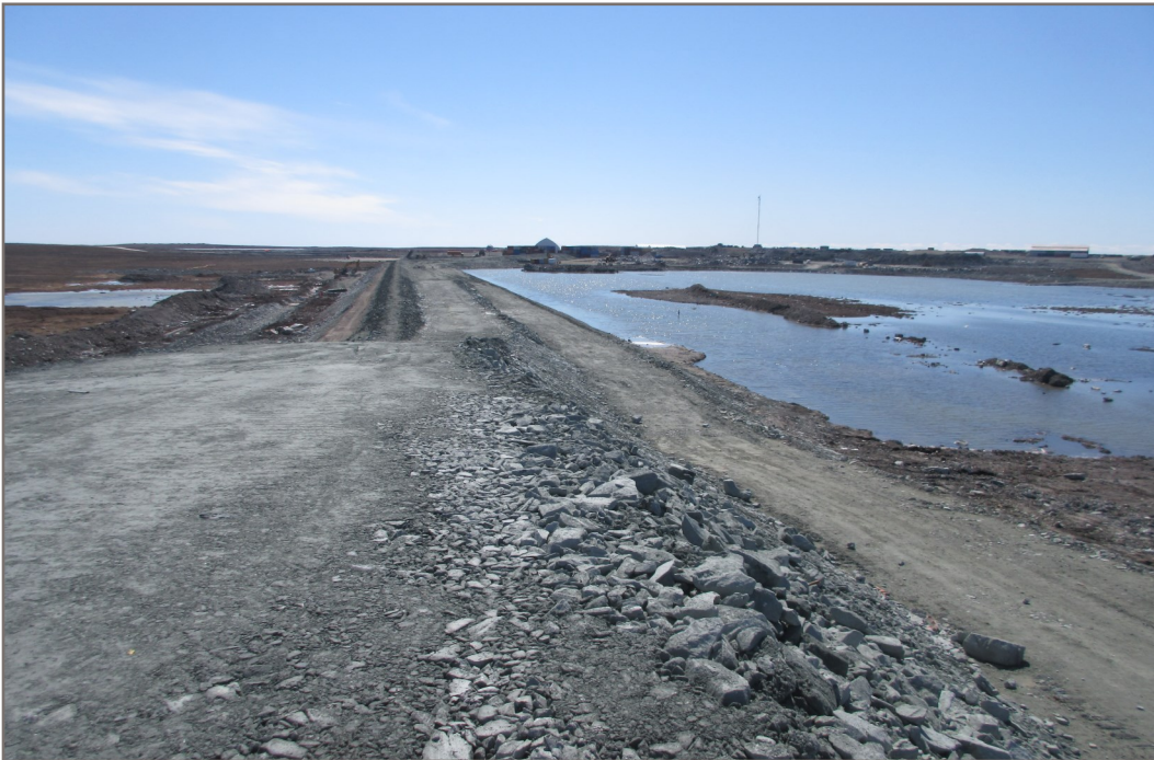
Photo 59: View of completed Dike D-CP1 from Station 1+585 facing upstream side
