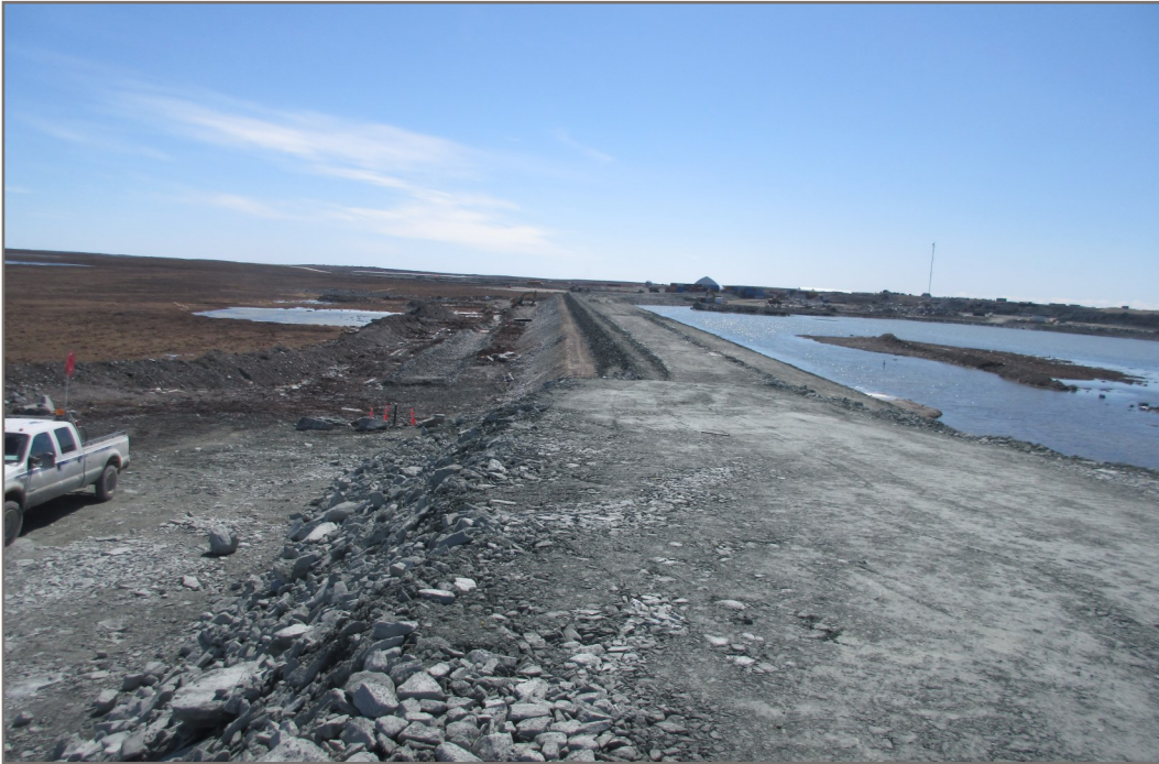
Photo 58: View of completed Dike D-CP1 from Station 1+585 facing downstream side
