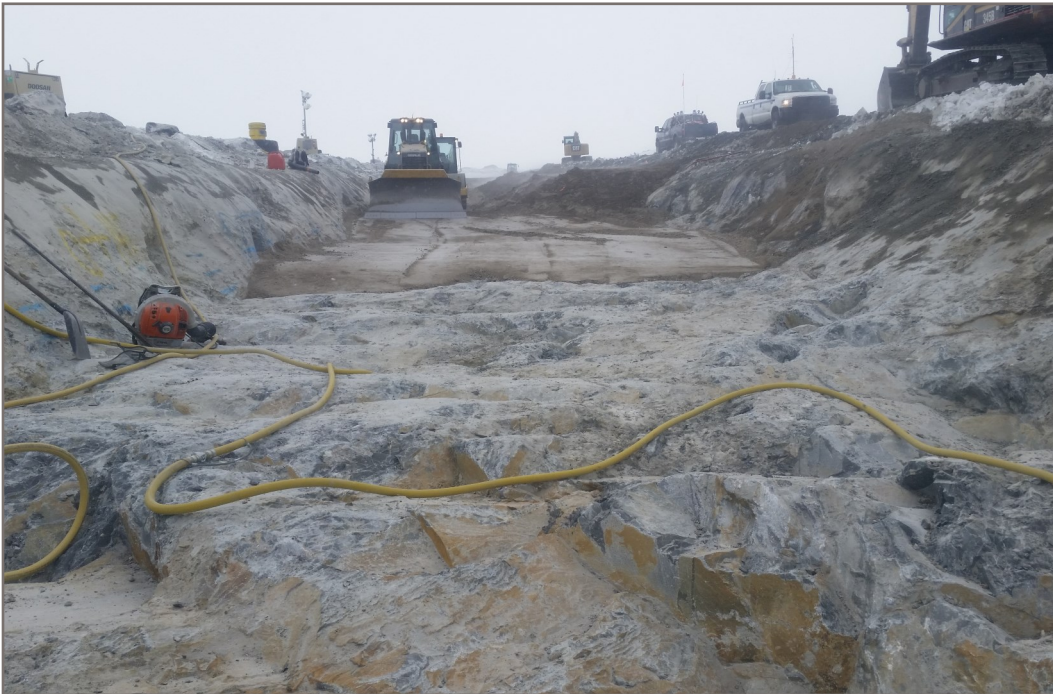
Photo 8: Type F material placement View from Station 0+155 facing down chainage
