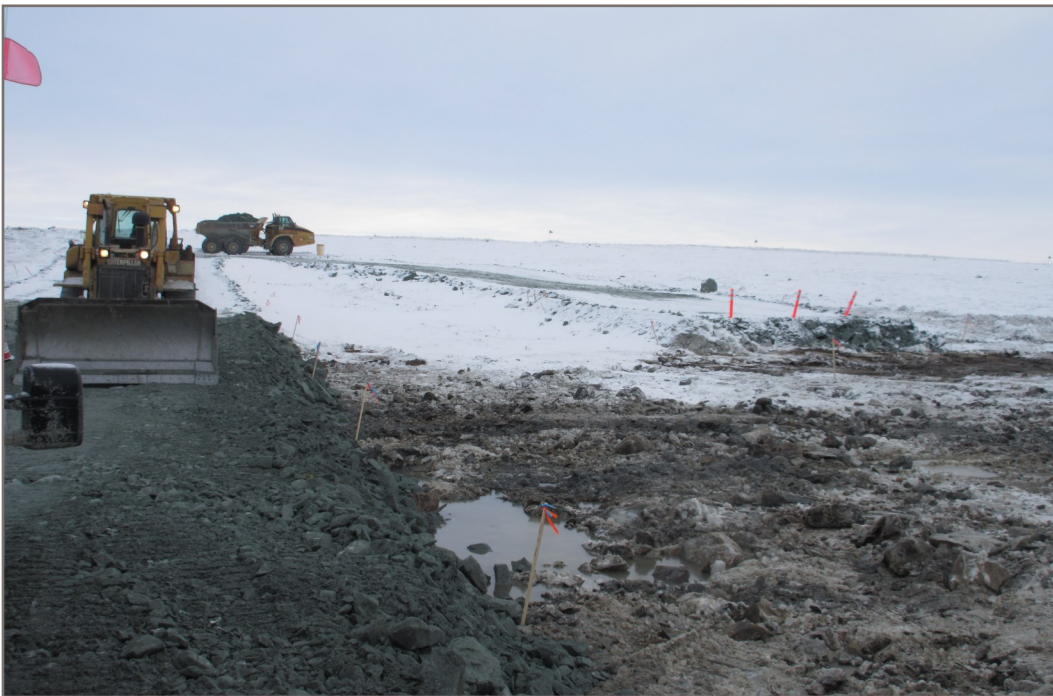
Photo 2: Placing first lift of Type A material (working platform) on the upstream side View from Station 1+280 facing up chainage
