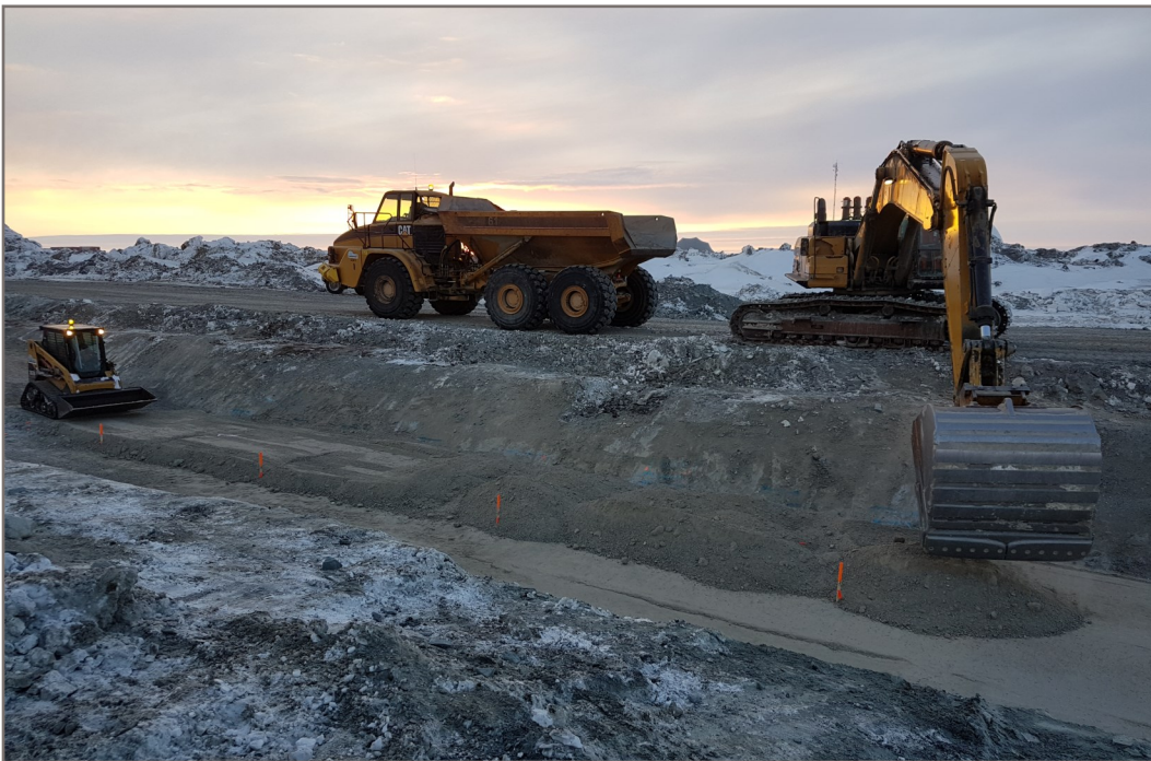
Photo 10: Placing first lift of upstream fillet Type F material View from Station 0+100 facing down chainage
