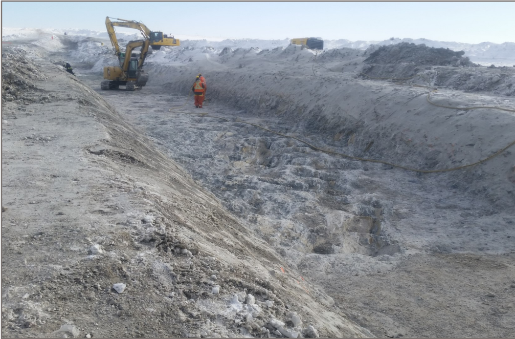
Photo 7: Final dental cleaning on key trench bottom prior to placing Type F material View from Station 0+30 facing up chainage
