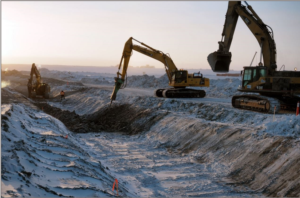
Photo 5: Key trench sloping and hammering View from Station 0+190 facing up chainage
