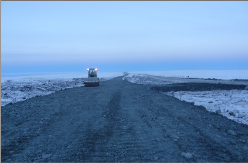
Photo 3: Compaction of first lift of Type A material on the upstream working platform View from Station 1+090 facing up chainage
