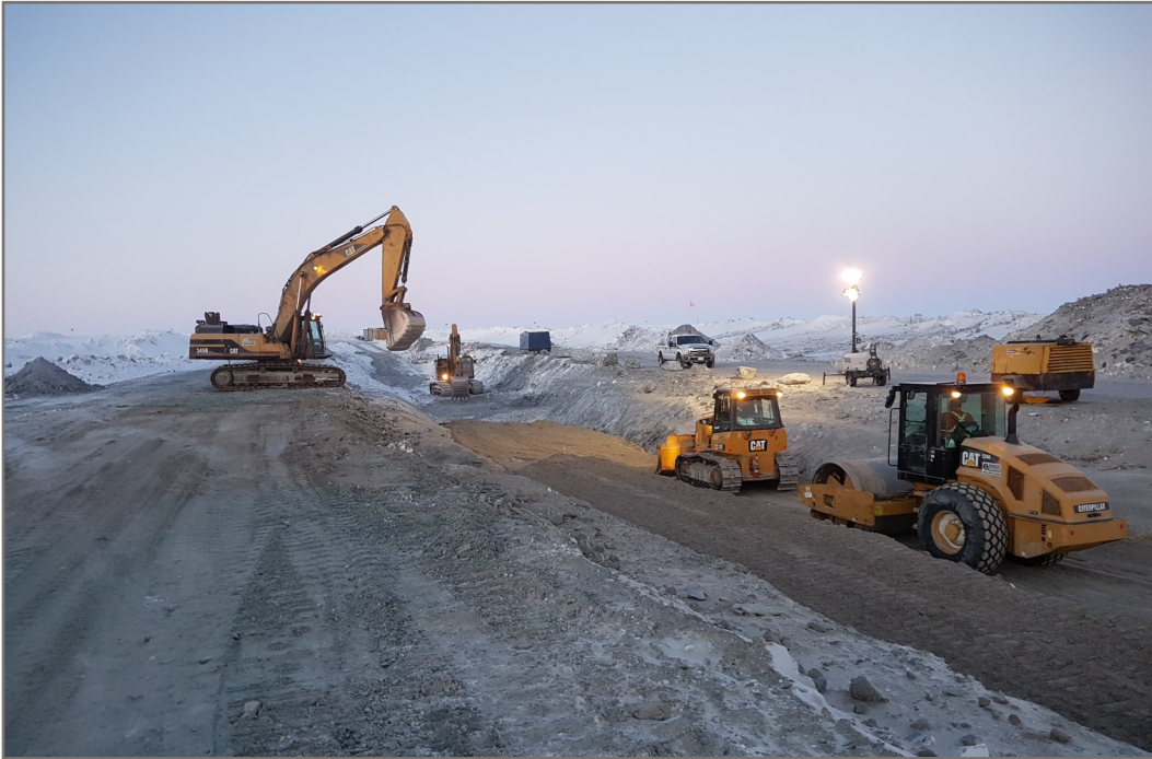
Photo 9: Type F material placement and compaction View from Station 0+180 facing up chainage
