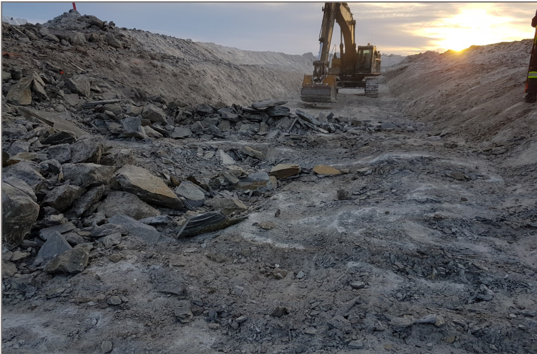
Photo 6: Key trench - bedrock encountered at ~1.4 m depth below original ground surface Between Stations 0+040 and 0+060
