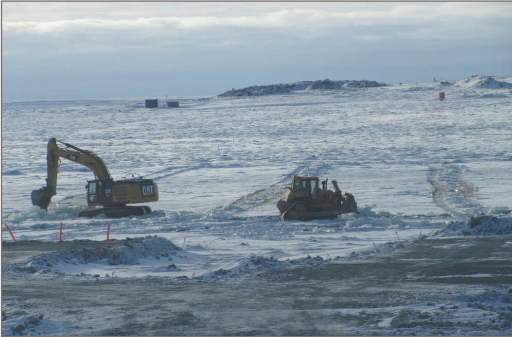
Photo 1: Pushing Lake Ice, snow, boulders and cobbles from dike's footprint to construct working platform (first lifts of dike's shell) View from Station 1+300 facing down chainage
