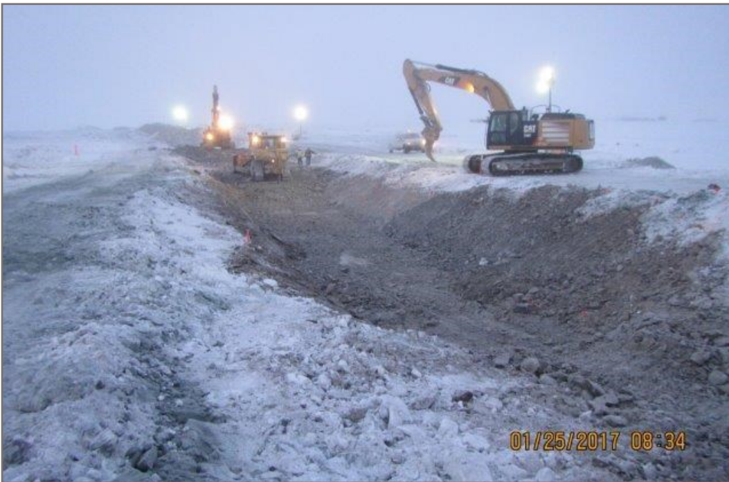
Photo 4: Key trench excavation between Stations 0+210 and 0+290
