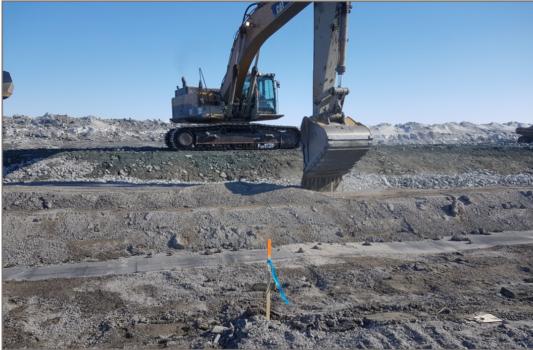
Photo 15: Excavator placing Type C below liner bedding material on dike upstream slope At Station 1+240
