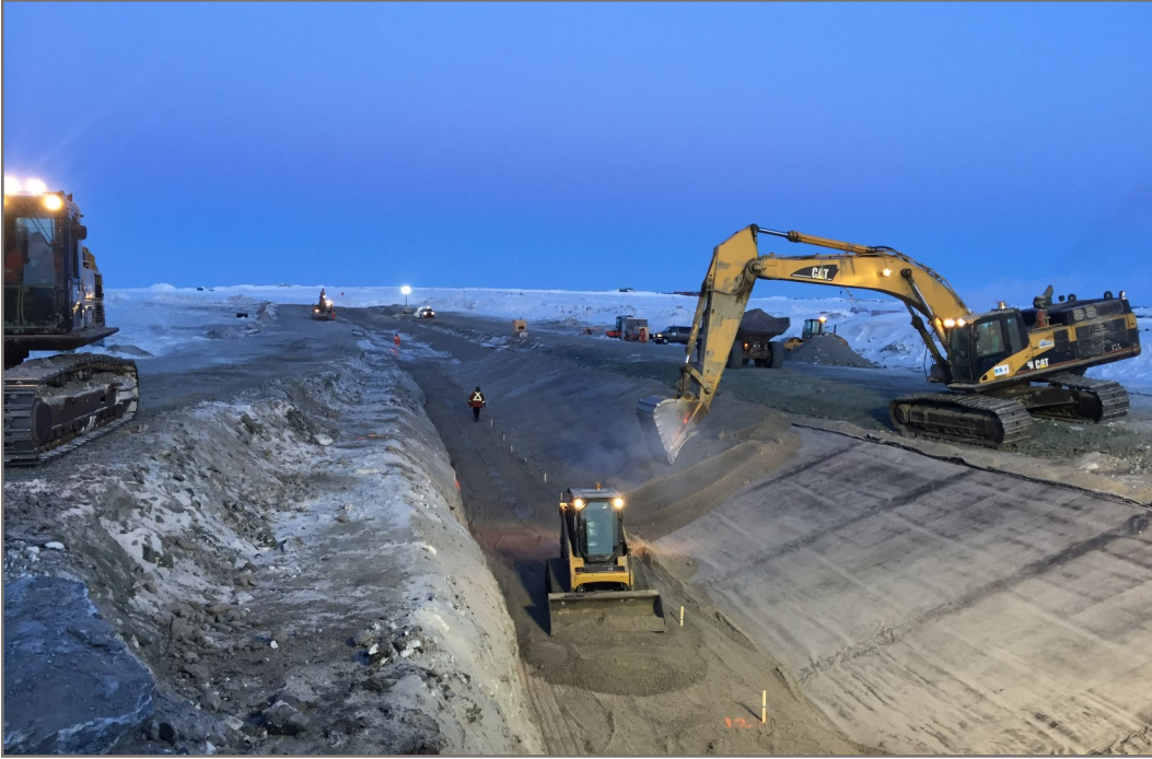
Photo 13: Excavator placing first lift of Type C over liner on upstream slope Skid Steer placing second lift of Type C over liner on key trench base View from Station 0+245 facing down chainage
