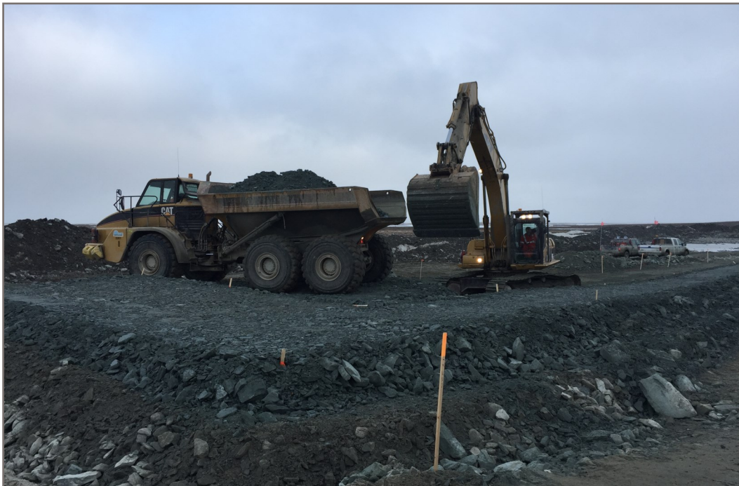
Photo 18: Placing Type A thermal cover around Station 1+320
