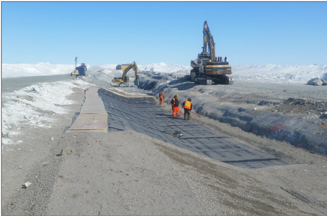
Photo 12: Placing downstream fillet Type F material View from Station 0+135 facing up chainage
