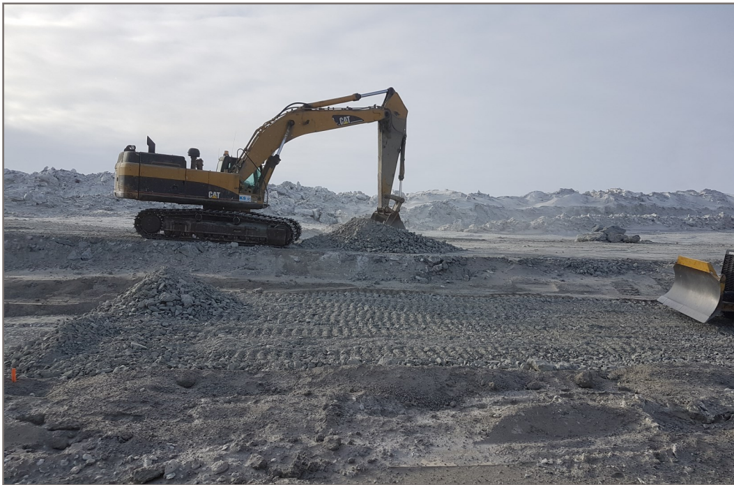
Photo 14: Placing and spreading a lift of Type B material around Station 0+200 Excavator placing and D5 dozer spreading
