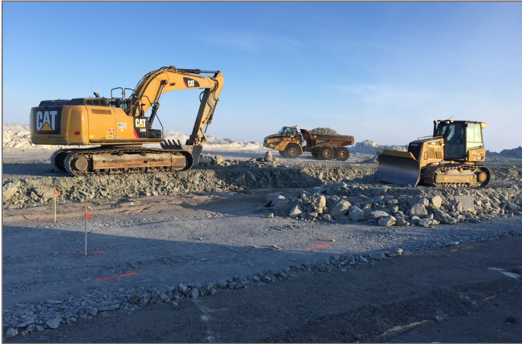
Photo 17: Placing Type A material View from Station 1+040 facing down chainage
