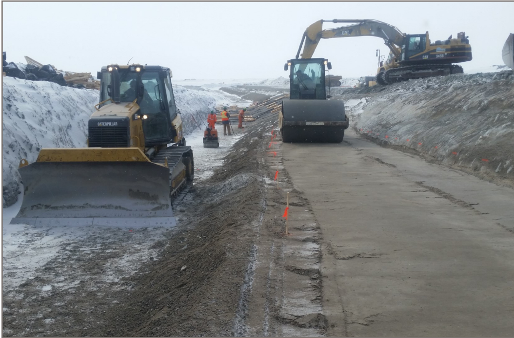
Photo 11: Compacting a lift of Type C upstream fillet View from Station 0+285 facing down chainage
