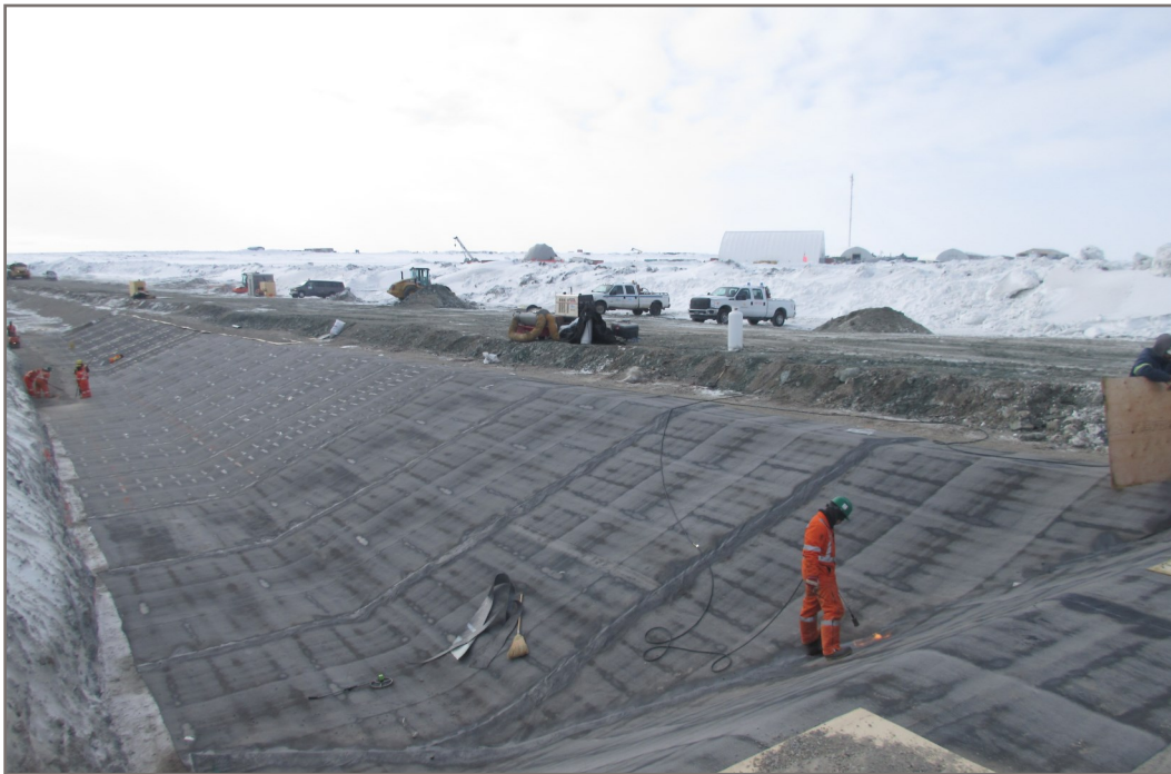
Photo 20: Placed Phase 1 liner View from Station 0+285 facing down chainage
