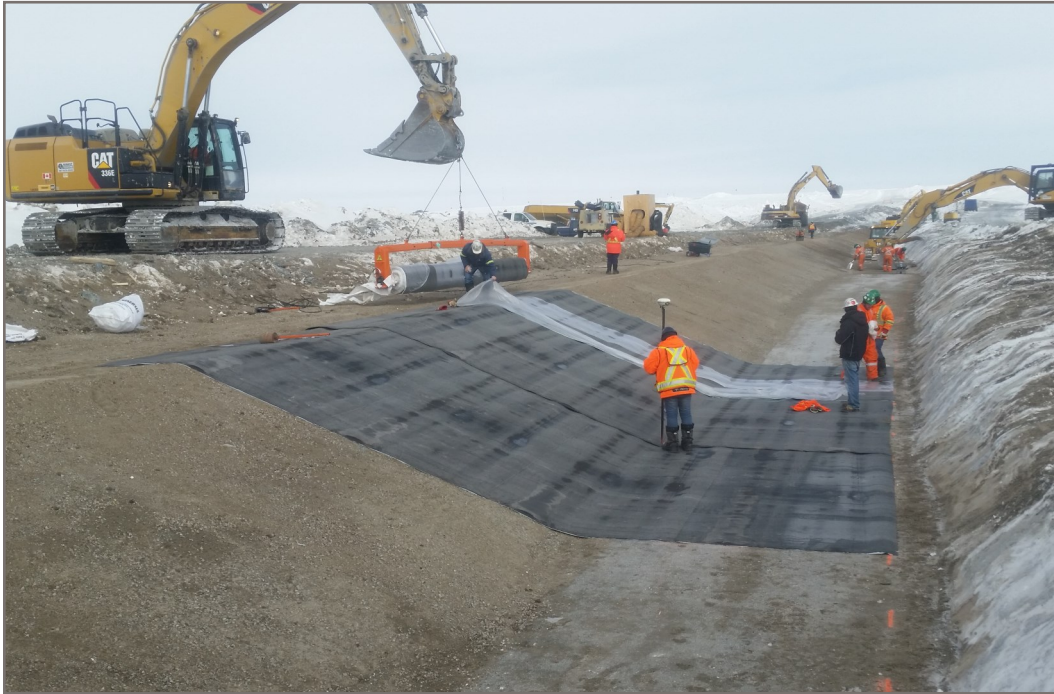
Photo 19: Deploying a Phase 1 liner panel View from Station 0+003 facing up chainage
