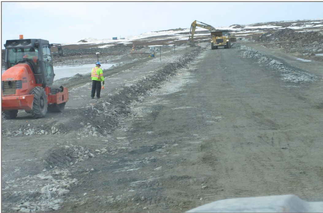
Photo 16: Placing and compacting Type B crest material View from Station 1+260 facing down chainage
