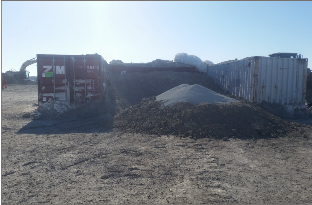
Photo 31: QC monitoring the mixing of Bentonite-Augmented (Type F) material Bentonite placed on Type C material waiting to be mixed by the IT62 CAT loader
