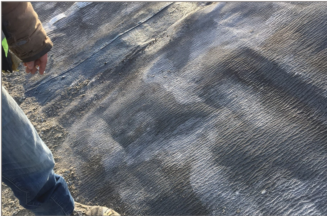
Photo 42: Area of water behind liner—granular material is Type F over liner at hinge point Approximate Station 1+190
