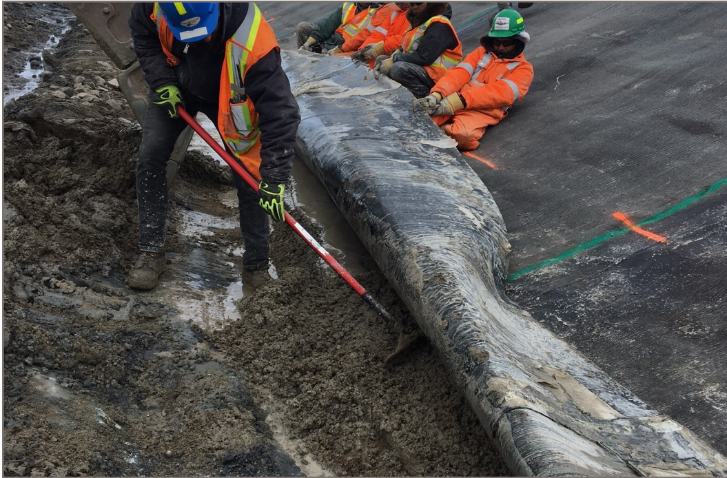
Photo 41: Removal of saturated Type F under liner at hinge point Approximate Station 1+210 facing up chainage
