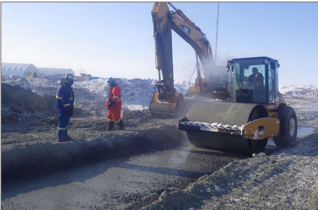
Photo 2: Compaction of watered lift at DP1-A. April 10, 2016.
