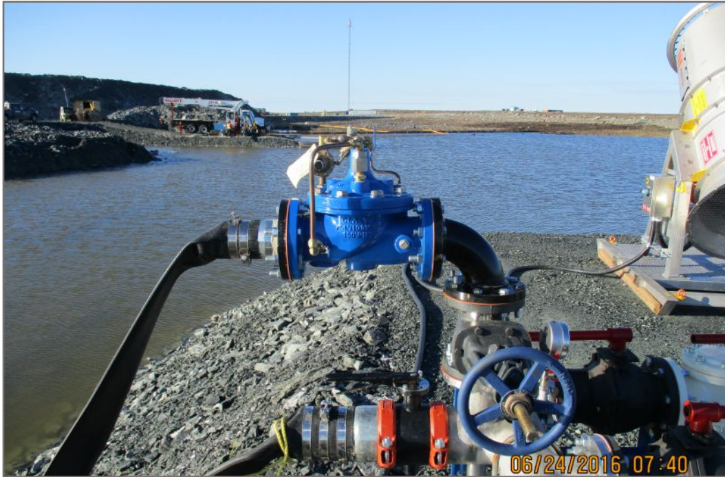
Photo 13: Pressure relief valve. June 24, 2016.
