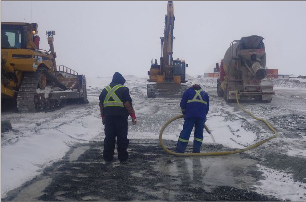
Photo 5: Watering a lift of Material 0-30 at DP3-A. April 15, 2016.
