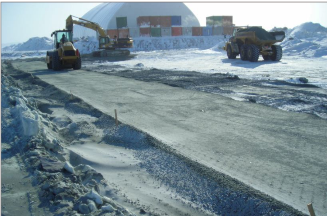
Photo 6: Compaction of the core material at DP3-A. April 22, 2016.
