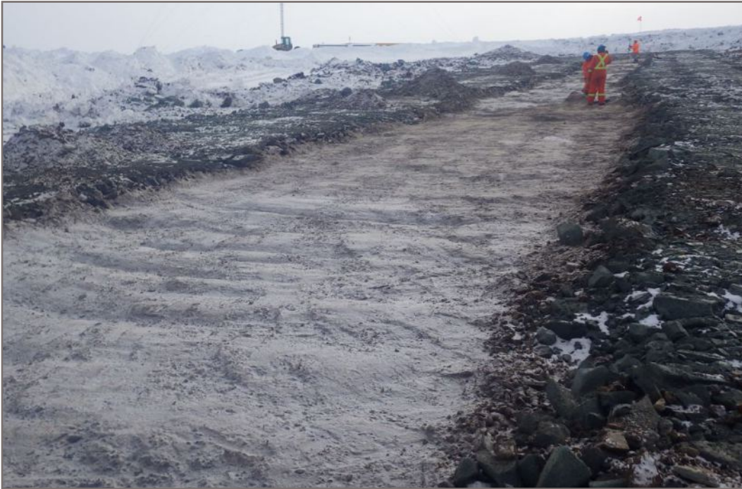
Photo 1: Prepared foundation at DP1-A (looking south). March 30, 2016.
