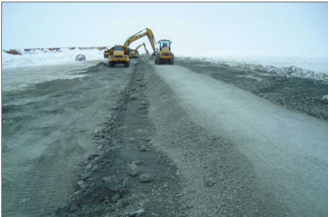
Photo 7: Compaction of core material at DP3-A (looking north). April 24, 2016.
