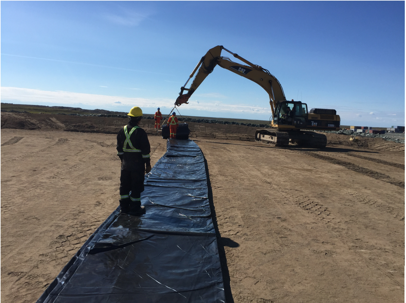
Photo 2: Geotextile membrane installation
