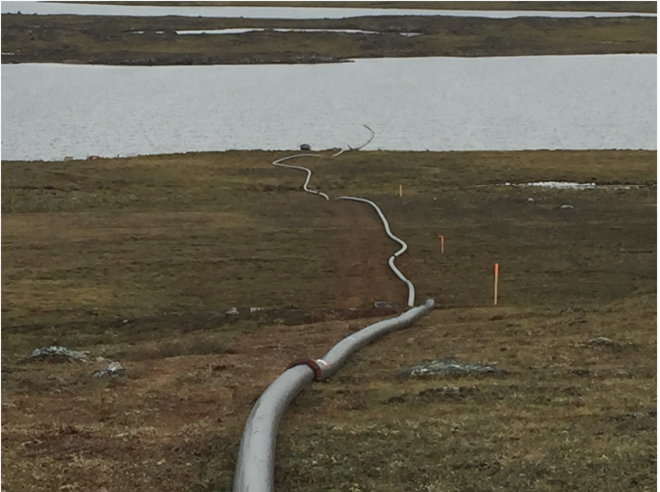
Photo 6: Meliadine Lake treated water discharge from the MWTP
