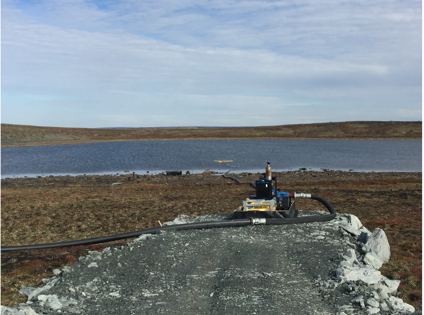
Photo 5: Pond H17 raw water intake pump pad to the MWTP
