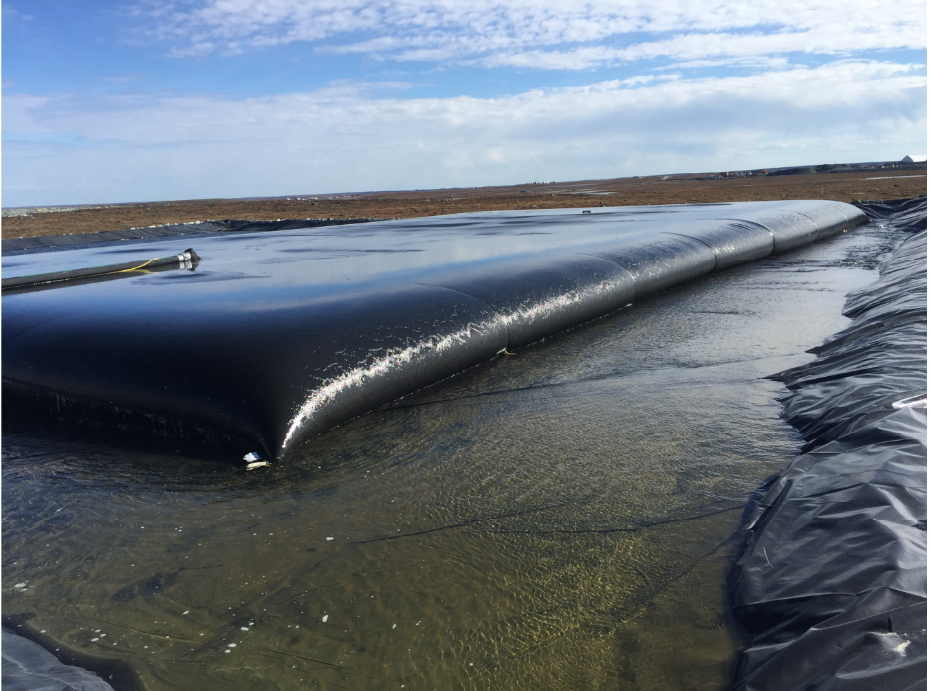
Photo 4: Geotubes filtration technology in operation
