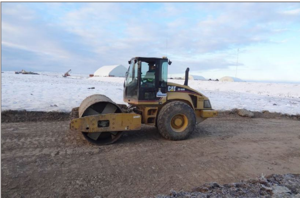
Photo 16: Compaction of till with roller
