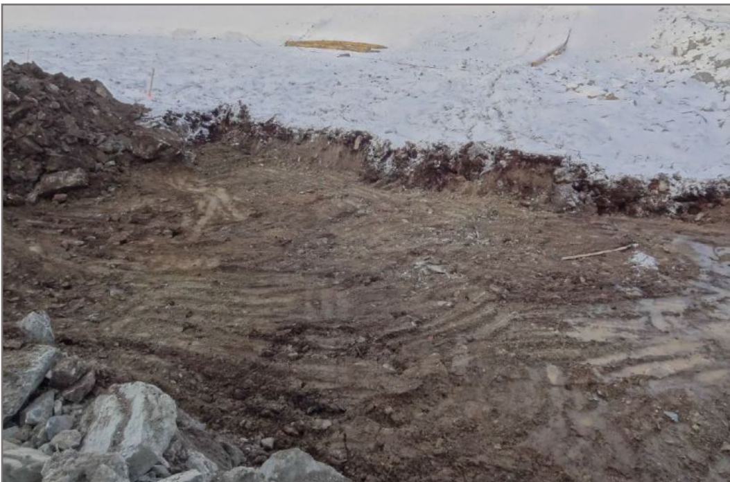
Photo 14: Berm trench after excavation of organics
