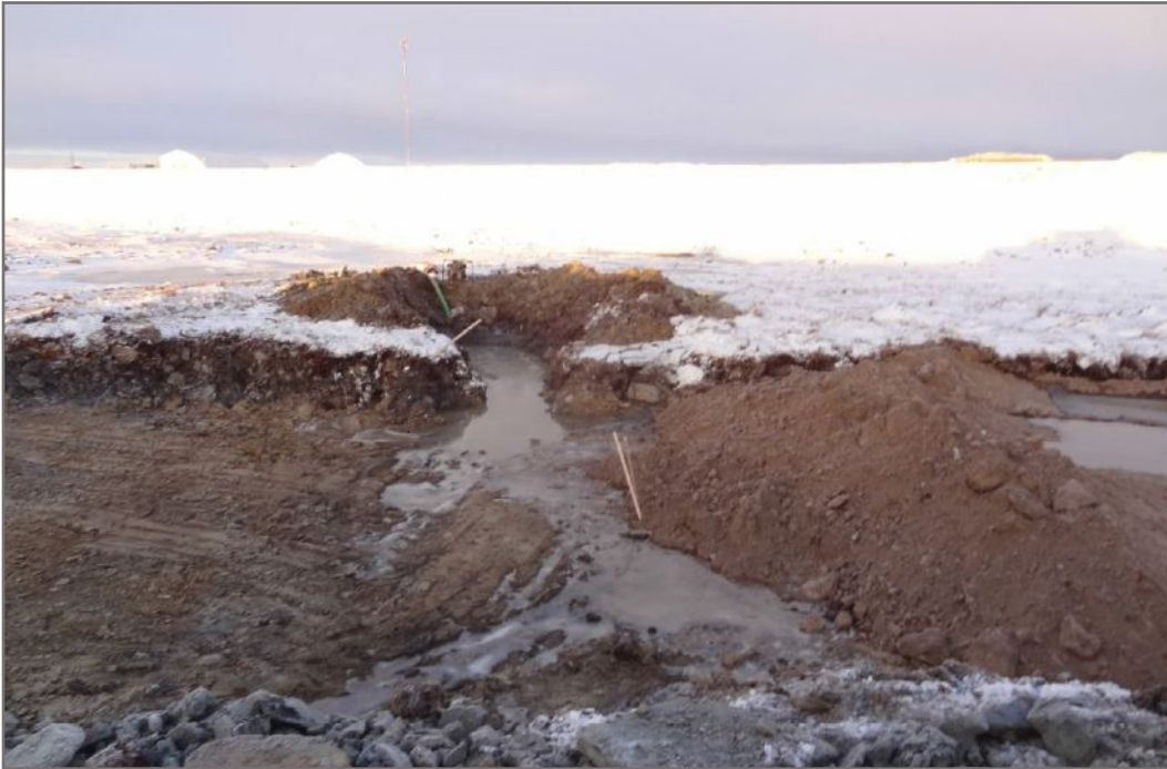
Photo 17: Temporary sump (west side)
