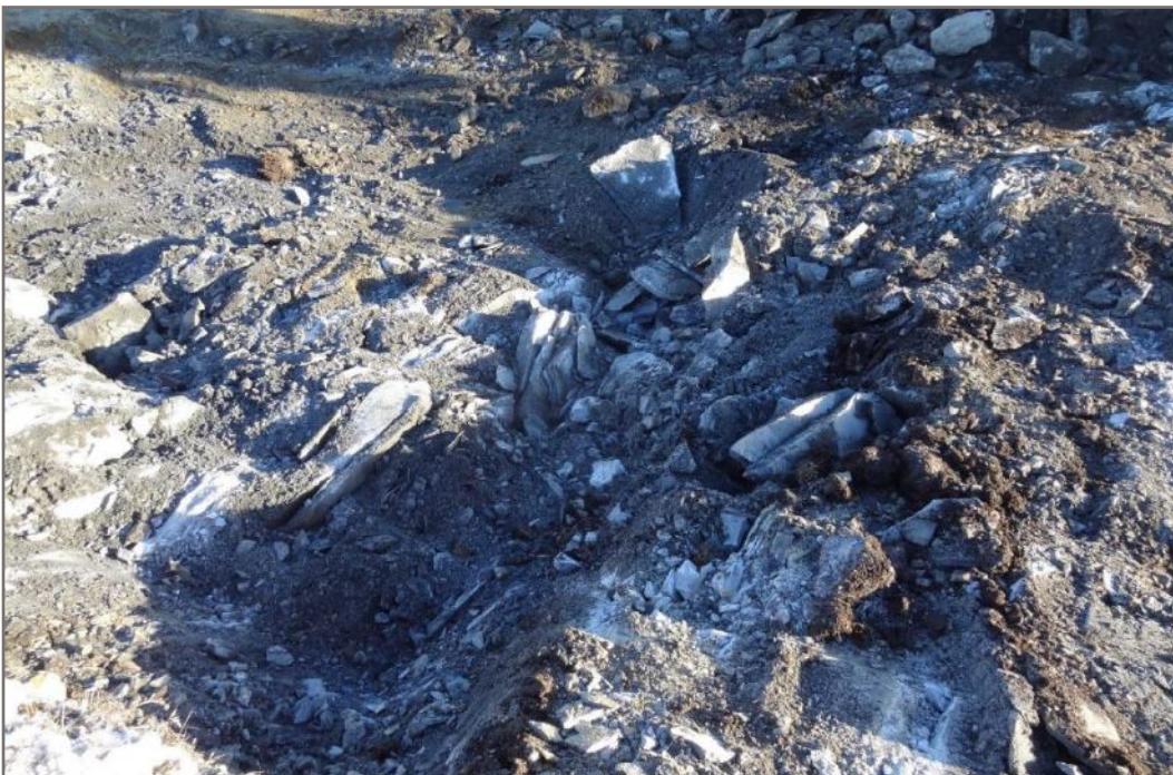
Photo 18: Bedrock encountered during trench excavation
