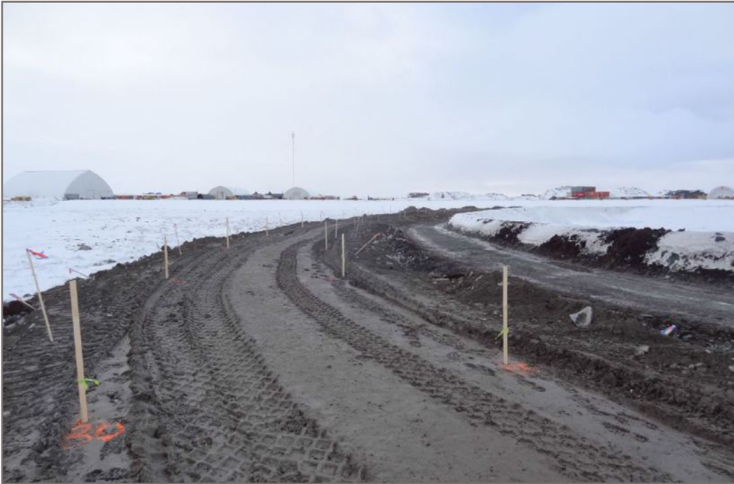
Photo 19: Crest and toe stakes showing overbuild, approx. chainage 0+190 (looking west)
