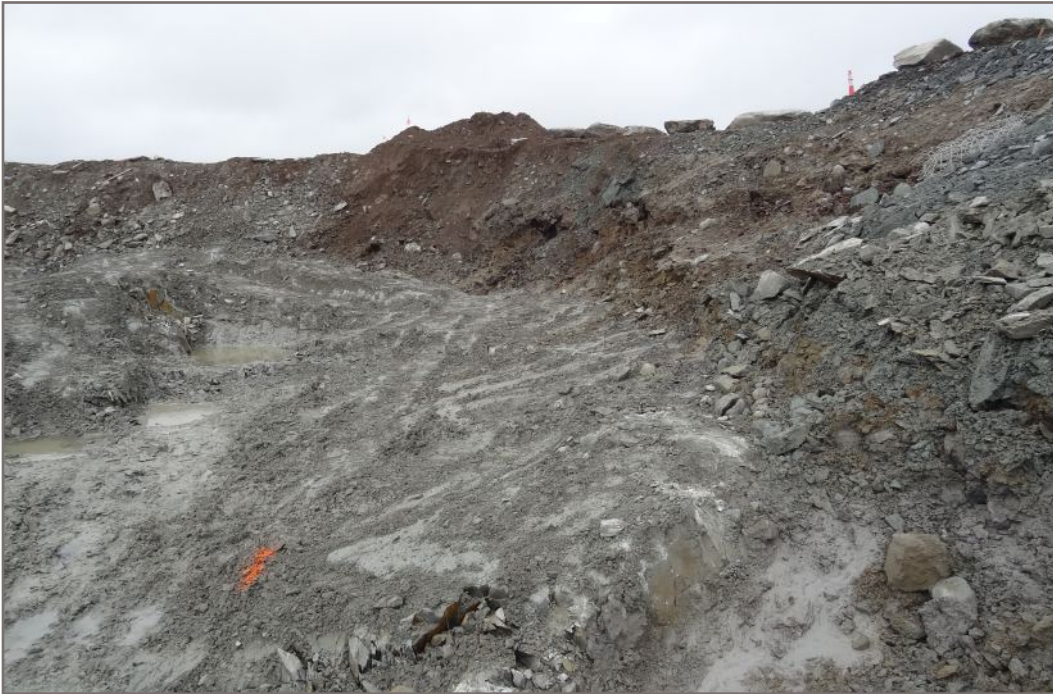
Photo 7: Over excavation of thawed overburden (northwest corner)
