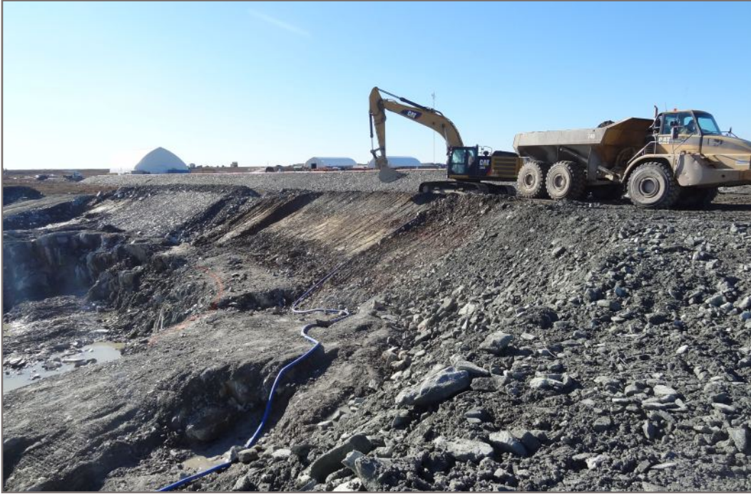
Photo 3: Shaping overburden slope (west wall)
