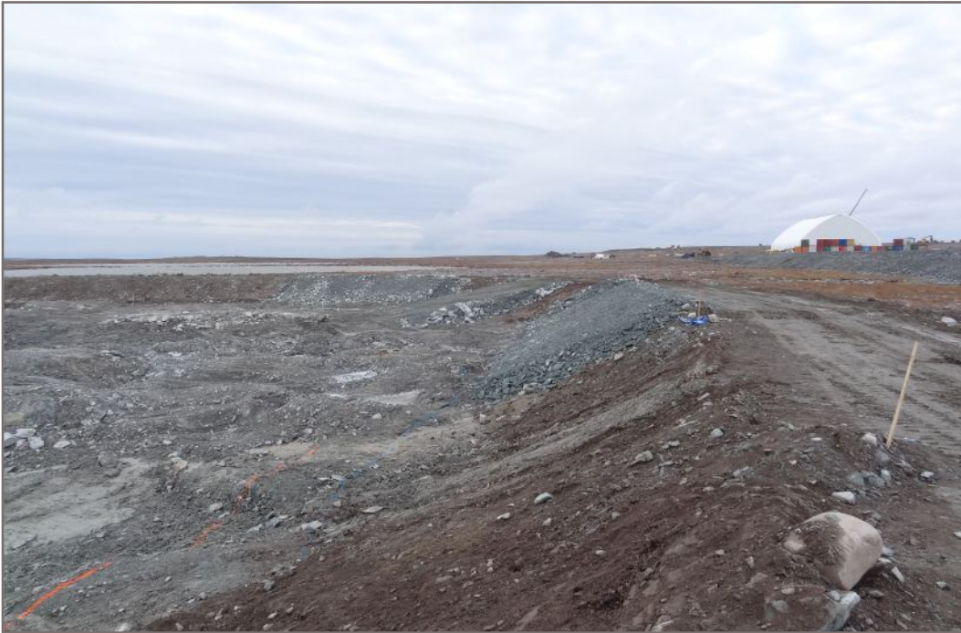
Photo 1: Excavation of overburden down to bedrock surface (looking south)
