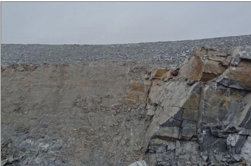
Photo 12: Excavating to stable foliation plane (south wall)
