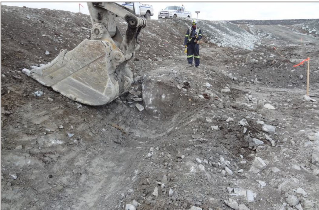
Photo 2: Shaping overburden slope (south wall)
