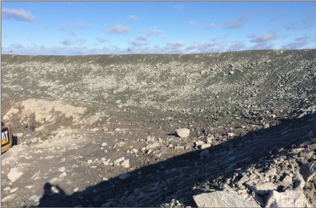
Photo 5: Completed ROM fillet (north wall)
