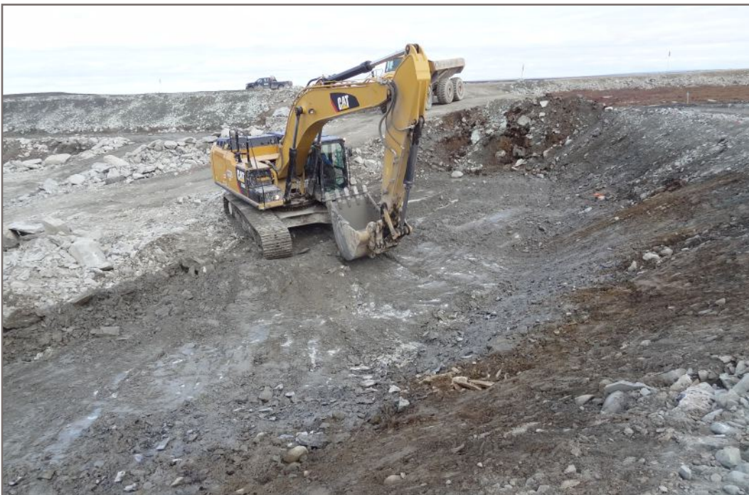
Photo 4: Excavating to competent bedrock (southeast corner)
