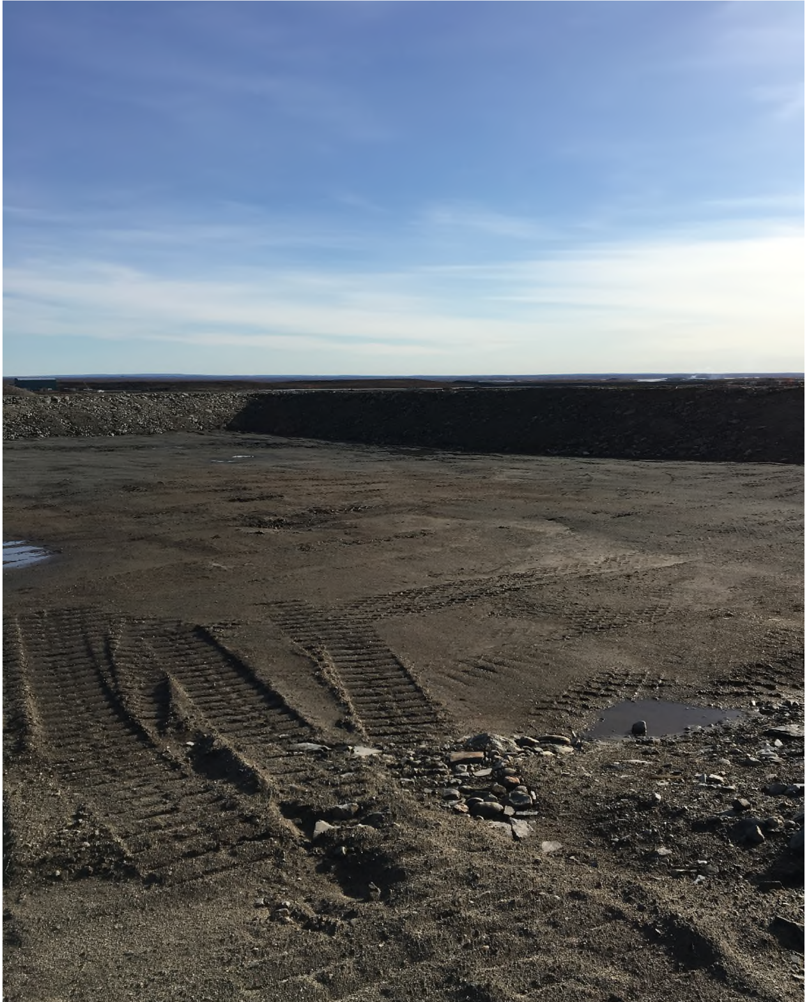
2017-08-28 Placement of second lift of Class A material on northwest berm
