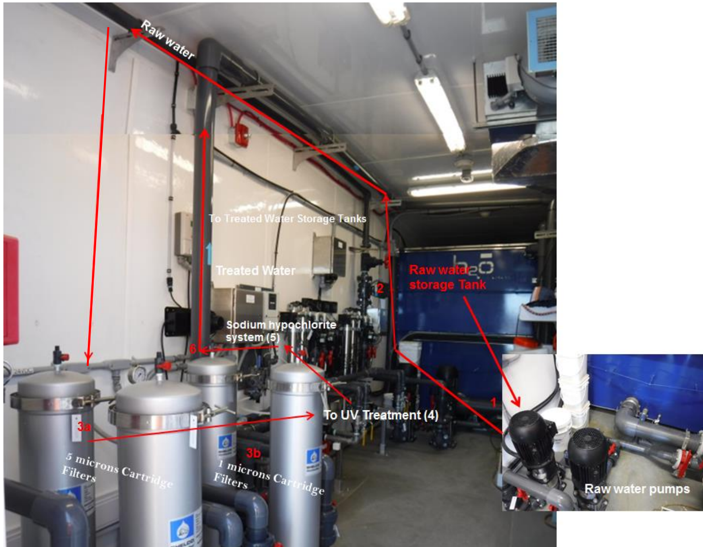
Photos of the Fresh water treatment system (Cartridge filters treatment and Chemical Treatment)
