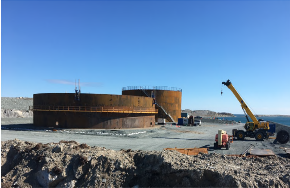
Picture 1: Construction of Rankin Inlet Itivia Site Fuel Storage and Containment Facilities (Tank #1 is in the foreground and Tank #2 is in the background)
