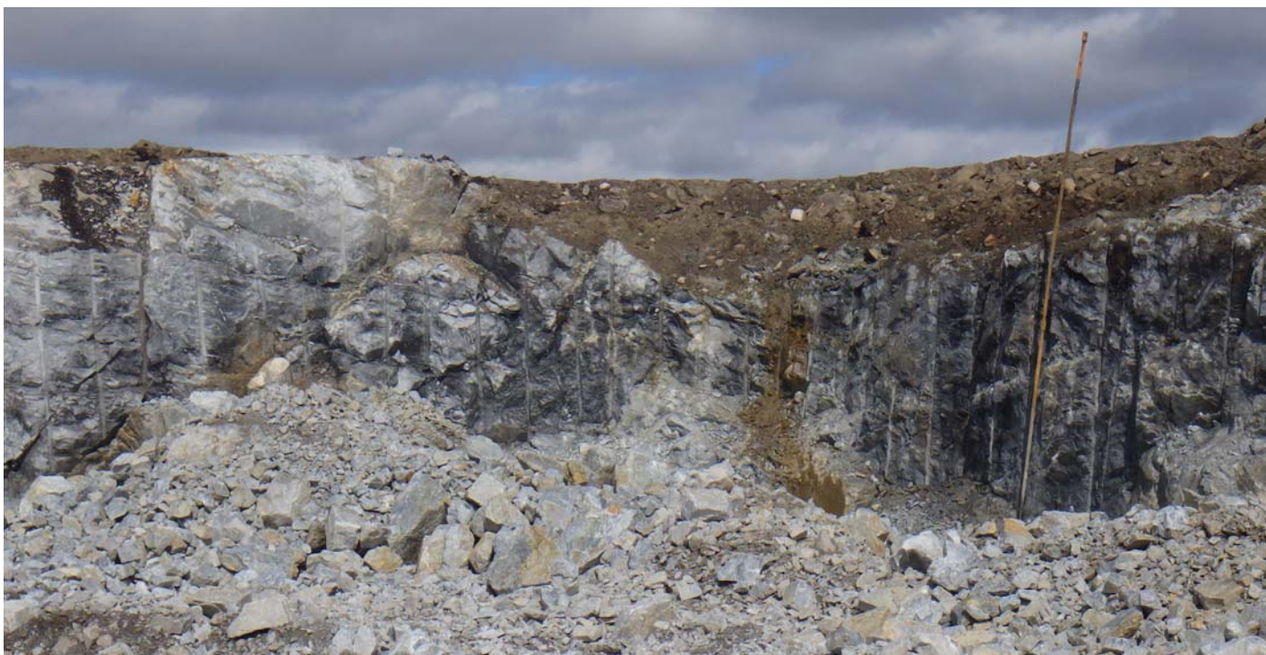
Figure 5 - Inspection area after scaling – corner area
