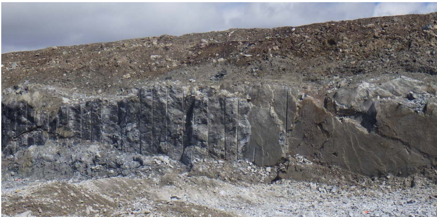
Figure 1 - Inspection area after scaling
