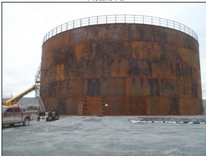
View of tank 2
