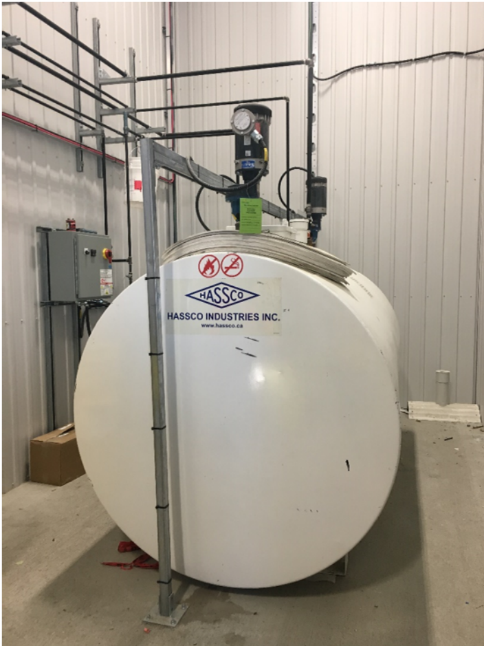
Photo 7 Incinerator's used oil tank
