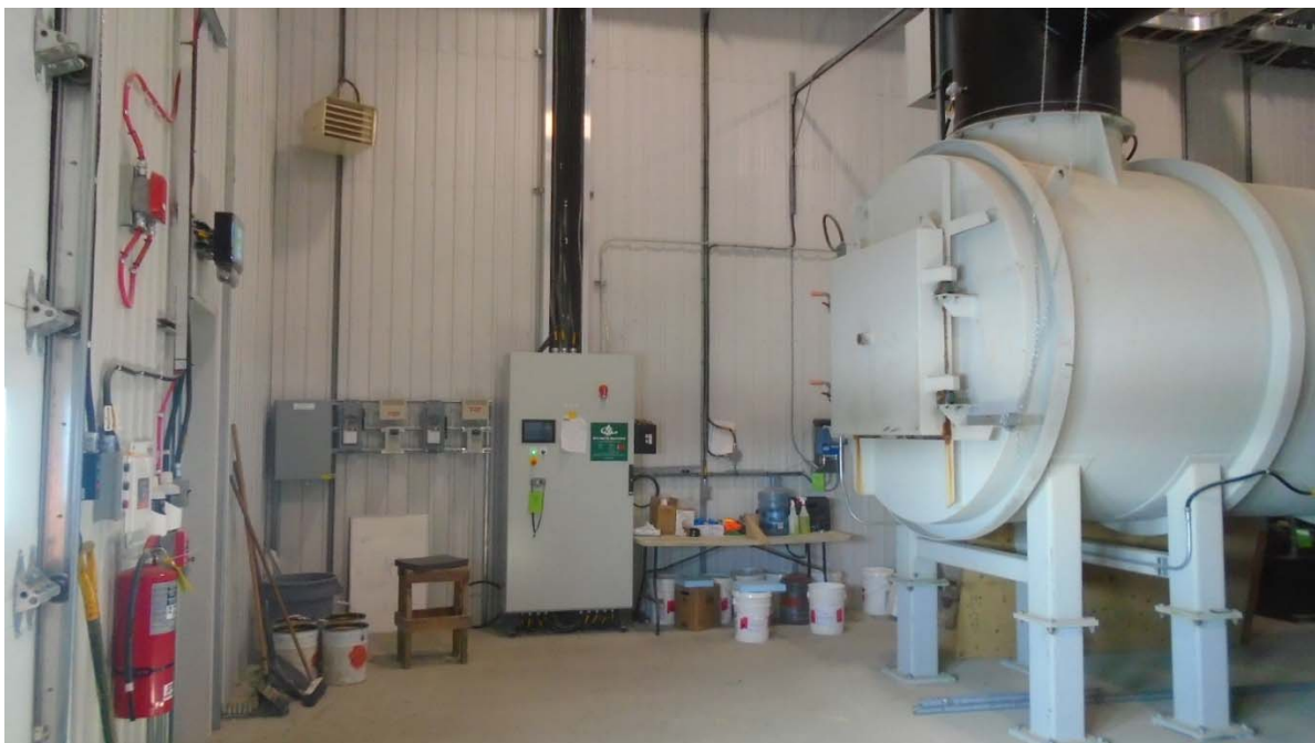
Photo 4 Incinerator's secondary chamber and control panel
