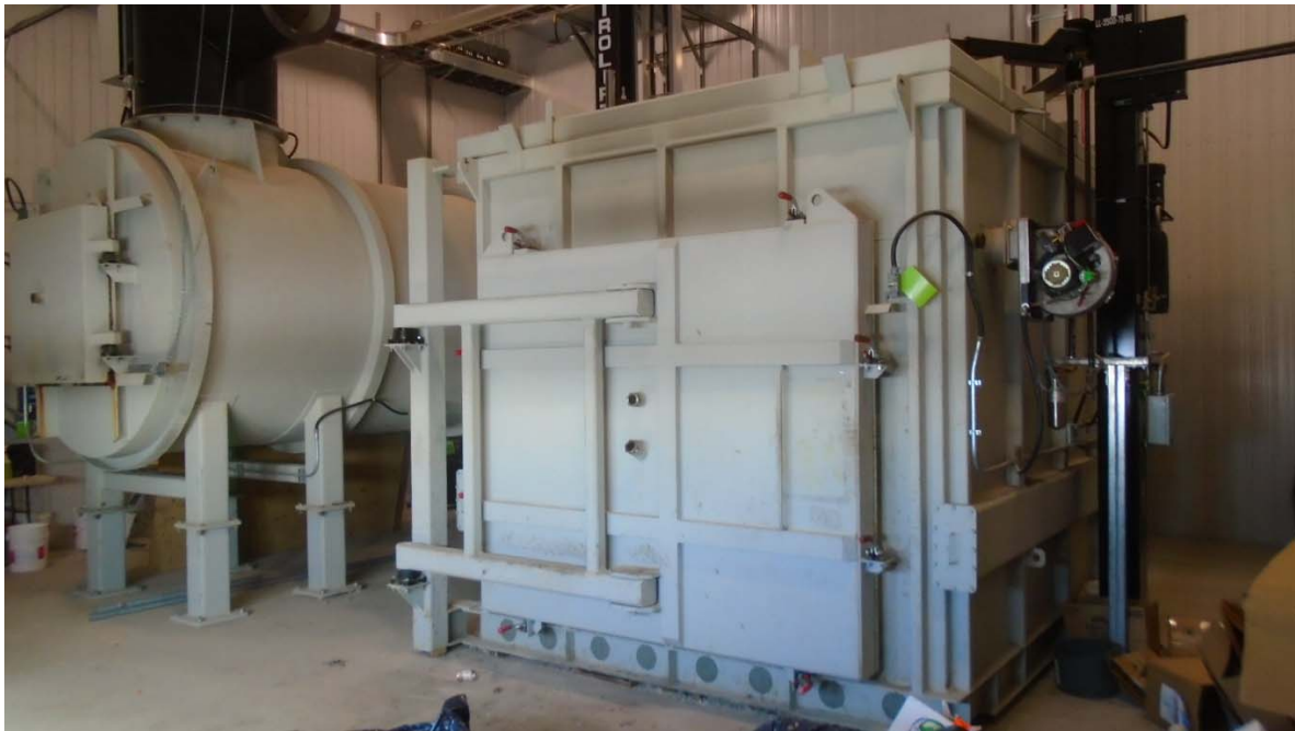
Photo 3 Incinerator's primary chamber (right) and secondary chamber (left)
