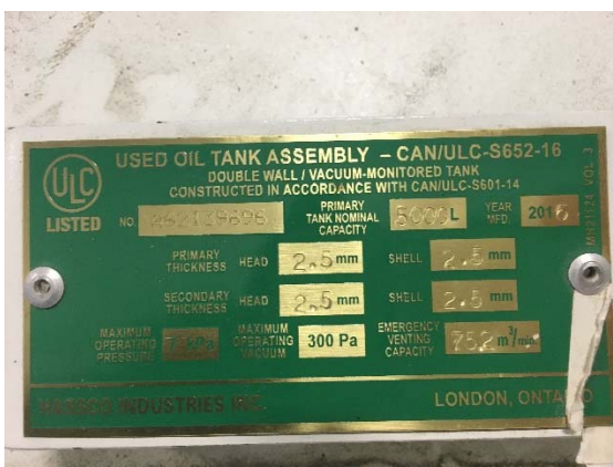
Photo 8 Incinerator's used oil tank plate
