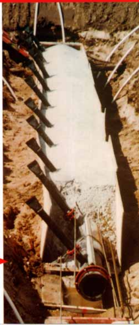
44 four-inch Tideflex diffuser valves installed on this award-winning diffuser system for a food processing plant discharging to the Des Moines River.
