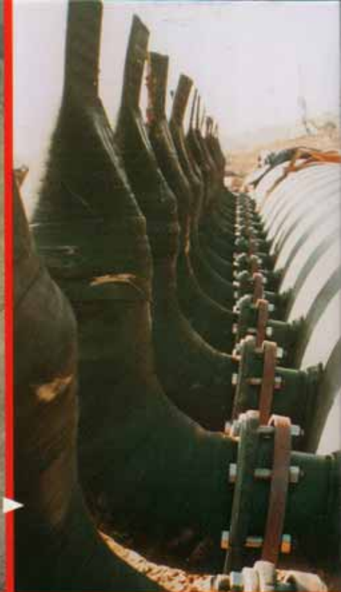
Eighteen 8" series 35D valves with integral 90° elbows for effluent diffuser in Georgia.
