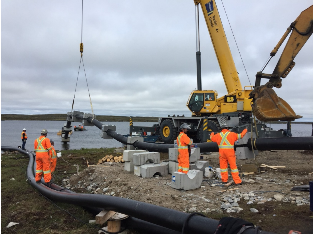
Photo 3 Installation of suction line and fresh water intake in Meliadine Lake
