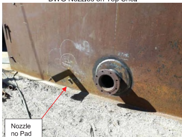
DWG Nozzles on Top Shell
