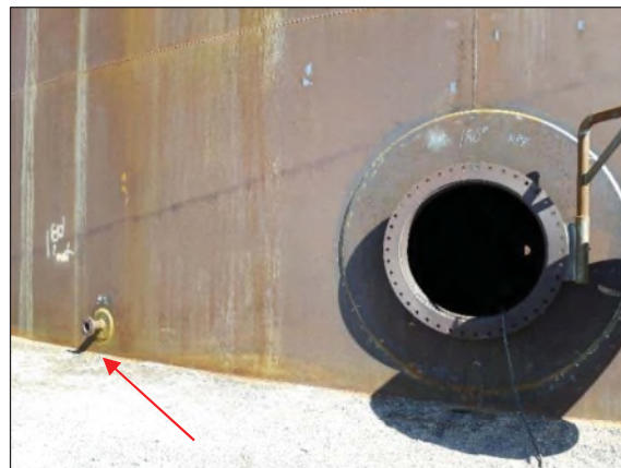
Nozzles 6 and 7 (Manhole 180°)
