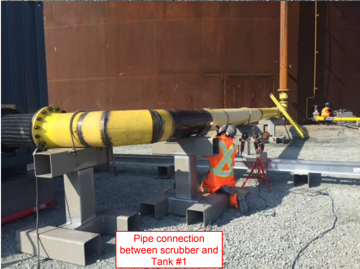
Pipe support installation
