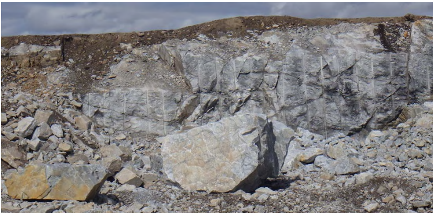
Figure 4 - Inspection area after scaling
