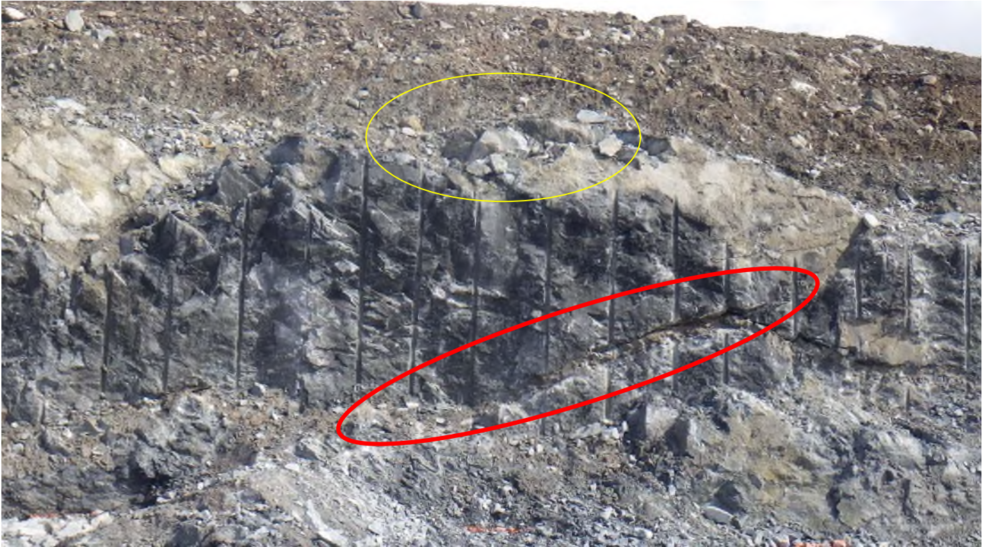
Figure 2 - Inspection area after scaling – showing fault
