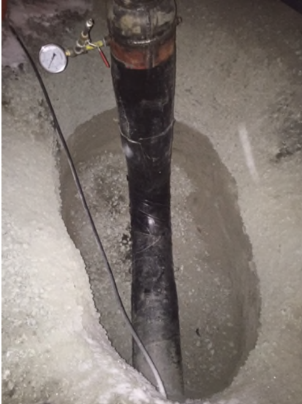
Photo 1b New double-wall elbow and vertical section on the East side of the road
