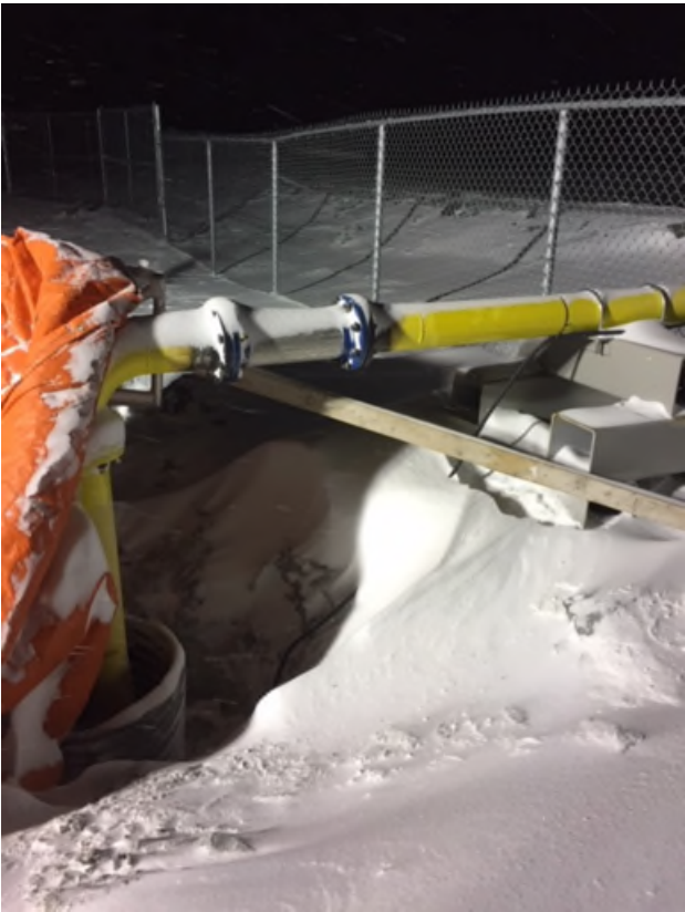
Photo 1c New double-wall elbow and vertical section on the East side of the road
