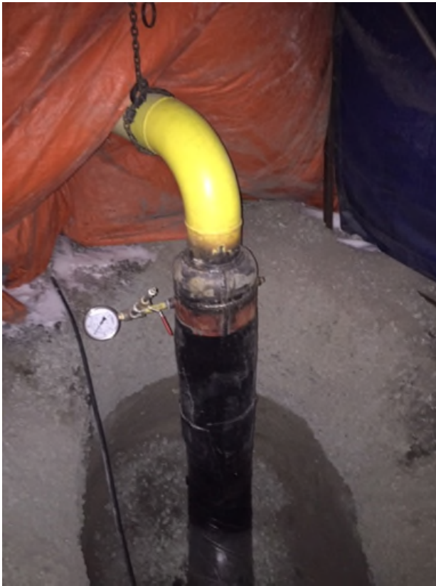
Photo 1a New double-wall elbow and vertical section on the East side of the road
