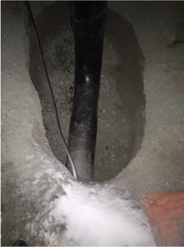
Photo 1c New double-wall elbow and vertical section on the East side of the road
