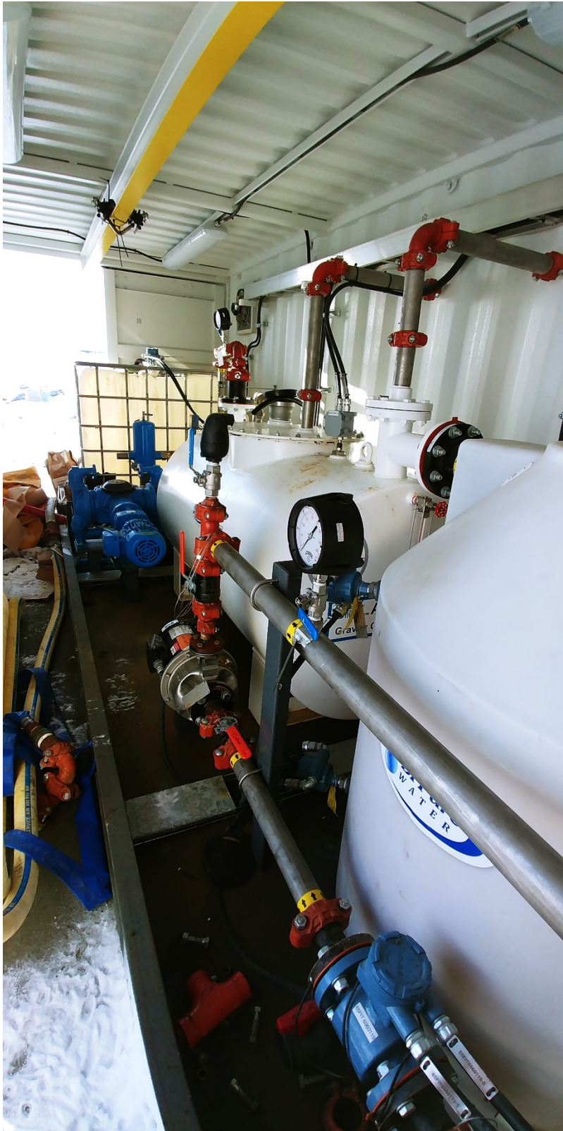
Photo 3 View inside the oil separator container (treated water tank and flow meter (forefront), oil separator (middle) and waste oil tote (back))
