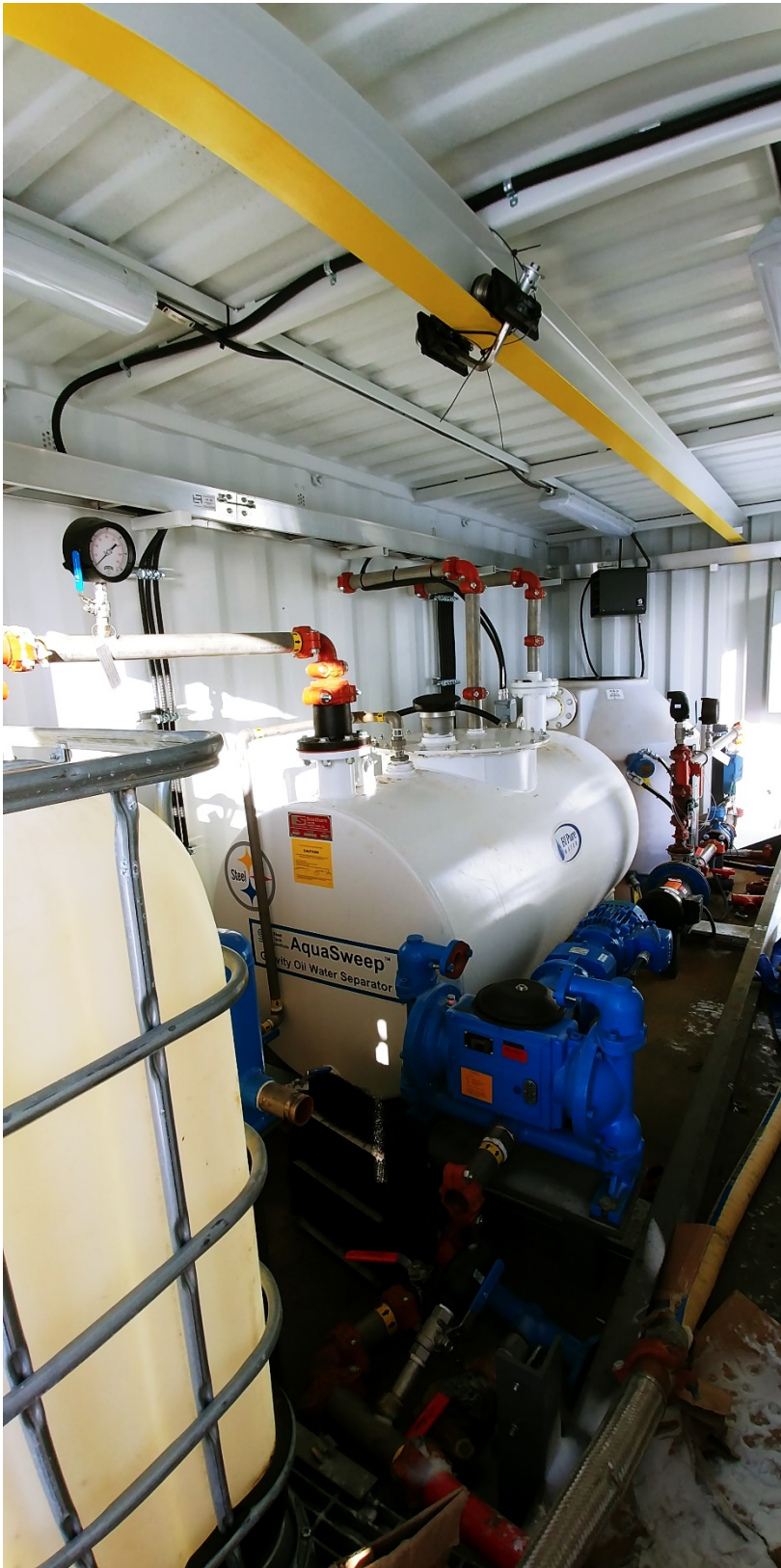
Photo 2 View inside the oil separator container (waste oil tote (forefront), oil separator (middle) and treated water tank (back))
