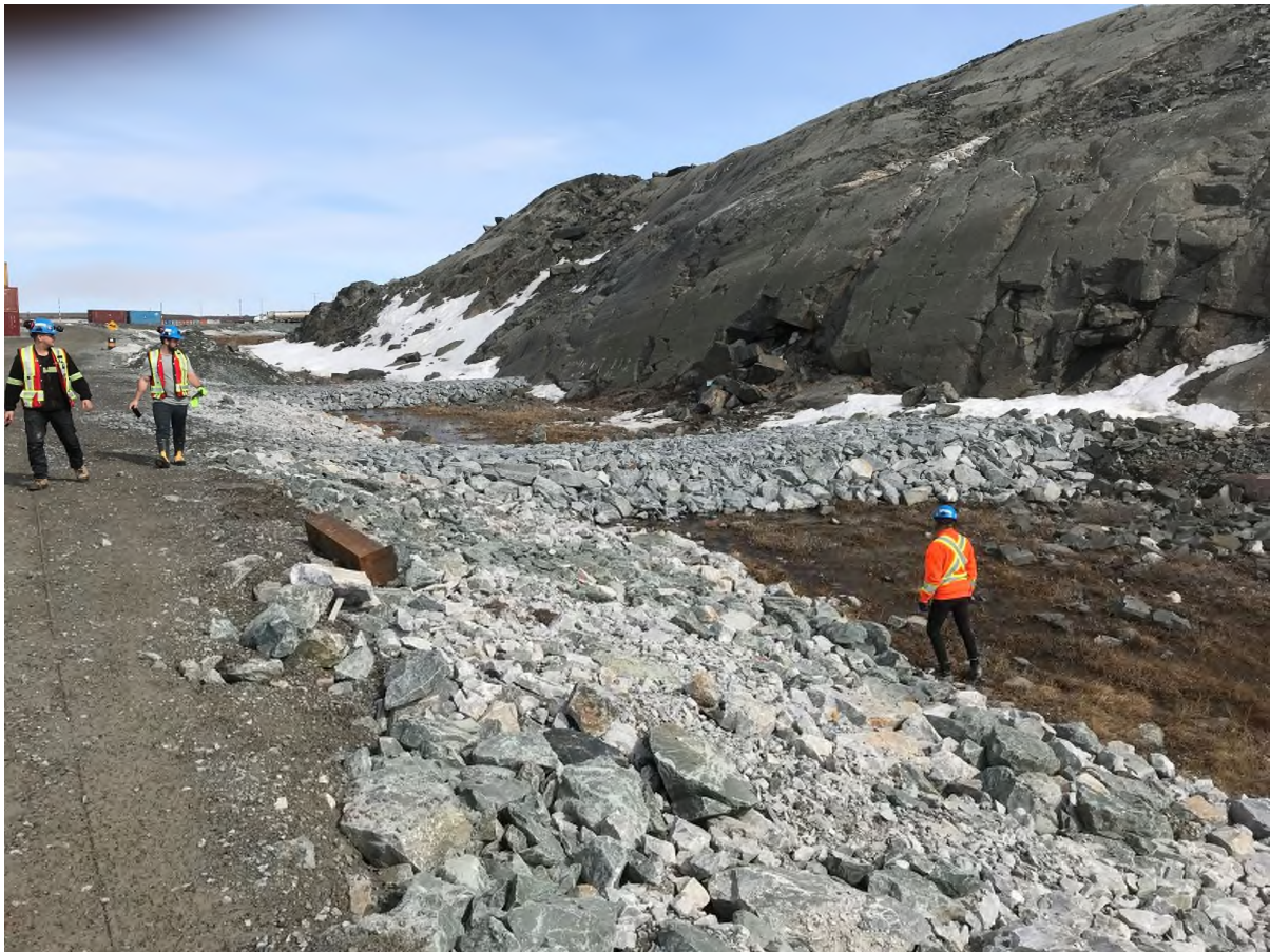
Photo taken looking upstream at the drainage culvert
