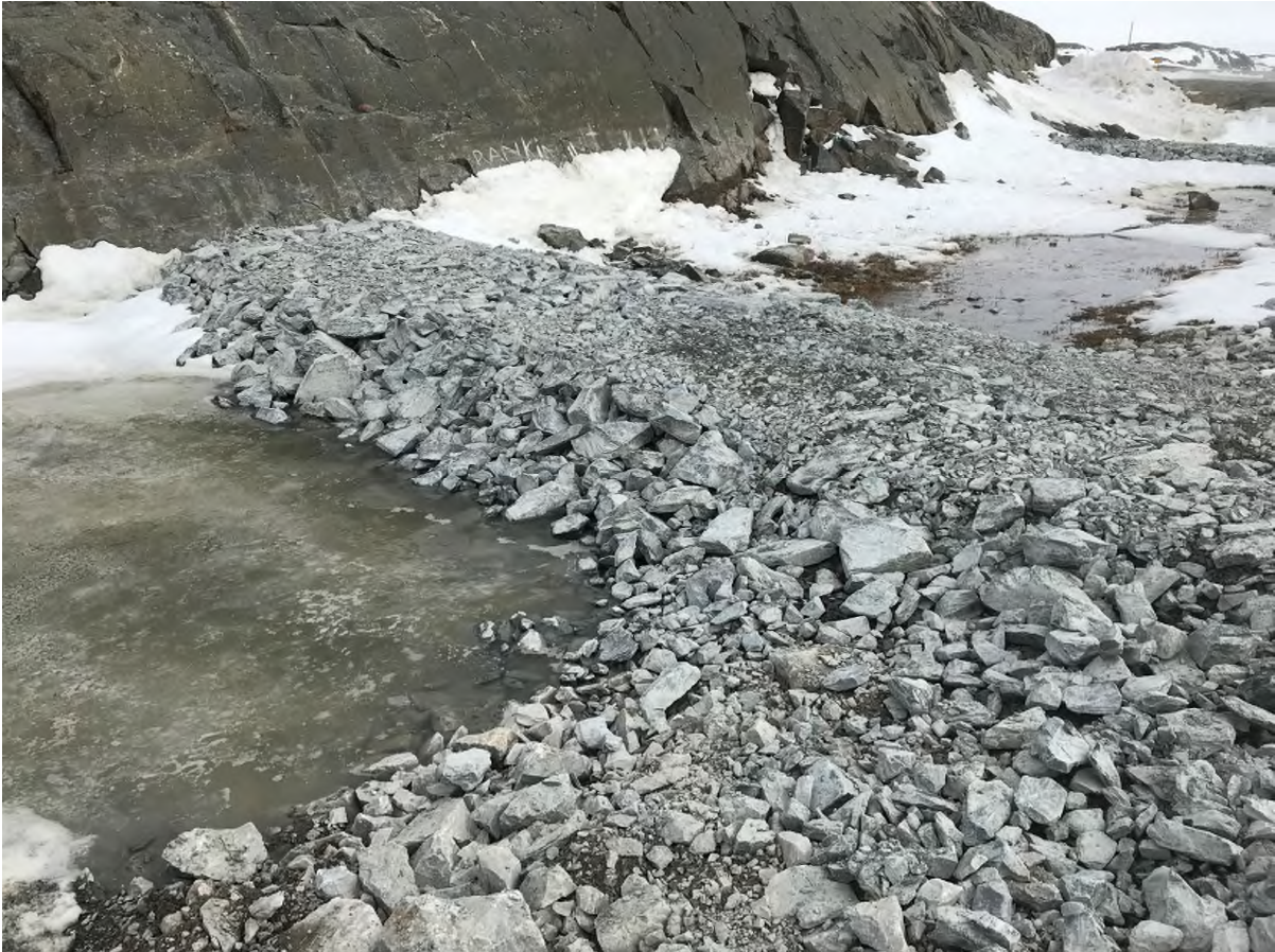
Photo taken of the upstream Rock Check Dam Retaining some Water
