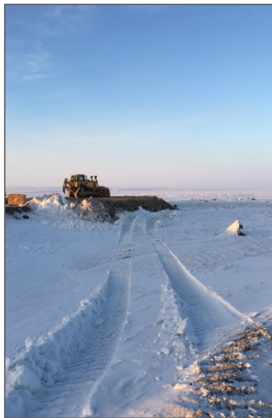
Photo 21: 11 25 2018 Berm CP3 - Pushing overburden lift; view facing northwest
