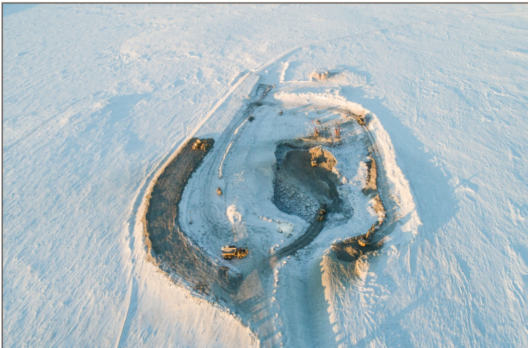
Photo 18: 12 08 2018 Pond CP3 - Excavation after Blast 5; drone view
