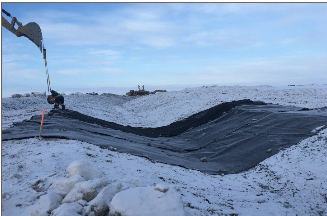
Photo 10: 11 30 2018 Channel3 - Geotextile placement; Station 1+580 facing up-chainage
