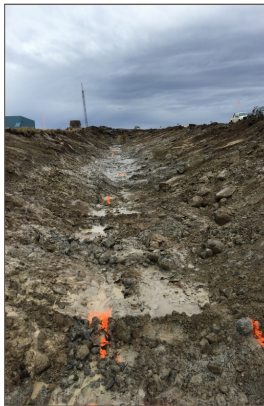
Photo 5: 08 29 2018 Channel3 - Mechanical excavation; Station 0+090 facing down-chainage
