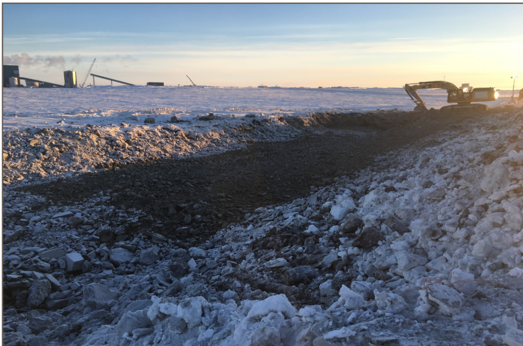
Photo 9: 11 26 2018 Channel3 - Overburden removal from Blast 1; Station 1+600 facing down-chainage
