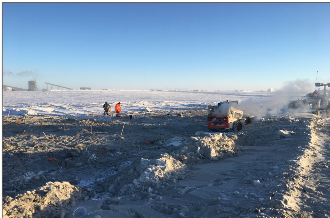
Photo 8: 11 24 2018 Channel3 - Loading holes Blast 1; Station 1+590 facing down-chainage
