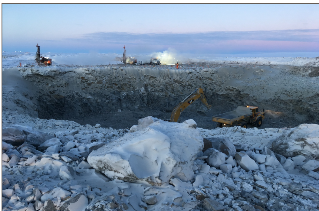
Photo 15: 12 06 2018 Pond CP3 - Excavation after Blast 4; view facing northeast
