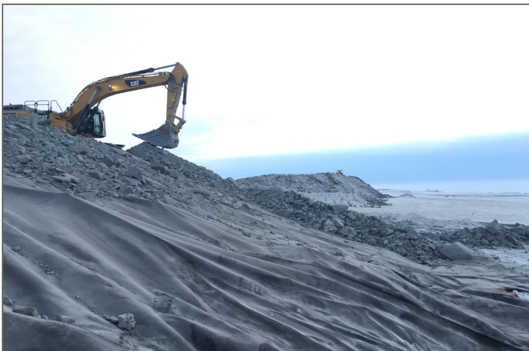
Photo 24: 12 18 2018 Berm CP3 - Geotextile and placement of downstream rock protection; view facing south
