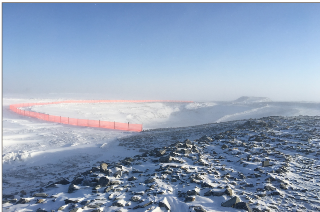
Photo 20: 02 16 2019 Pond CP3 - Completed snow fence; view facing southeast
