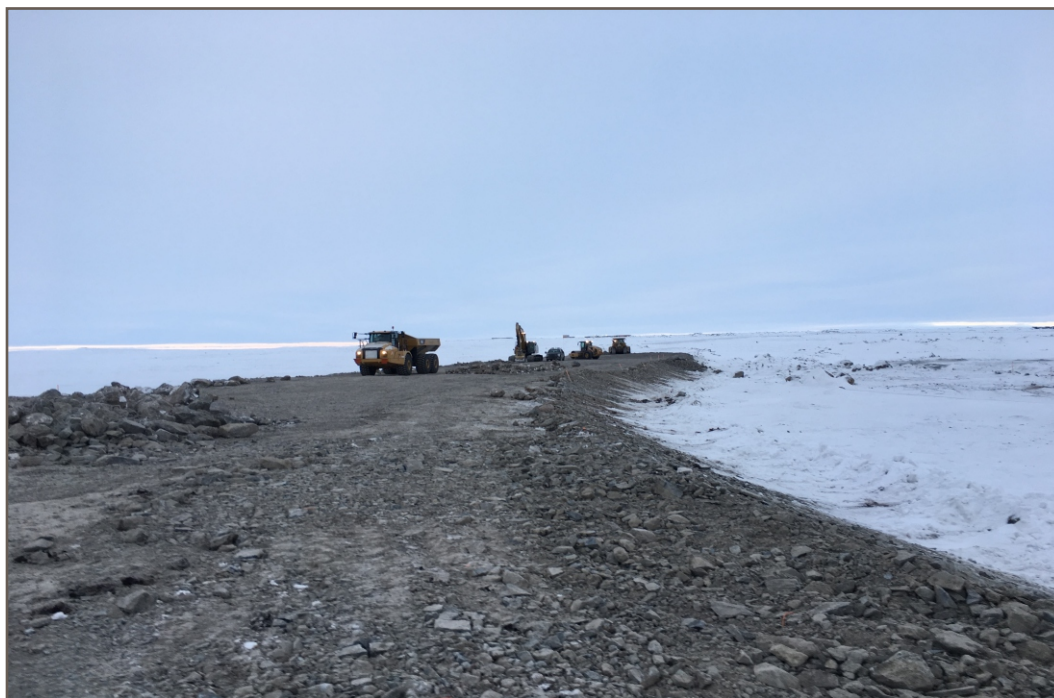
Photo 22: 11 27 2018 Berm CP3 - Placement of overburden Lift 2; view facing north
