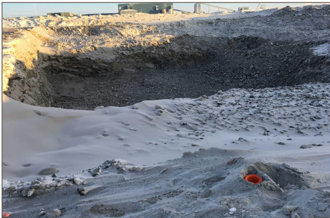
Photo 16: 12 07 2018 Pond CP3 - Excavation after Blast 4; view facing east
