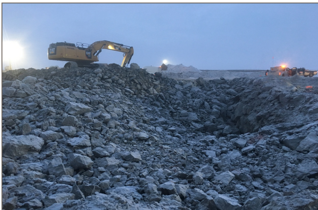
Photo 13: 11 29 2018 Pond CP3 - Excavation after Blast 3
