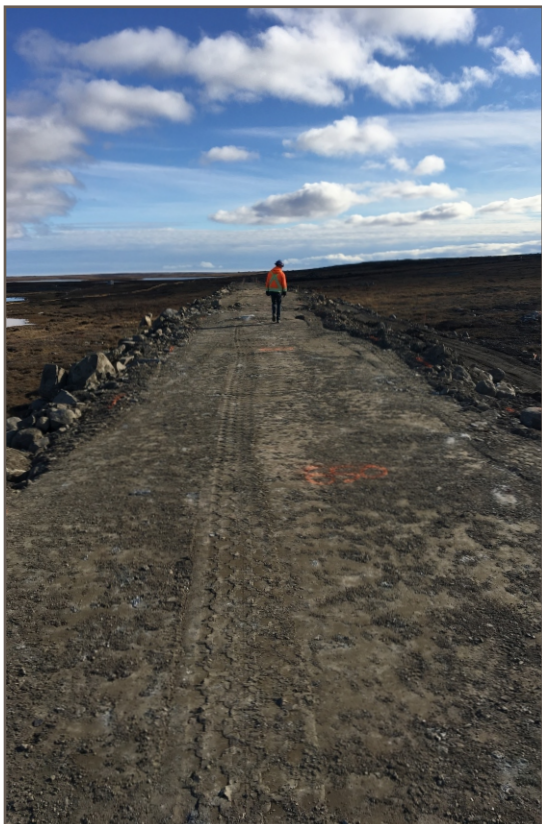
Photo 2: 09 13 2018 Berm2 - Compacted esker material; view from Station 0+240 facing down-chainage
