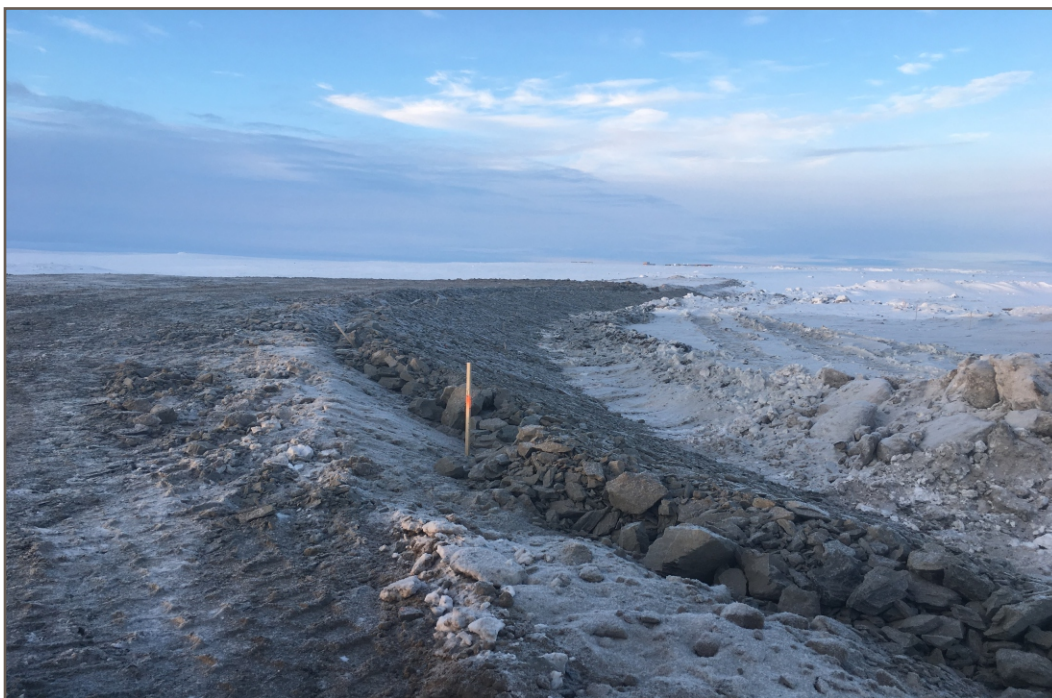
Photo 23: 11 29 2018 Berm CP3 - Placement of upstream rock protection; view facing north
