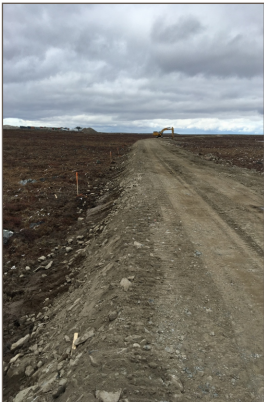
Photo 4: 09 16 2018 Berm2 - Sloping downstream; view from Station 0+400 facing up-chainage
