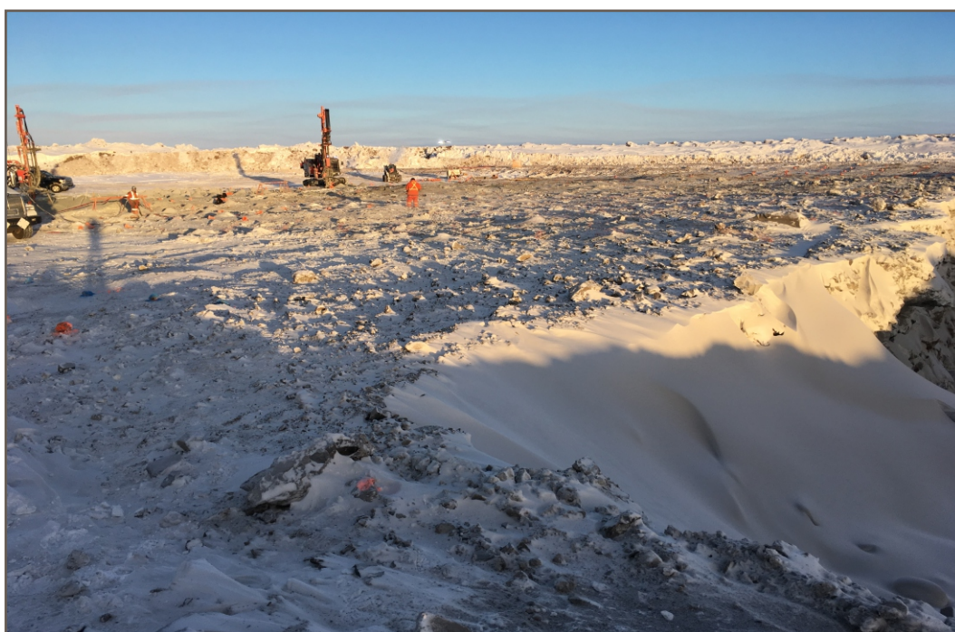
Photo 17: 12 07 2018 Pond CP3 - Loading emulsion for Blast 5; view facing northeast
