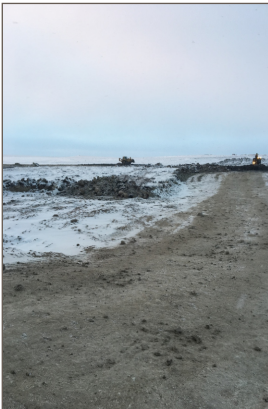
Photo 12: 10 23 2018 Pond CP3 - Mechanical overburden excavation; view facing north
