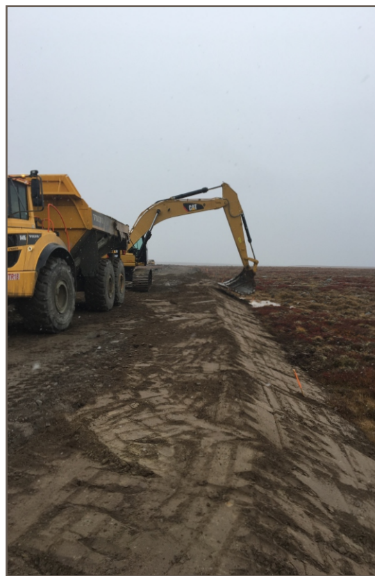
Photo 1: 09 11 2018 Berm2 - Sloping of upstream till; view from Station 0+520 facing down-chainage
