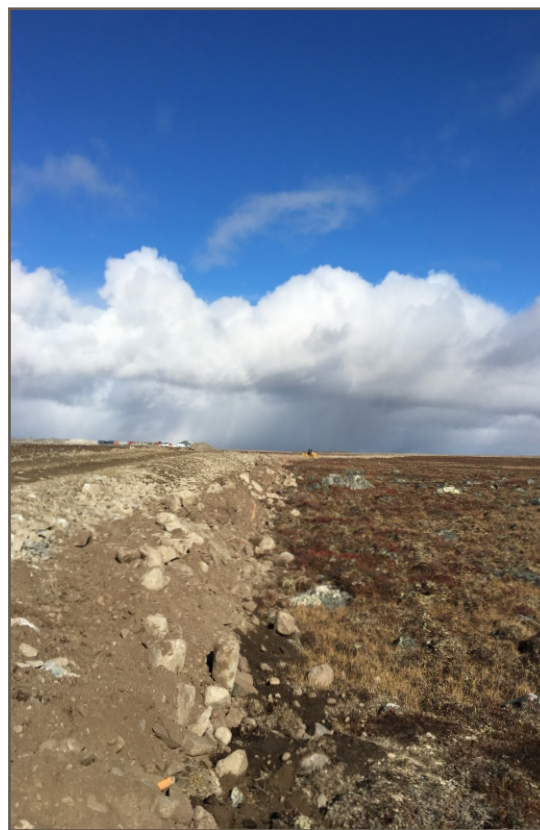
Photo 3: 09 15 2018 Berm2 - Unfinished downstream slope; view from Station 0+120 facing up-chainage
