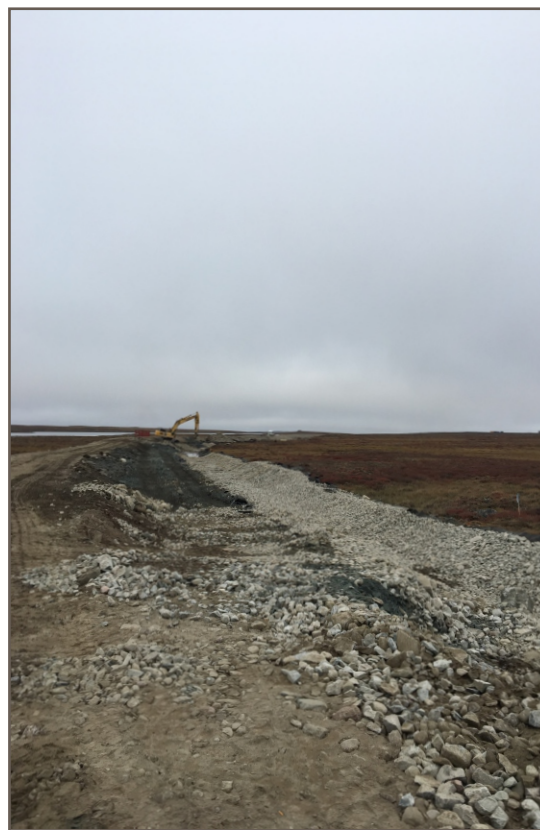
Photo 7: 09 03 2018 Channel3 - Rebuilt bank and channel construction; Station 1+185 facing up-chainage
