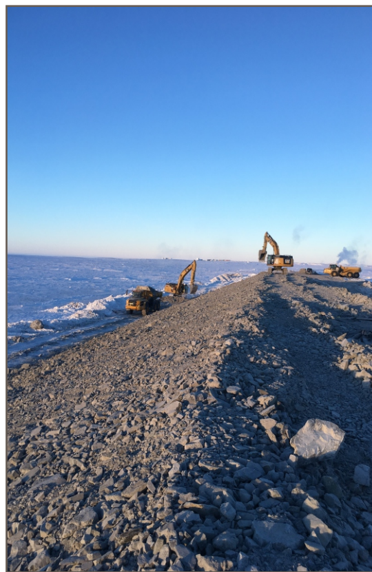
Photo 25: 12 19 2018 Berm CP3 - Final upstream slope; view facing north
