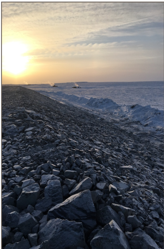
Photo 26: 01 22 2019 Berm CP3 - Completed downstream slope; view facing south
