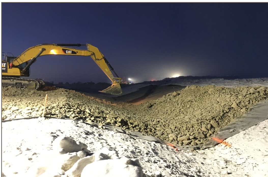
Photo 11: 11 30 2018 Channel3 - Rip rap placement; Station 1+580 facing up-chainage
