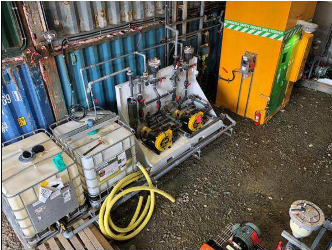
Hypochlorite dosing skid and emergency shower
