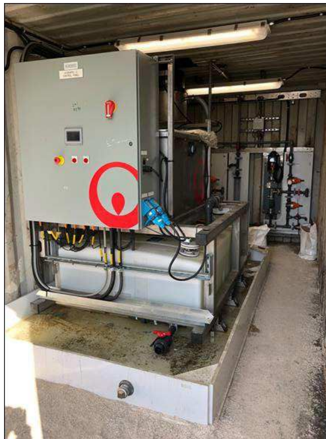
Polymer make down and dosing skid
