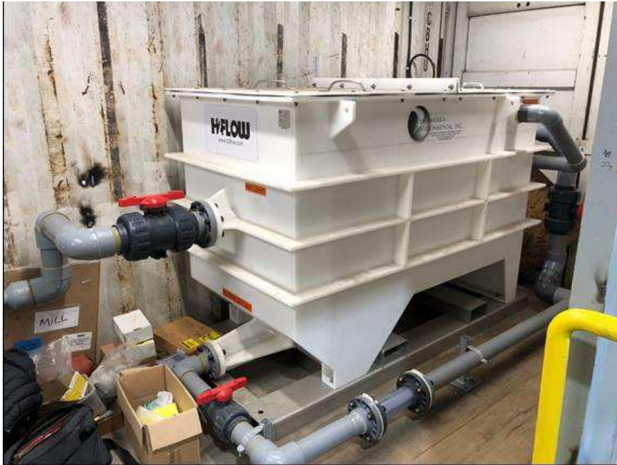
Oils and grease separator
