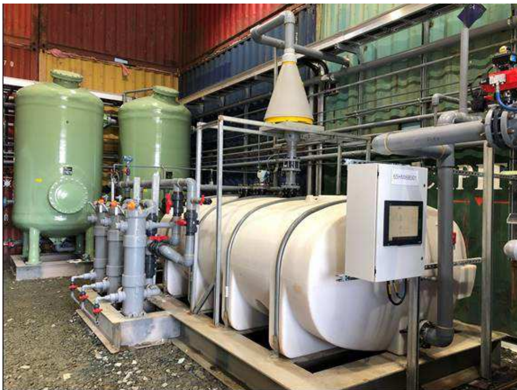
Chlorination reactor and pre-filter skids
