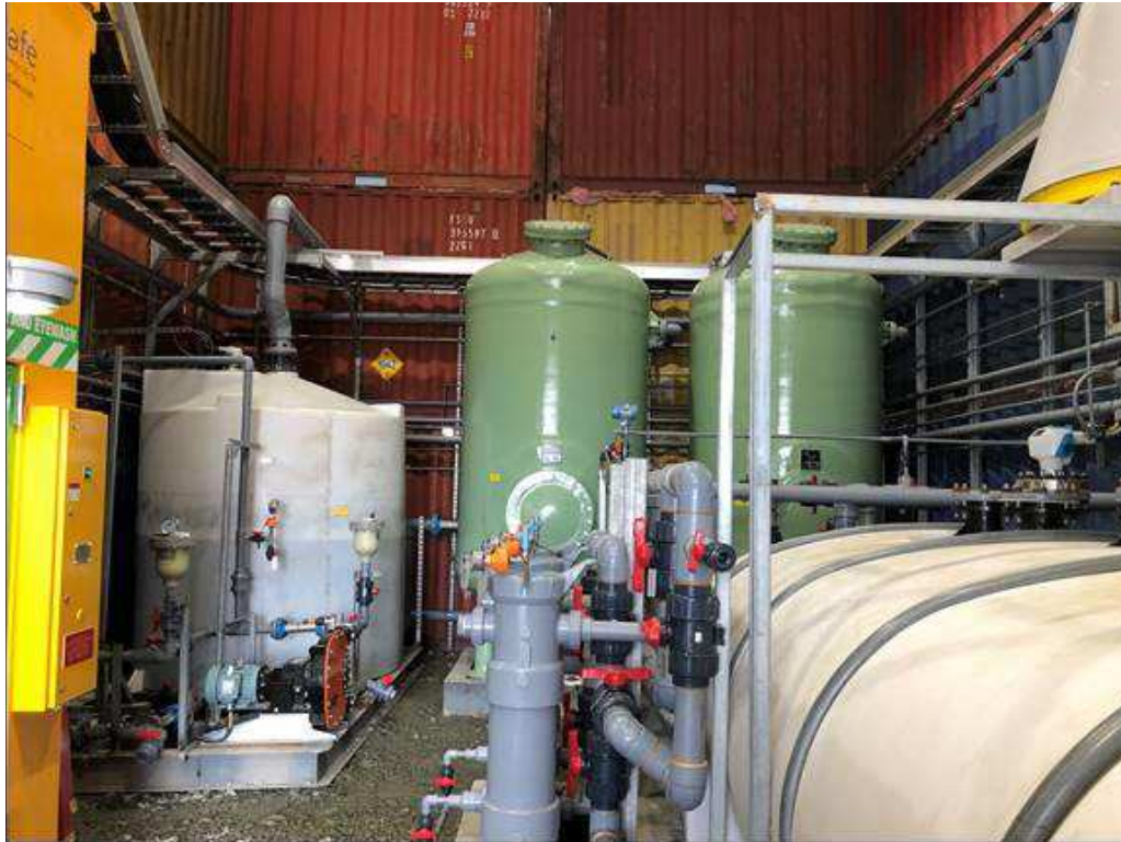
Activated carbon filter and backwash tank
