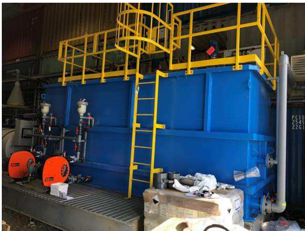
Multiflo clarifier and sludge recirculation pumps
