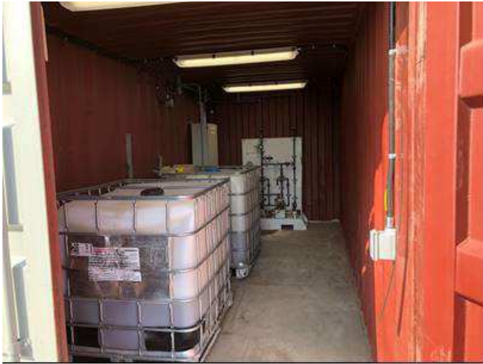
Coagulant dosing Skid
