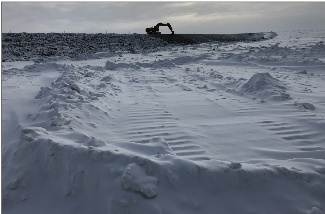
Photo 27: 2019-02-15 Berm CP4 - Sloping overburden Berm CP4
