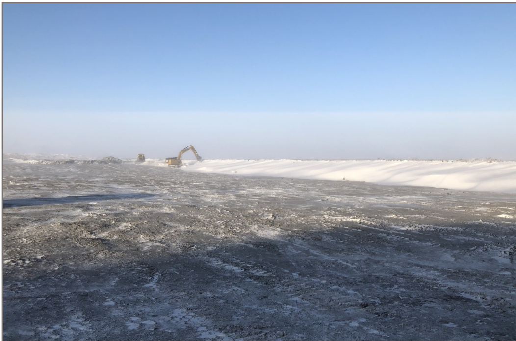
Photo 28: 2019-03-25 Berm CP4 - Snow removal prior to Berm CP4 construction with Pond CP4 overburden
