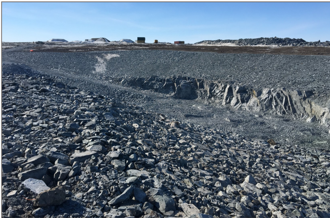
Photo 19: 2019-05-04 Pond CP4 - Completed Pond CP4
