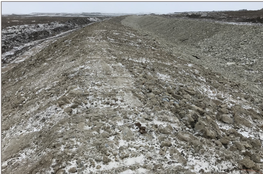
Photo 8: 2019-05-12 Channel4 - Completed Channel4 berm Station 0+460
