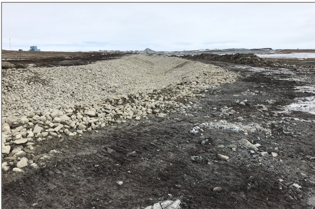
Photo 4: 2019-05-09 Channel4 - Completed Channel4 Station 0+160 up chainage
