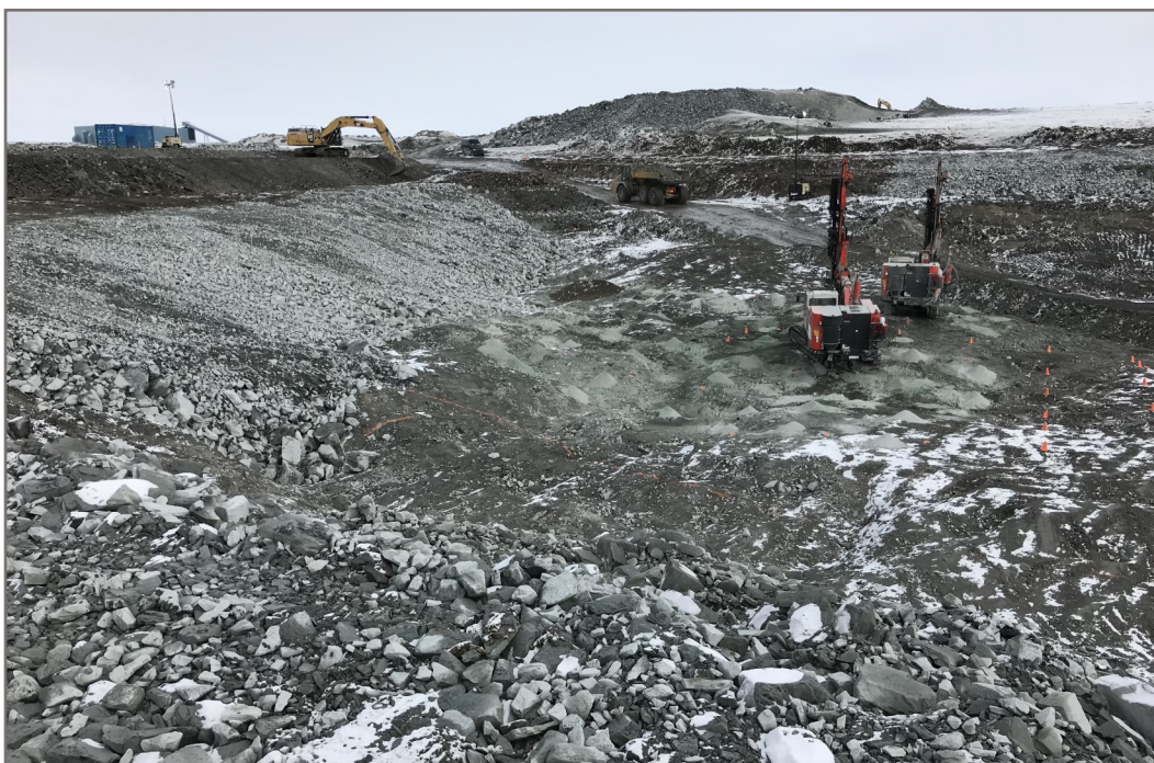
Photo 16: 2019-04-13 Pond CP4 - Drilling first rock blast and placing overburden protection
