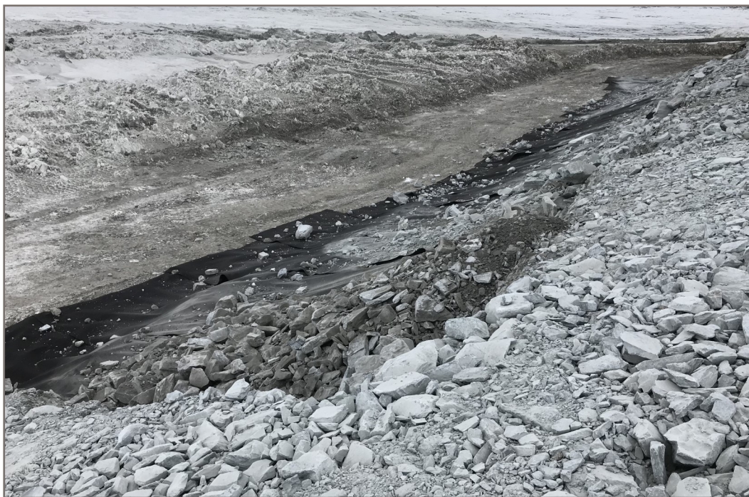
Photo 29: 2019-04-11 Berm CP4 - Rock placement over geotextile Berm CP4
