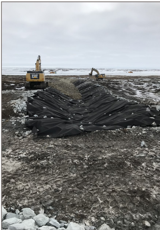
Photo 5: 2019-05-09 Channel4 - Riprap placement Station 0+020
