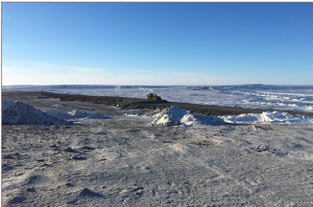
Photo 26: 2019-02-07 Berm CP4 - Pushing Berm CP4 with SP2 overburden
