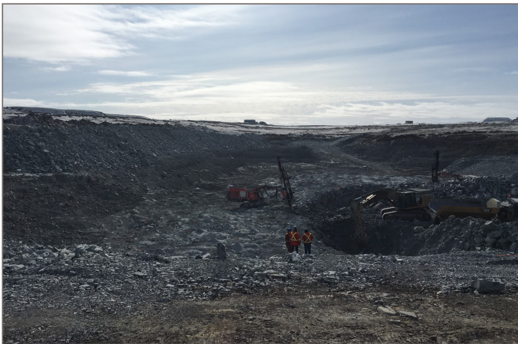
Photo 17: 2019-04-16 Pond CP4 - Mucking first rock blast (No.5) Pond CP4
