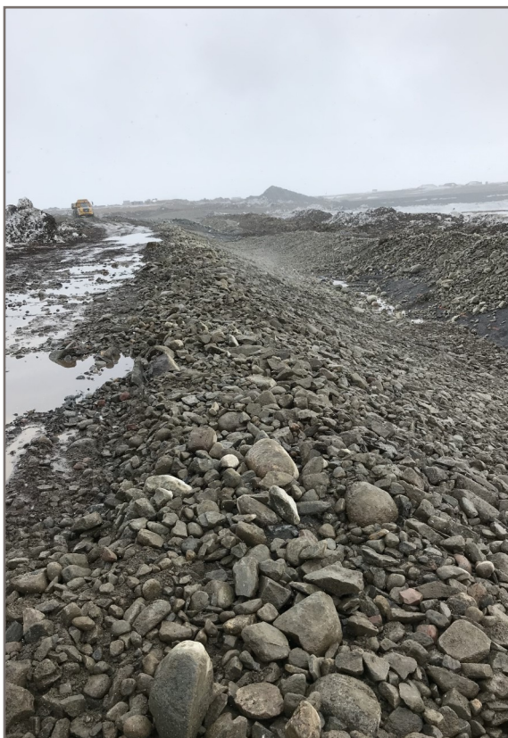
Photo 3: 2019-05-08 Channel4 - Riprap placement Station 0+700
