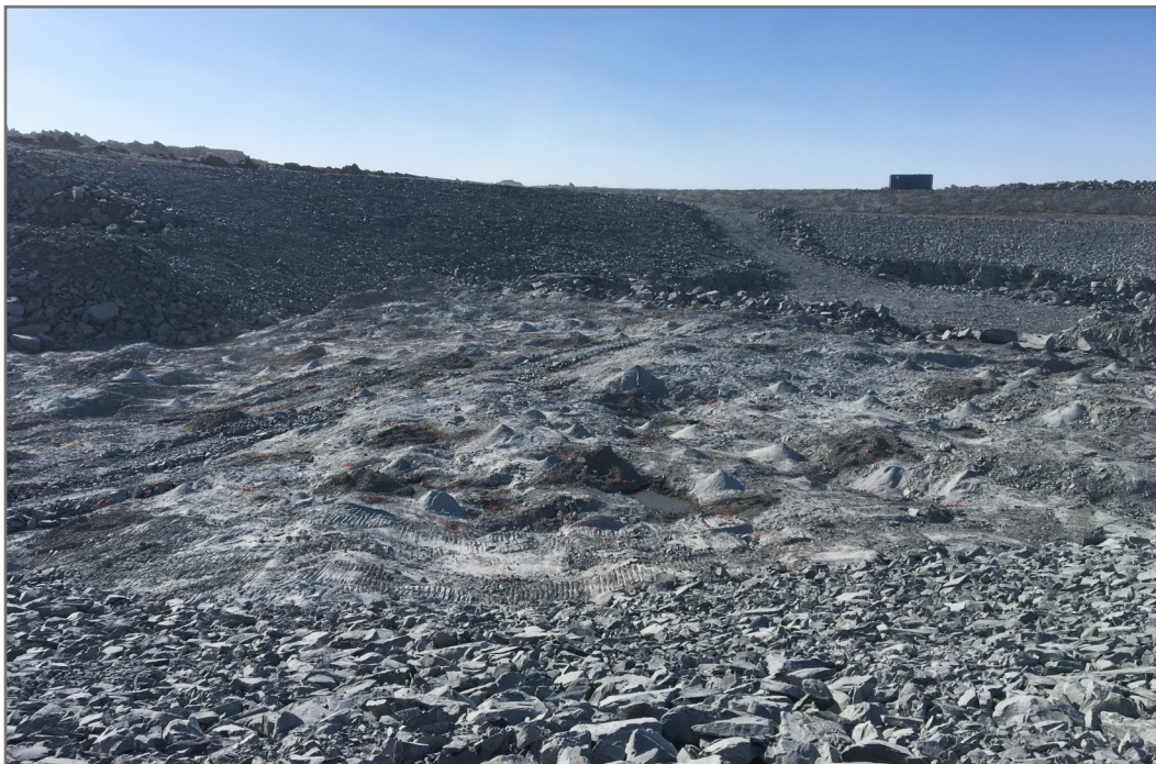
Photo 18: 2019-04-20 Pond CP4 - Overburden protection and bedrock surface before blasting
