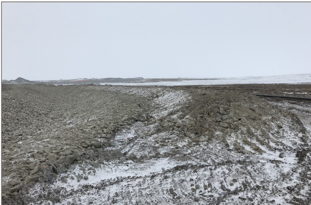
Photo 7: 2019-05-12 Channel4 - Completed Channel4 berm Station 0+180 up chainage
