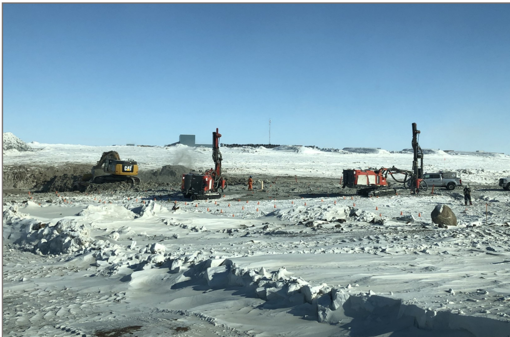
Photo 12: 2019-03-21 Pond CP4 - Drill blast operations Pond CP4
