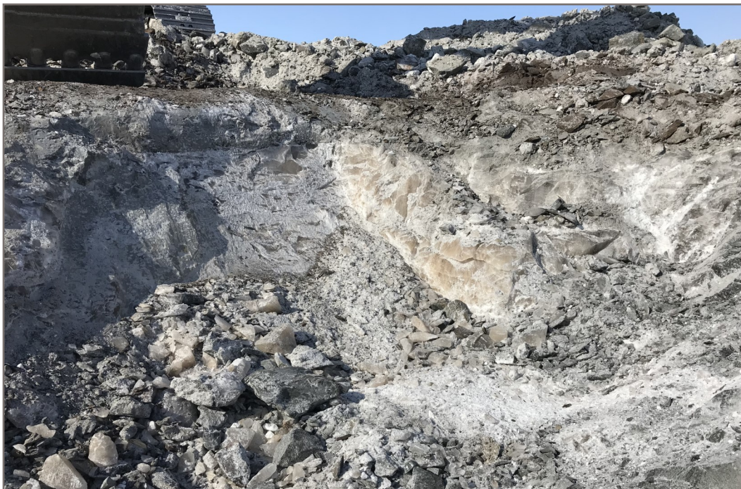
Photo 14: 2019-04-03 Pond CP4 - Excavating ice wedge from Pond CP4 wall
