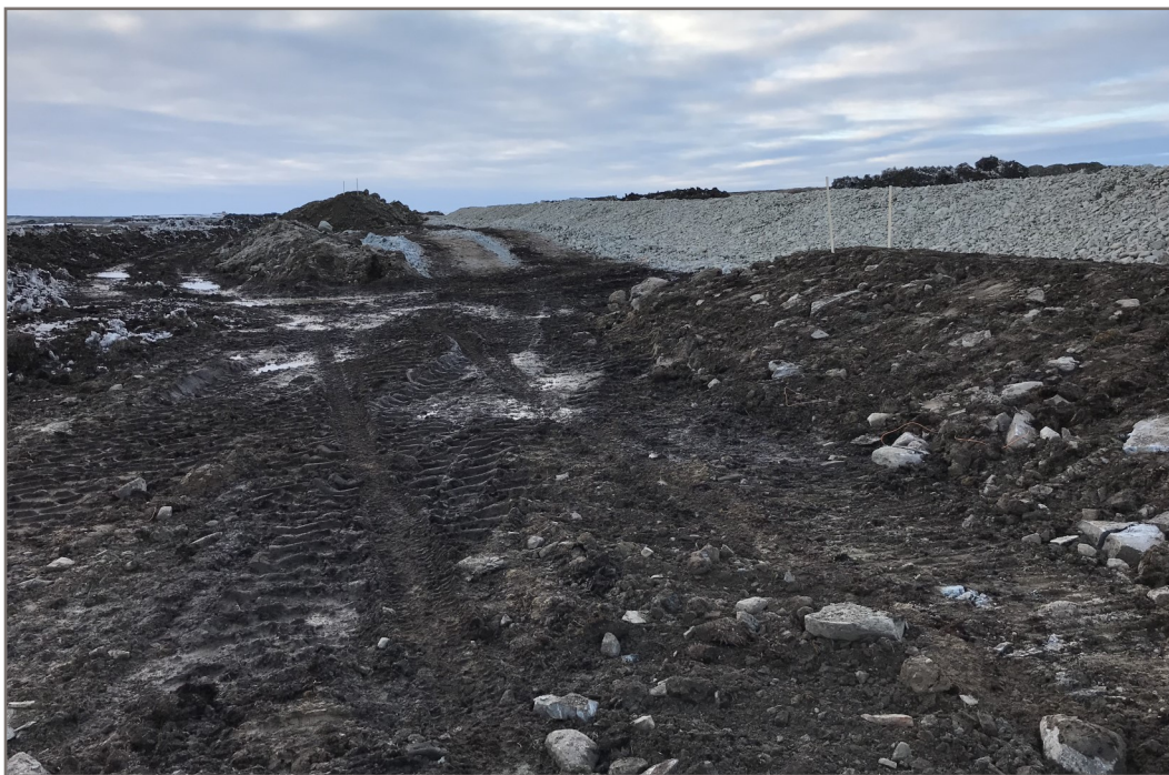
Photo 6: 2019-05-11 Channel4 - Shaping Channel4 berm
