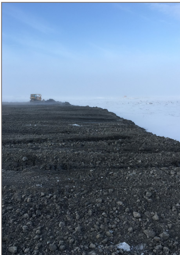
Photo 25: 2018-11-03 Berm CP4 - Pushing lift #1 of Berm CP3
