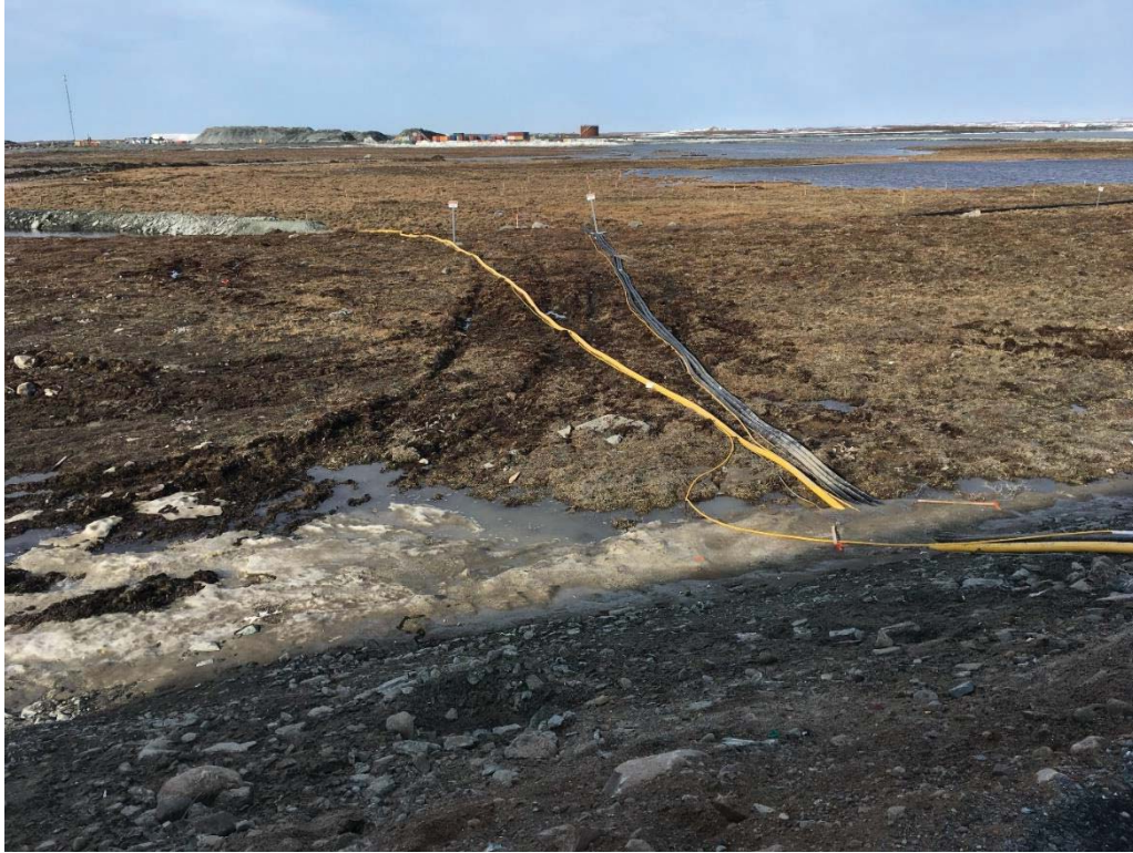
Photograph 1: Electrical cables across OP2 footprint to protect prior to ROM placement, these cables were identified with tires being place on top of the pad after ROM placement; view facing northwest (June 10, 2018)
