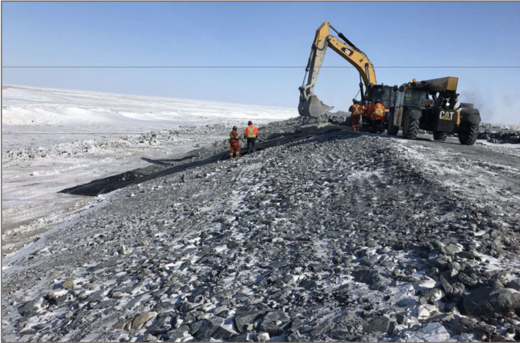
Photo 9: 2020-03-30 Berm CP6 - Placing geotextile on upstream slope on Berm CP6; view facing northeast
