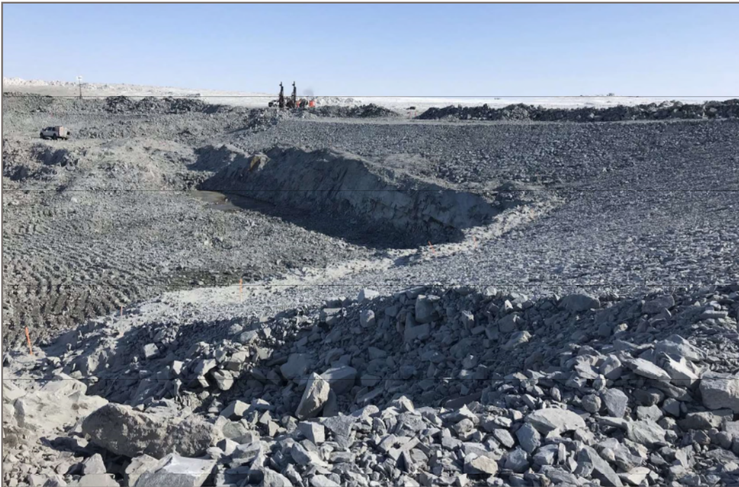
Photo 10: 2020-03-30 Berm CP6 - Placement of thermal protection on Berm CP6; view facing northeast
