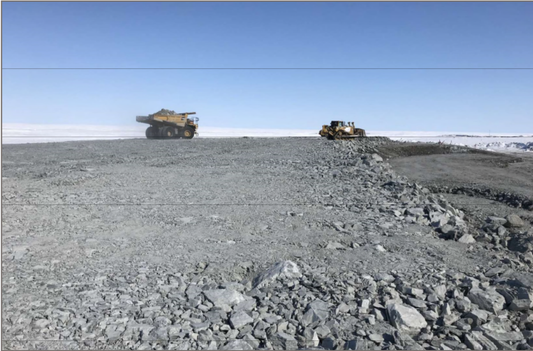
Photo 15: 2020-04-05 Berm CP6 - Placement of final erosion cover on Berm CP6; view facing northeast.
