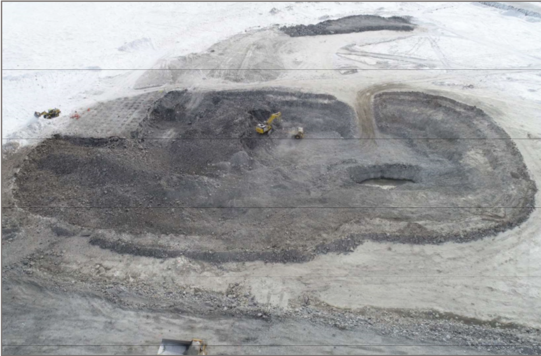
Photo 7: 2020-03-22 - Drone view of Pond CP6 and Berm CP6
