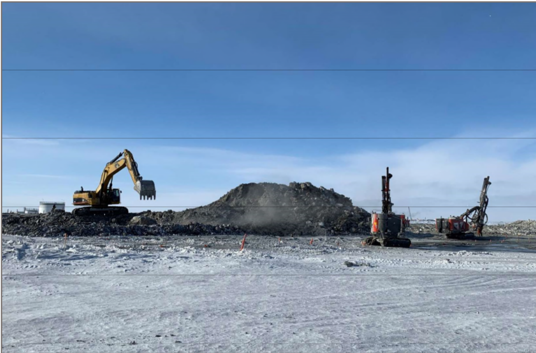
Photo 2: 2020-03-10 Pond CP6 - Mucking first blast; view facing north
