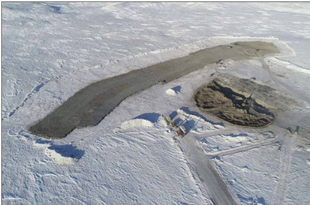
Photo 4: 2020-03-13 - Drone view of Pond CP6 and Berm CP6
