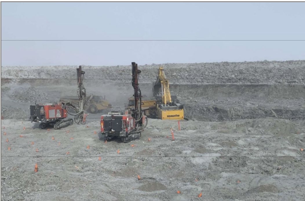
Photo 12: 2020-04-01 Berm CP6 - Drilling and mucking rock bench on Berm CP6; view facing north
