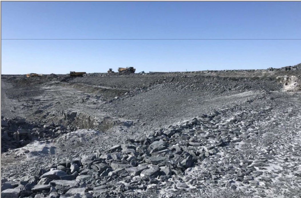
Photo 14: 2020-04-04 Berm CP6 - Placement of thermal protection on Berm CP6; view facing southwest
