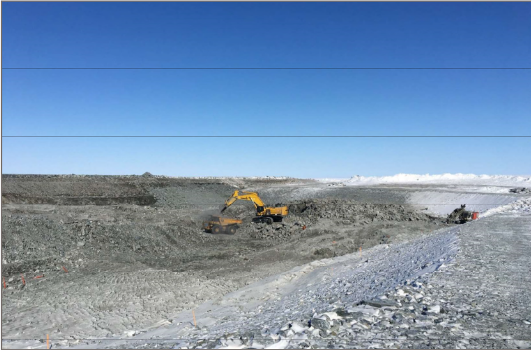
Photo 13: 2020-04-04 Pond CP6 - Mucking blast rock from Pond CP6; view facing northeast
