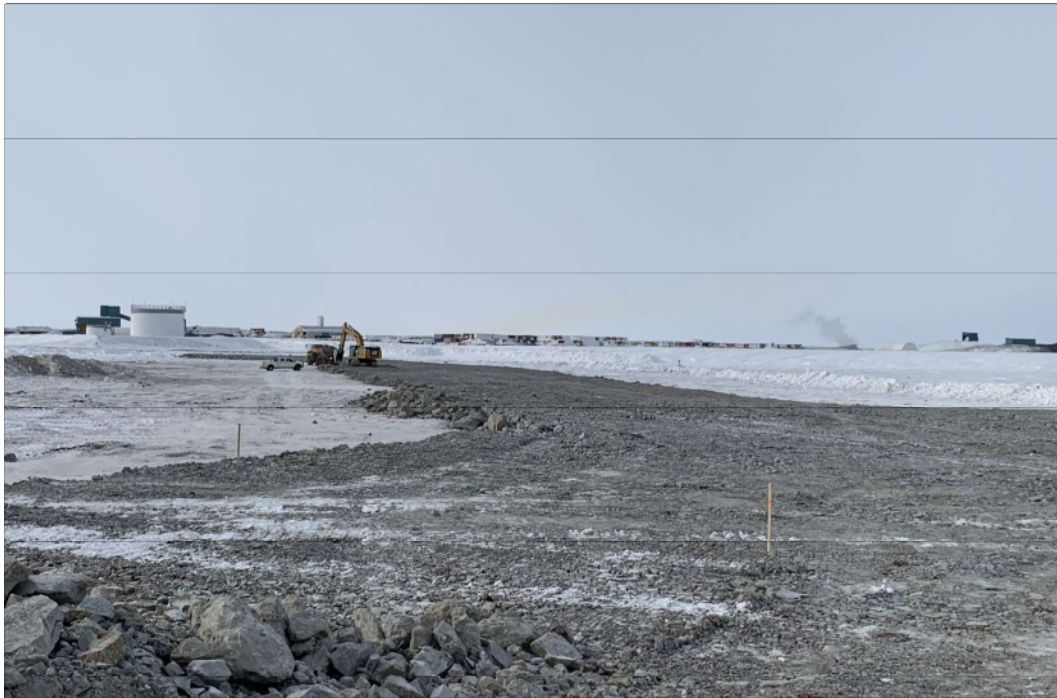
Photo 3: 2020-03-12 Berm CP6 - First lift overburden on Berm CP6; view facing southwest
