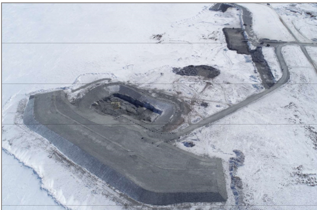
Photo 17: 2020-04-11 - Drone view of Pond CP6 and Berm CP6
