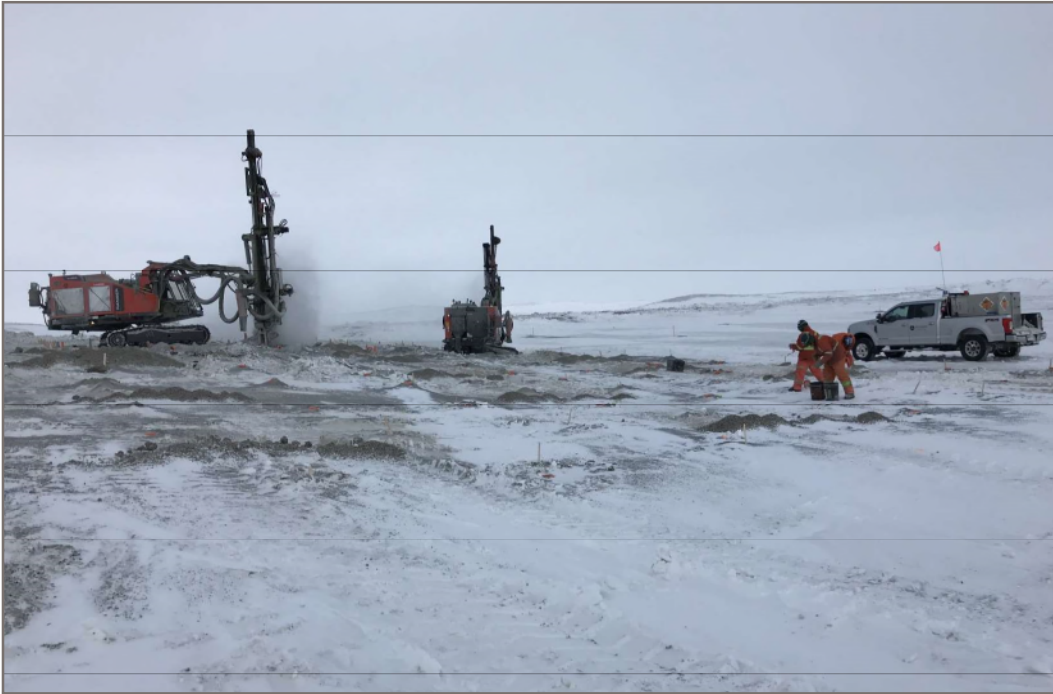
Photo 1: 2020-03-05 Pond CP6—Drilling first blast pattern; view facing east
