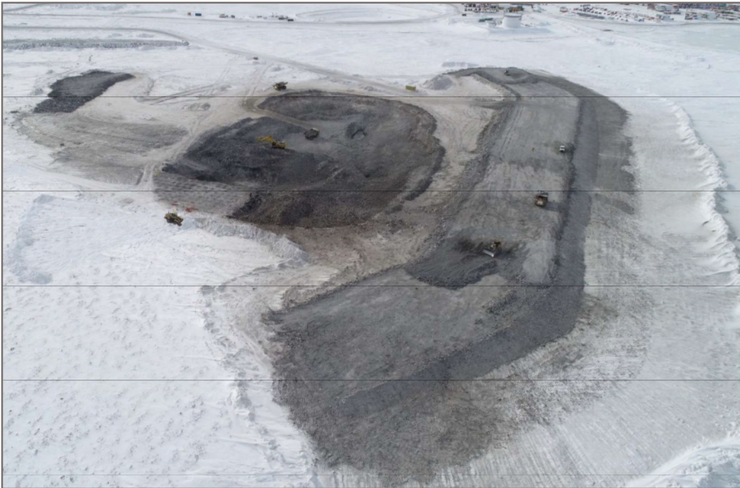
Photo 6: 2020-03-22 - Drone view of Pond CP6 and Berm CP6
