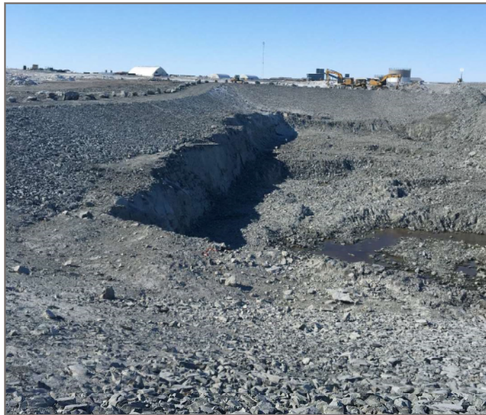
Photo 16: 2020-04-08 Pond CP6 - Final interior view of Pond CP6; view facing southwest
