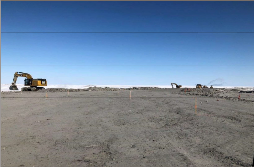
Photo 5: 2020-03-21 Berm CP6 - Sloping and building Berm CP6; view facing east
