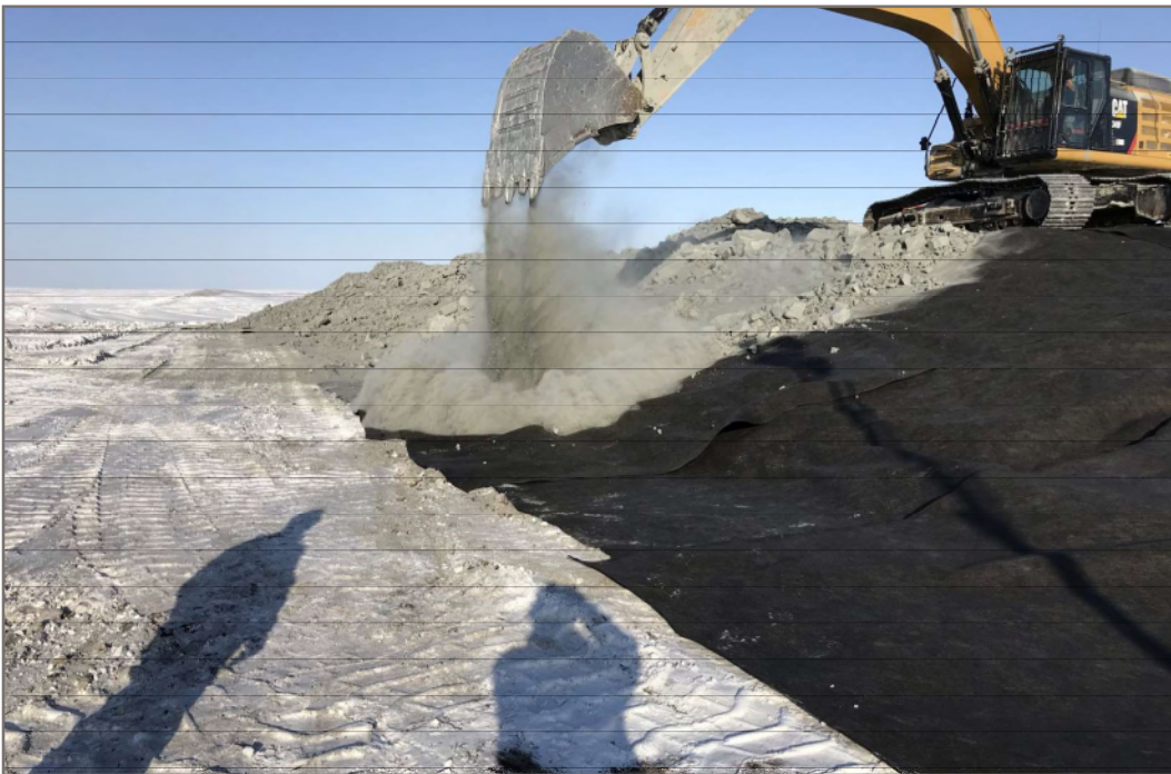
Photo 8: 2020-03-30 Berm CP6 - Placing erosion protection over geotextile on Berm CP6;; view facing northeast
