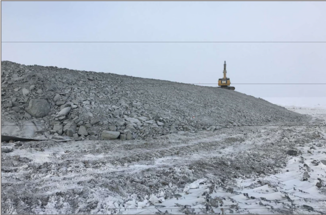
Photo 11: 2020-04-01 Berm CP6 - Sloping final erosion cover on Berm CP6; view facing southwest.
