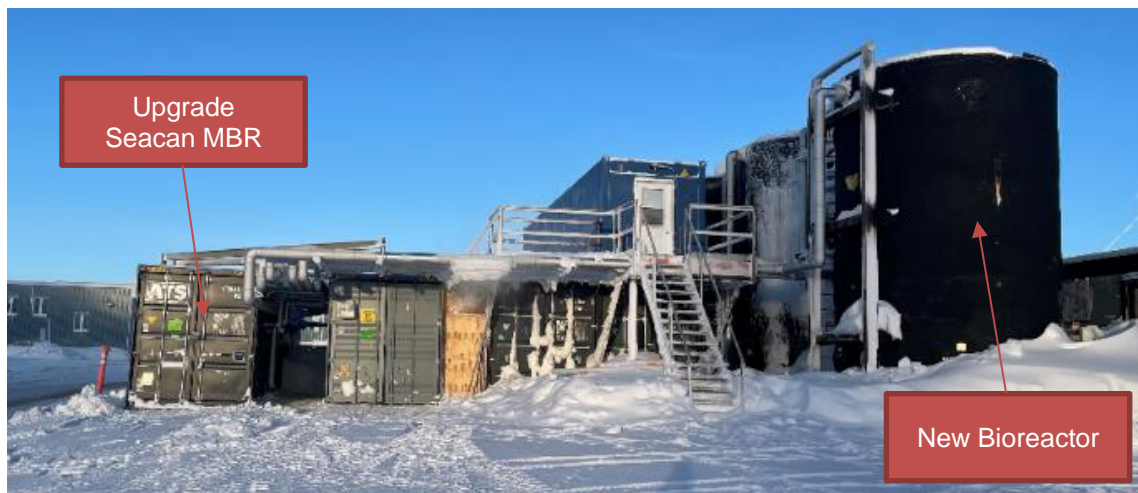
New Seacan and reactor
