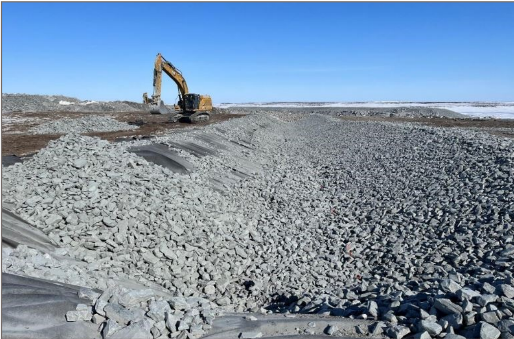
Photo 18: 2022-04-30 Channel10— Placing riprap on channel10; view facing north
