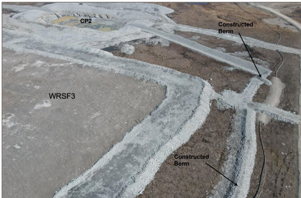
Photo 20: 2022-05-09 Channel10— Overview of constructed berms for channel10
