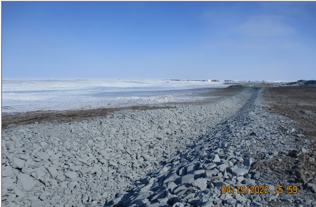
Photo 13: 2022-04-19 Channel9—Placement of rockfill before geotextile and riprap; view facing southeast
