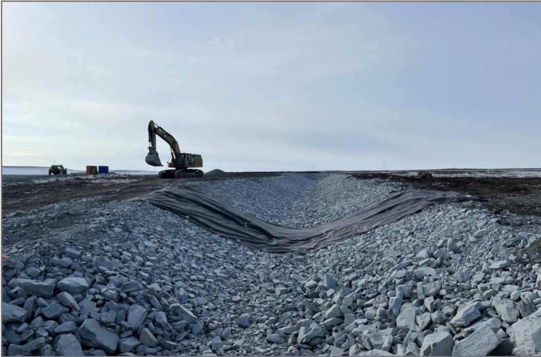
Photo 17: 2022-04-29 Channel10—Placing geotextile on channel10 after rockfill; view facing south
