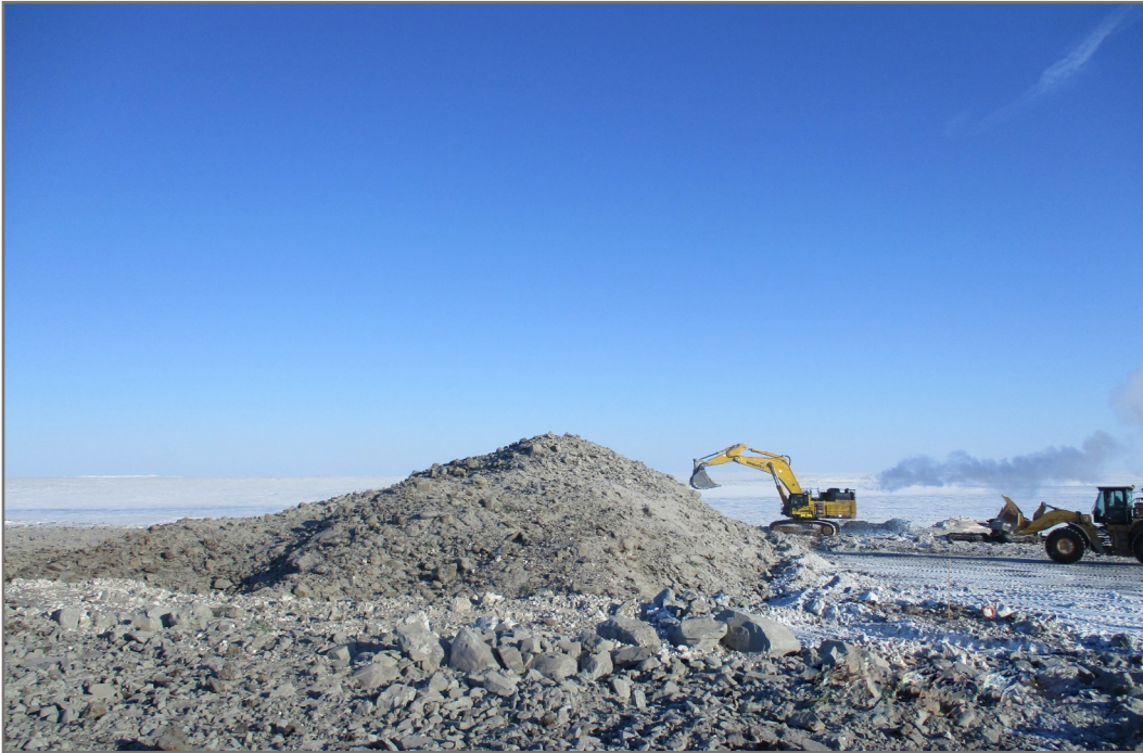
Photo 3: 2022-02-28 Pond CP2—Overburden being excavated from first blast; view facing east
