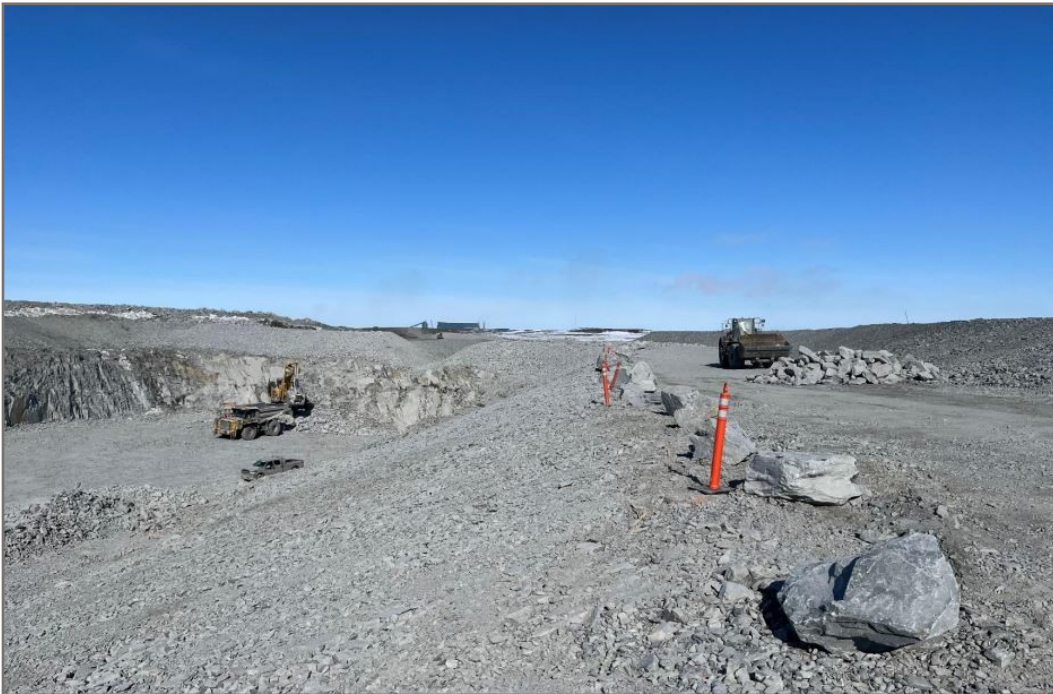
Photo 6: 2022-04-29 Pond CP2—Sloped rockfill for thermal protection; view facing north
