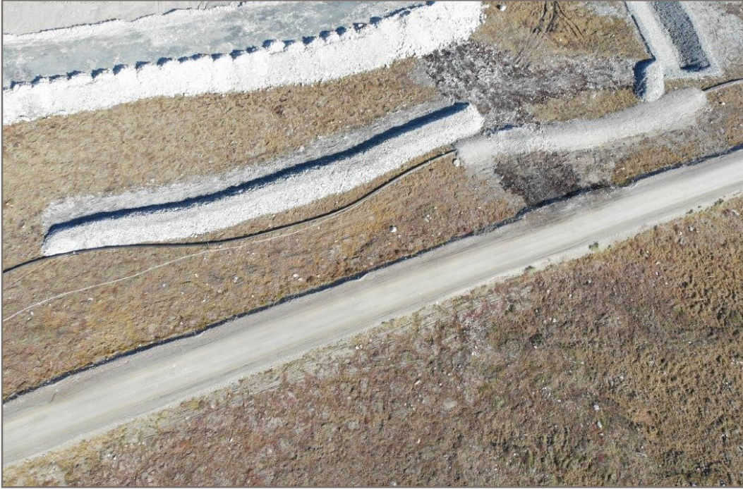
Photo 21: 2022-09-04 Channel10— Overview of constructed berms for channel10 with access road removed
