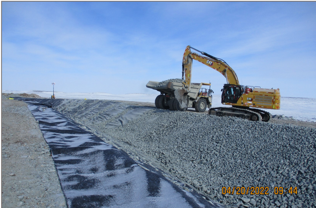
Photo 15: 2022-04-20 Channel9—Placing and sloping of riprap on geotextile; view facing northeast
