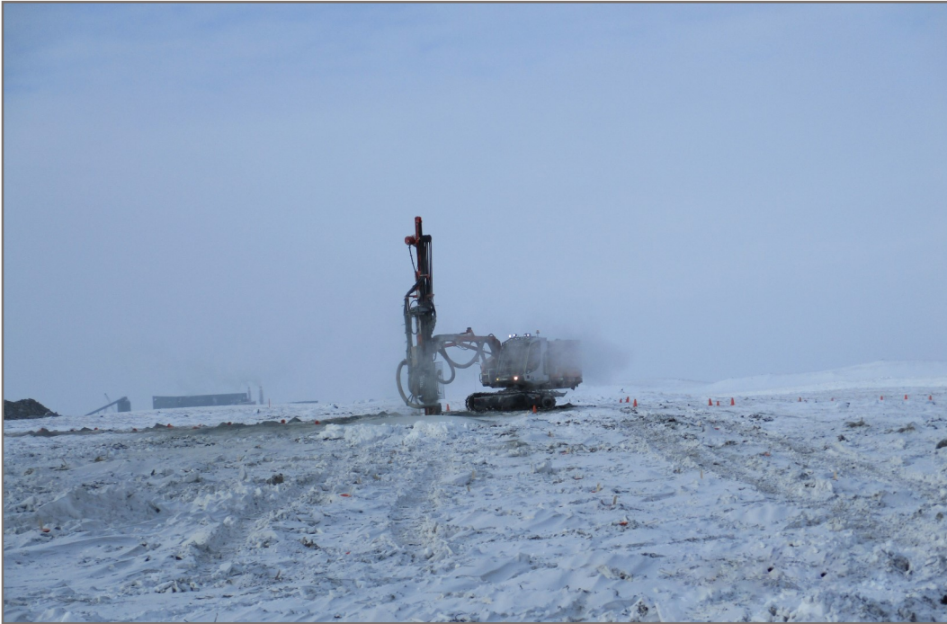
Photo 1: 2022-02-25 Pond CP2—Drilling first blast pattern; view facing north
