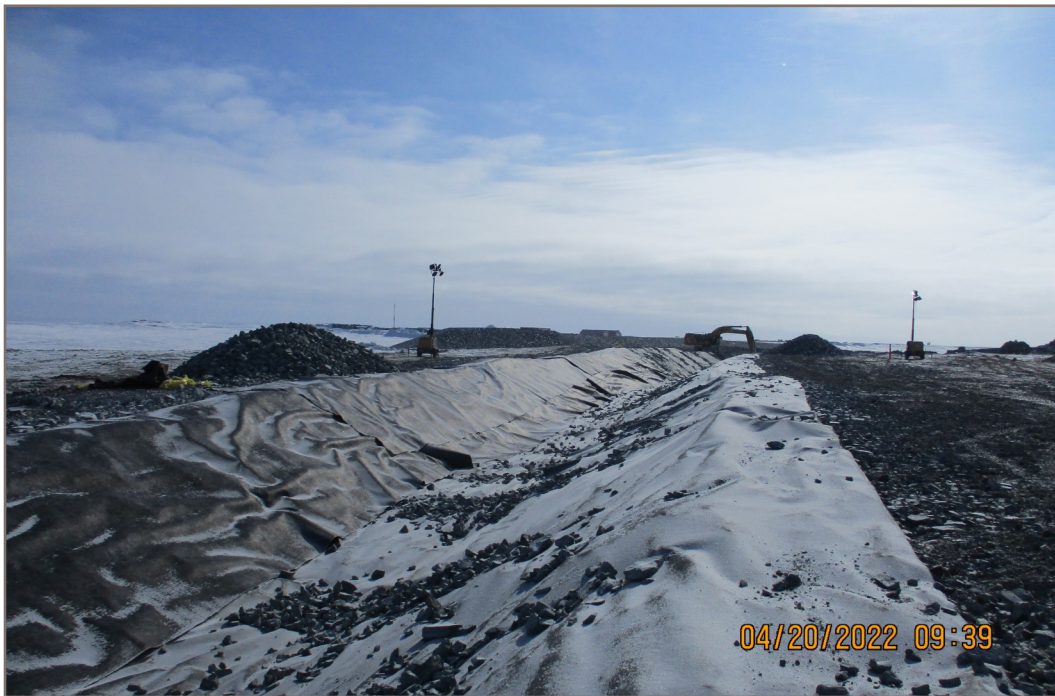
Photo 14: 2022-04-20 Channel9—Placement of geotextile; view facing south
