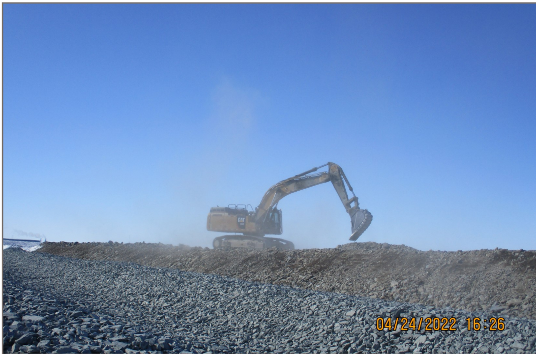
Photo 16: 2022-04-24 Channel9—Overburden fill placement of channel9 berm; view facing northeast
