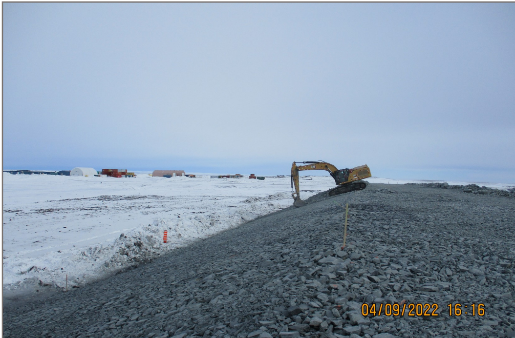
Photo 11: 2022-04-09 Berm CP2—Sloping of rockfill on berm; view facing south
