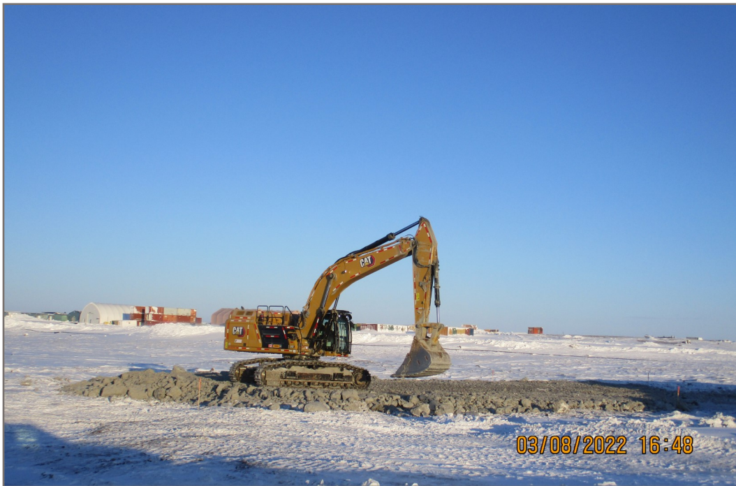
Photo 8: 2022-03-08 Berm CP2—First lift of overburden till; view facing southeast
