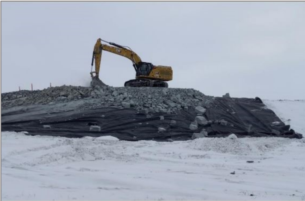
Photo 10: 2022-03-23 Berm CP2—Placing of geotextile and rockfill; view facing west
