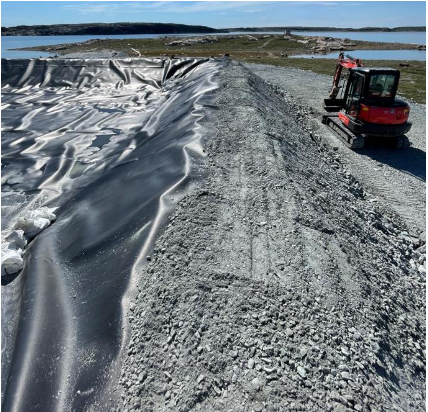
01-08-2024 Installed Liner System in the Drilling Mud Recirculation, North side
