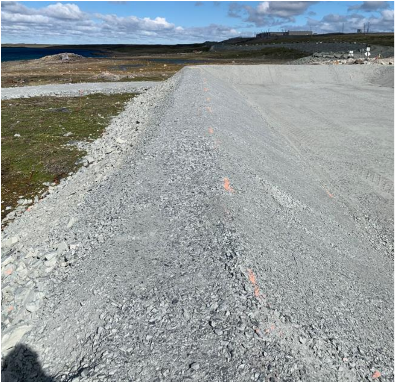
07-07-2024 Under Liner Material Placement of the Lined Containment Area, West Side
