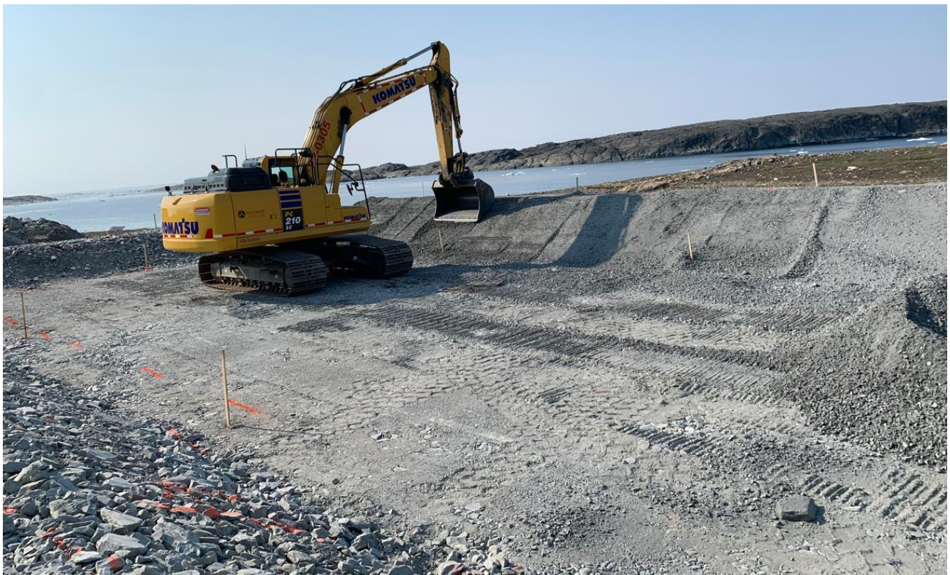
04-07-2024 30 mm minus Under Liner Material Placement of the Lined Containment Area
