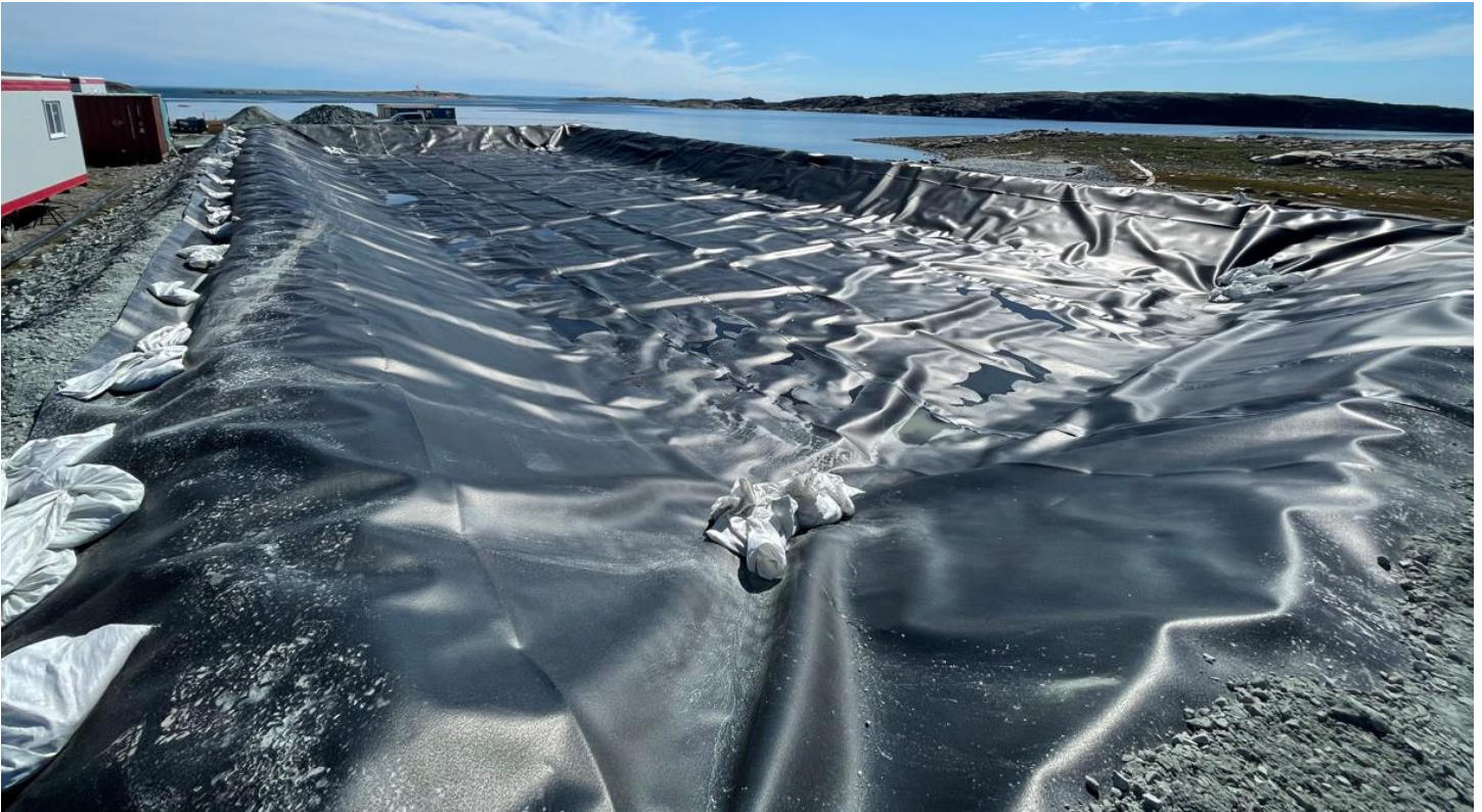
01-08-2024 Installed Liner System in the Drilling Mud Recirculation
