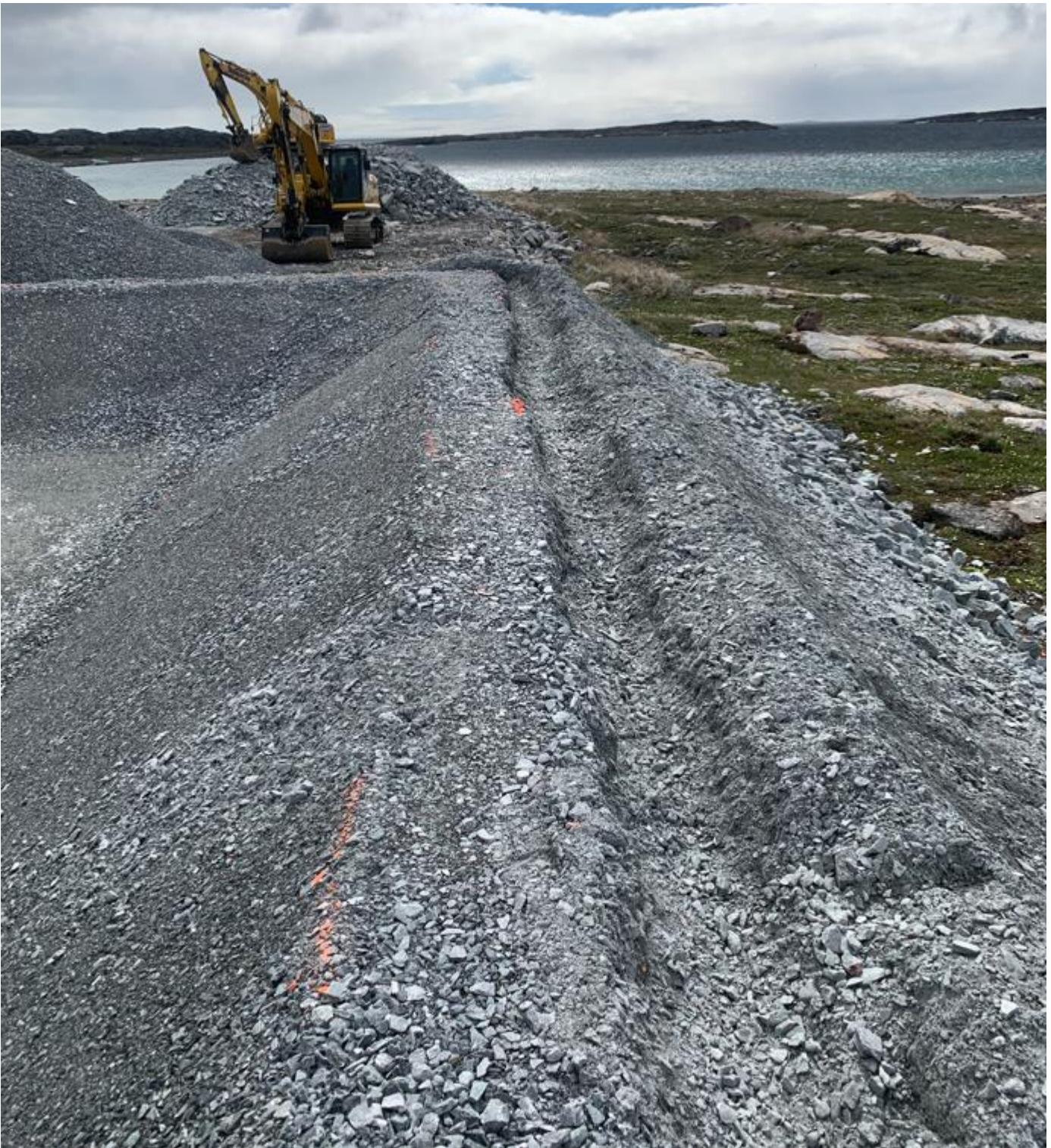
07-07-2024 Key Trench for Under Liner Material of the Lined Containment Area
