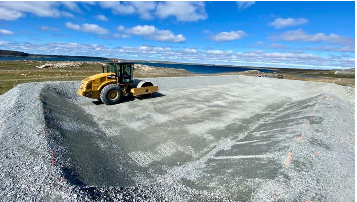
06-07-2024 Roller Packer over 30 mm minus Under Liner Material of the Lined Containment Area
