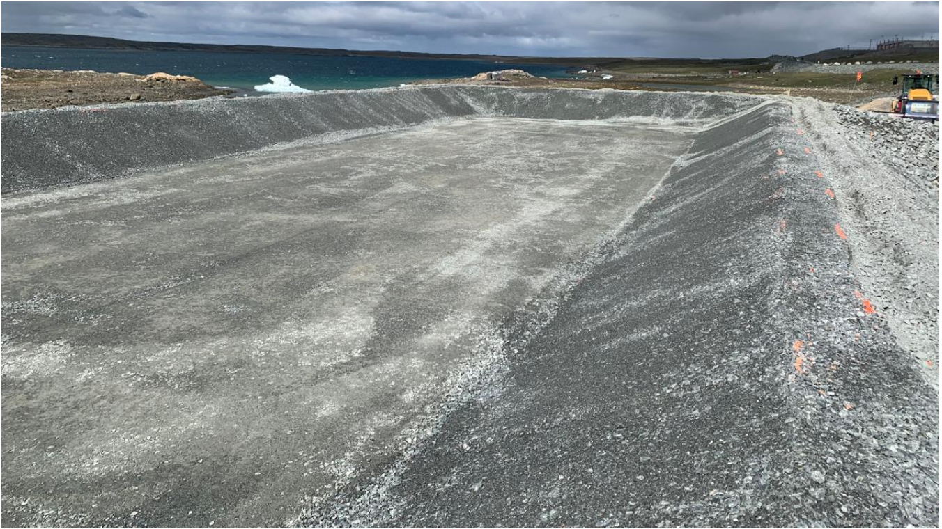
07-07-2024 Key Trench for Under Liner Material of the Lined Containment Area
