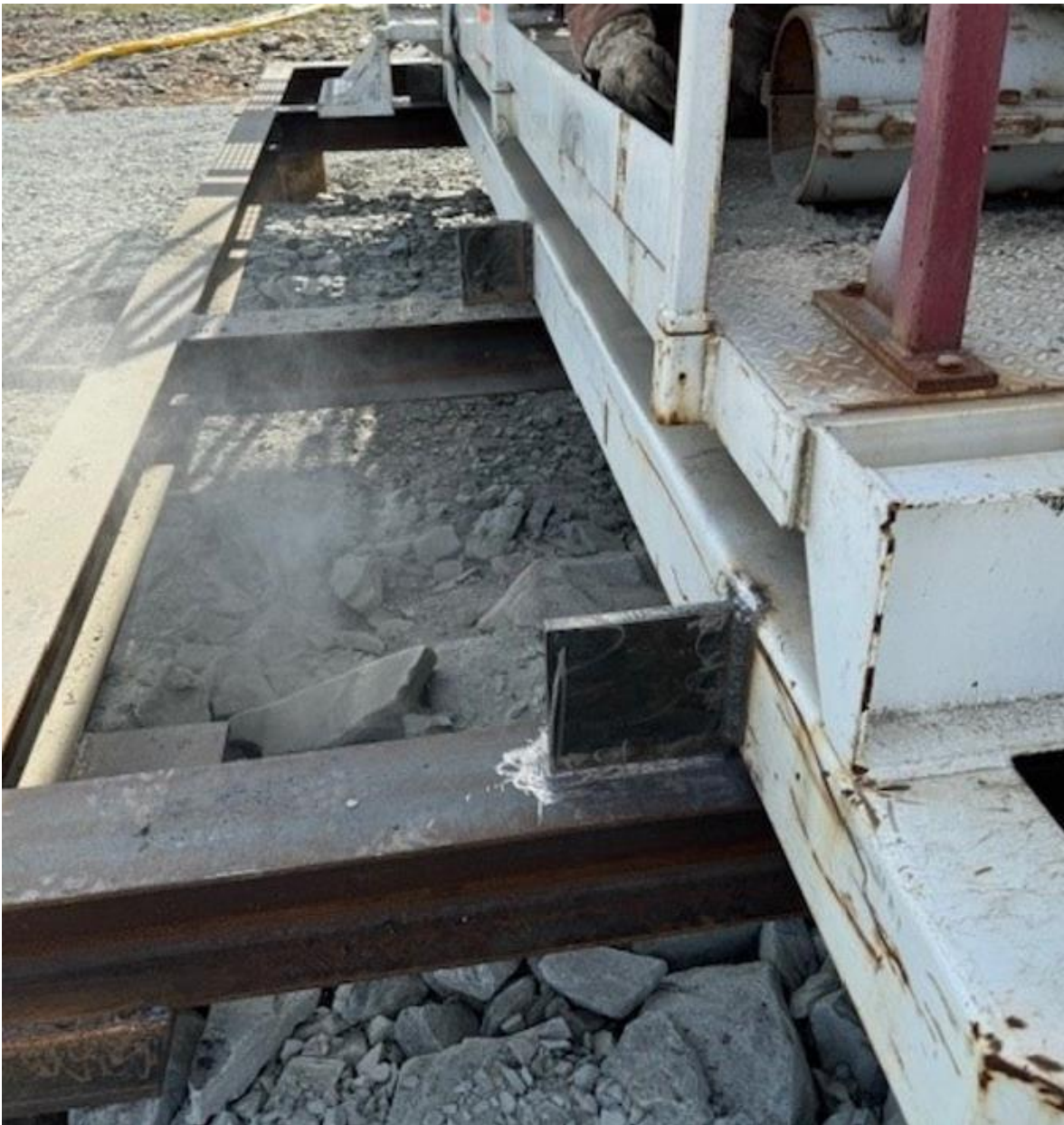
18-08-2024 Welding the Drill Platform to the Steel Frame
