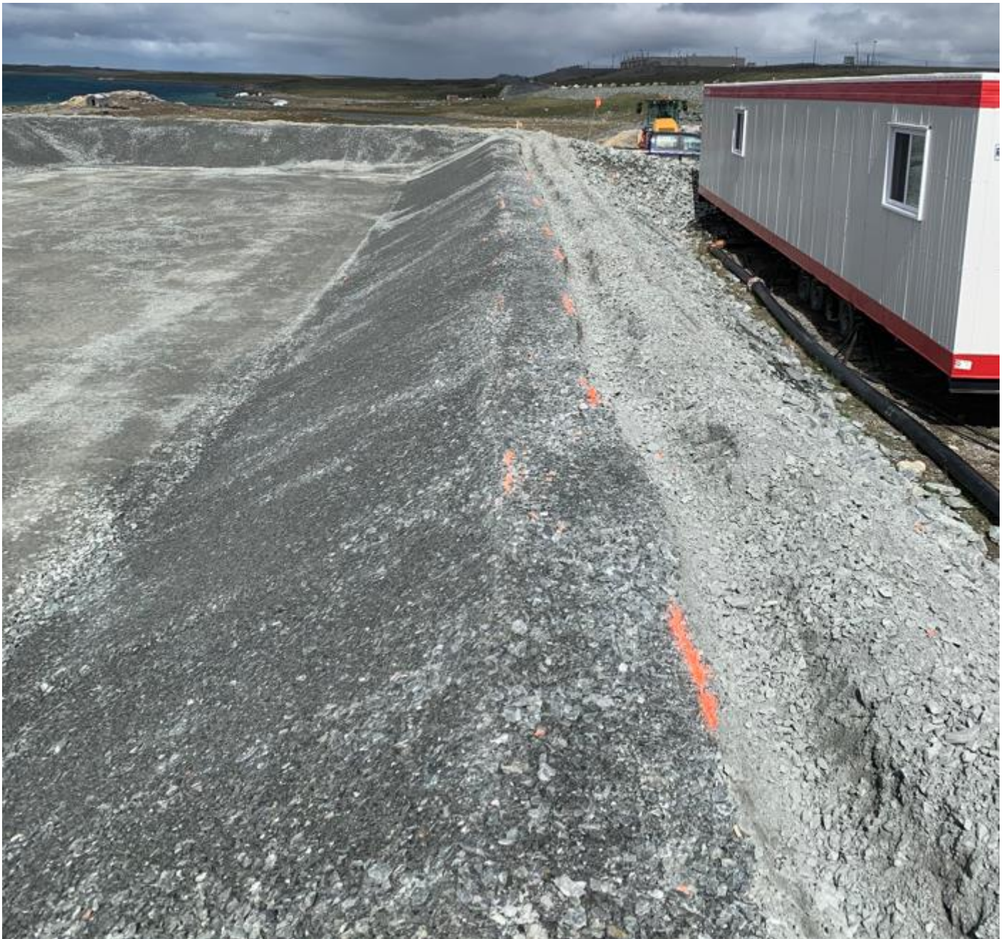
07-07-2024 Key Trench for Under Liner Material of the Lined Containment Area
