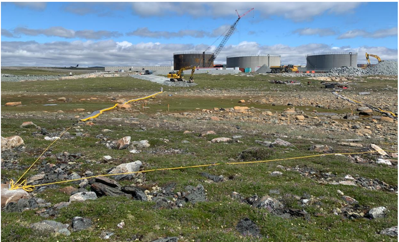
10-07-2024 Silt Curtain Prevent Erosion of Construction Material and Mix with Nature
