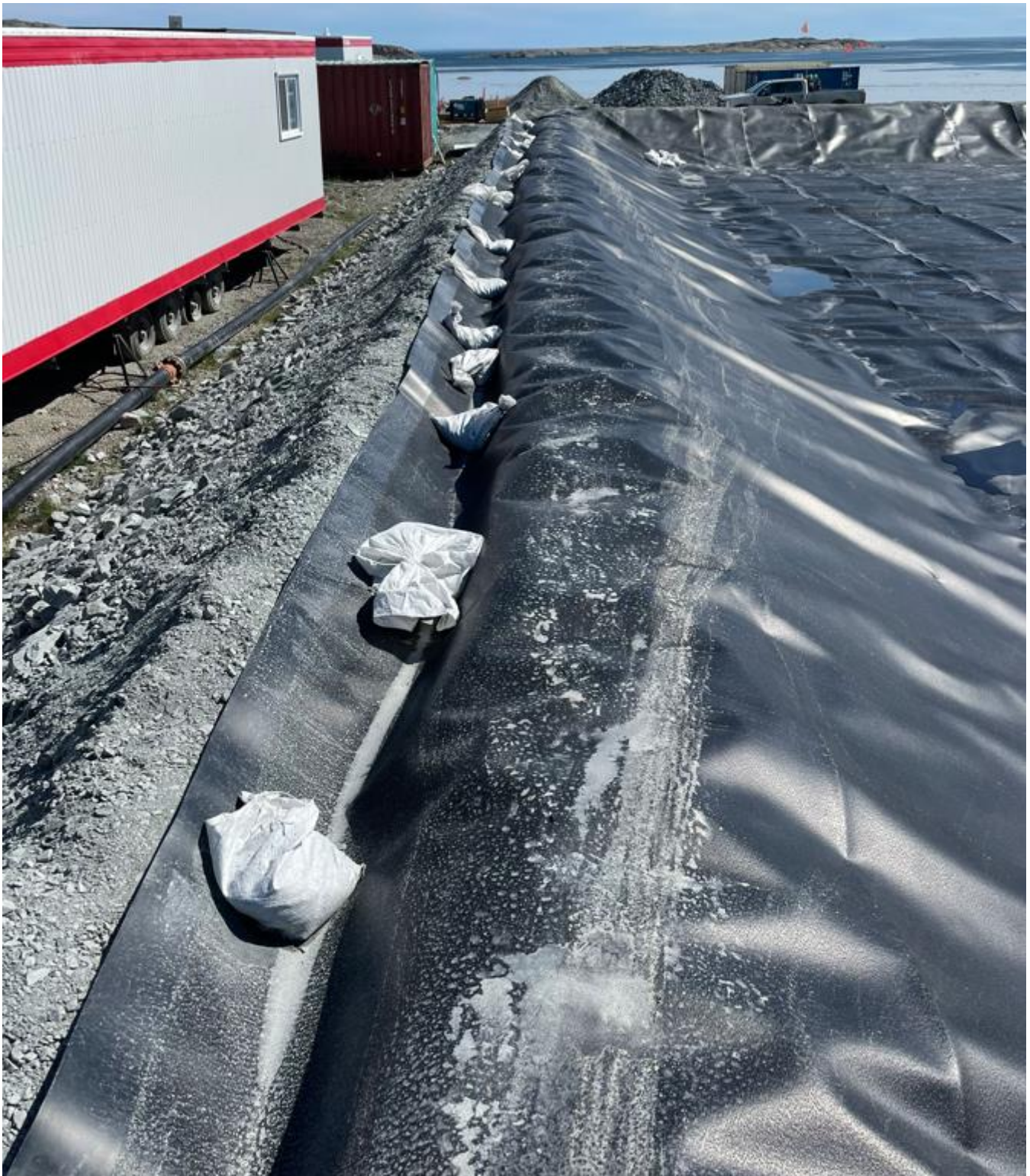
01-08-2024 Installed Liner System in the Drilling Mud Recirculation, East side
