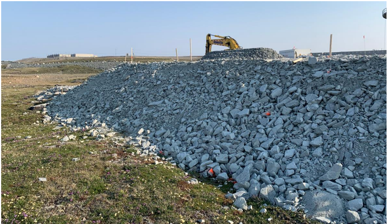
04-07-2024 Under Liner Material Placement of the Lined Containment Area
