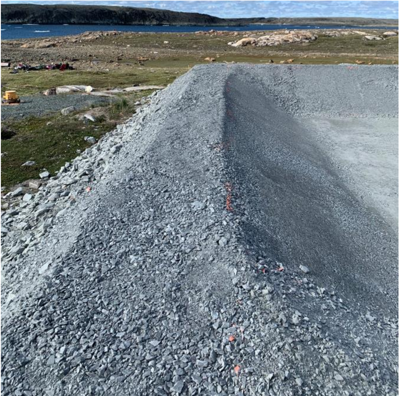
06-07-2024 Under Liner Material Placement of the Lined Containment Area, South Side
