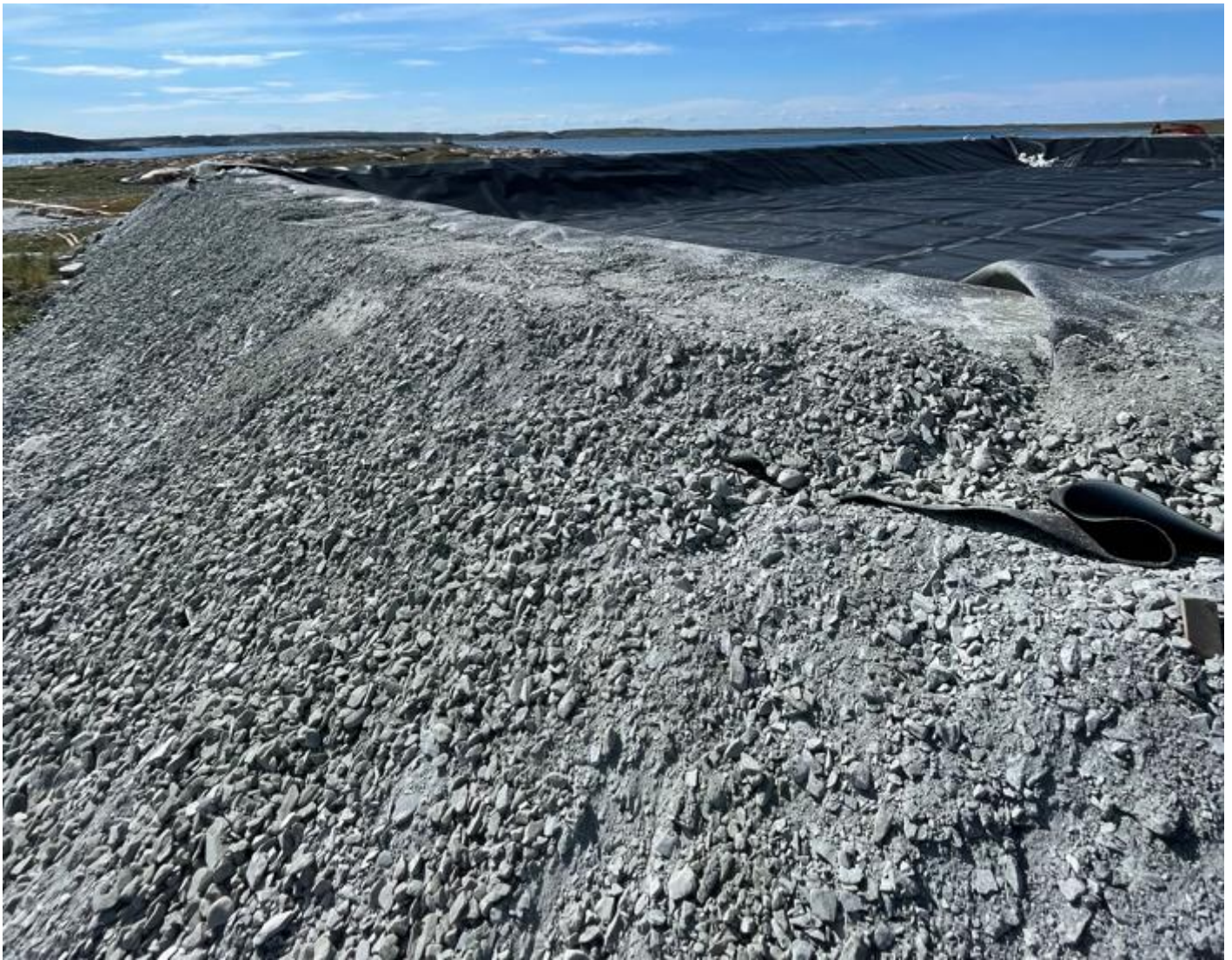
01-08-2024 Installed Liner System in the Drilling Mud Recirculation, South side
