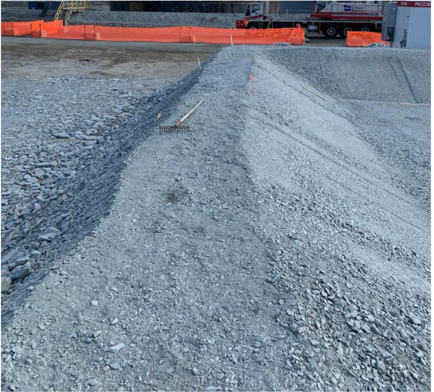
07-07-2024 Under Liner Material Placement of the Lined Containment Area, North Side
