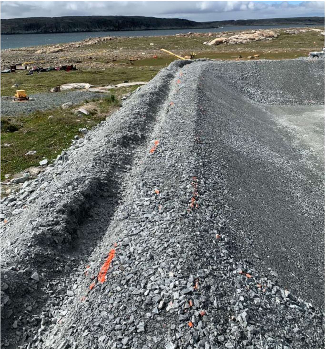
07-07-2024 Key Trench for Under Liner Material of the Lined Containment Area
