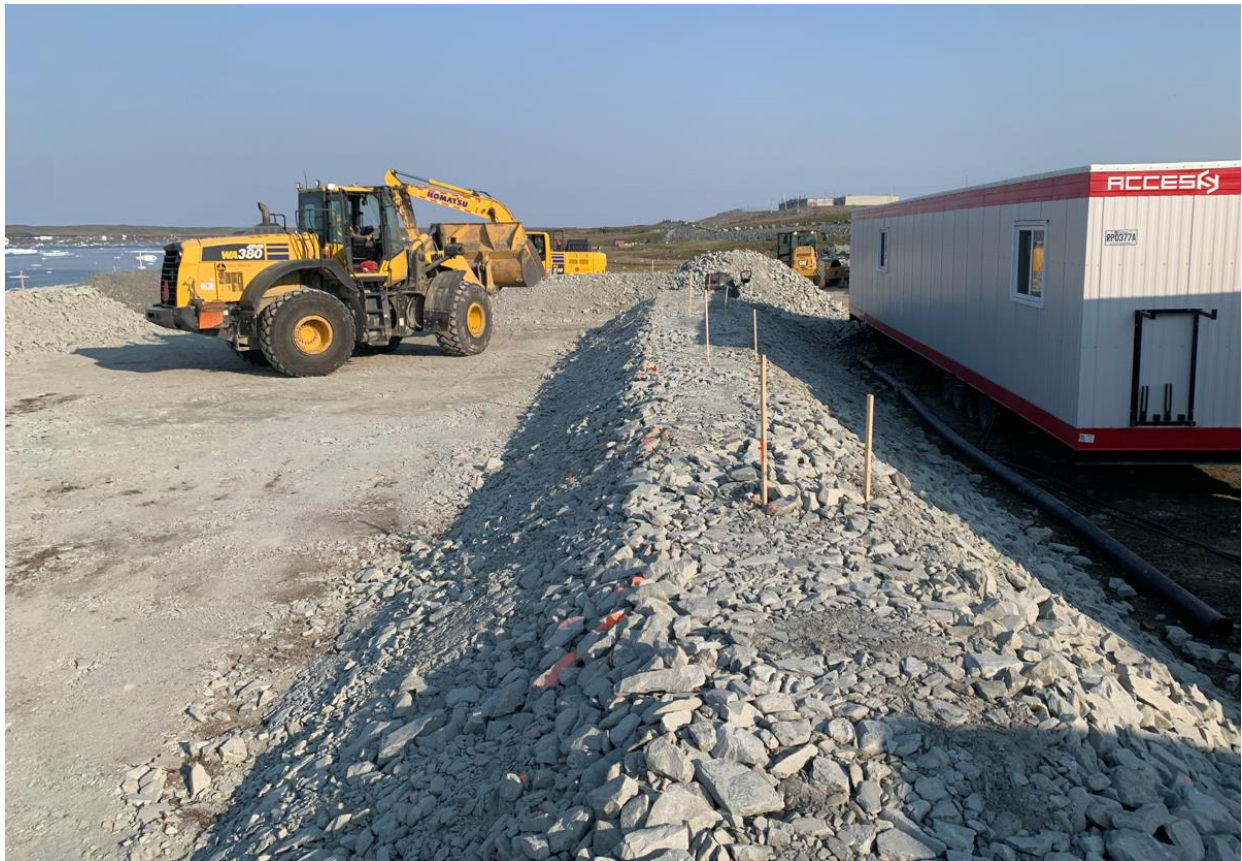
04-07-2024 150 mm minus Under Liner Material Placement of the Lined Containment Area, East Side
