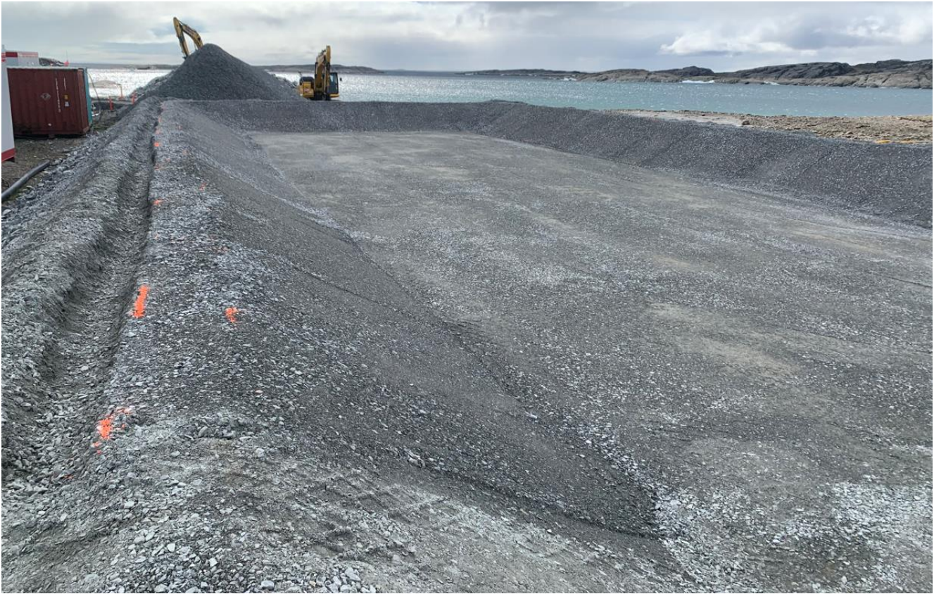
07-07-2024 Under Liner Material Placement of the Lined Containment Area
