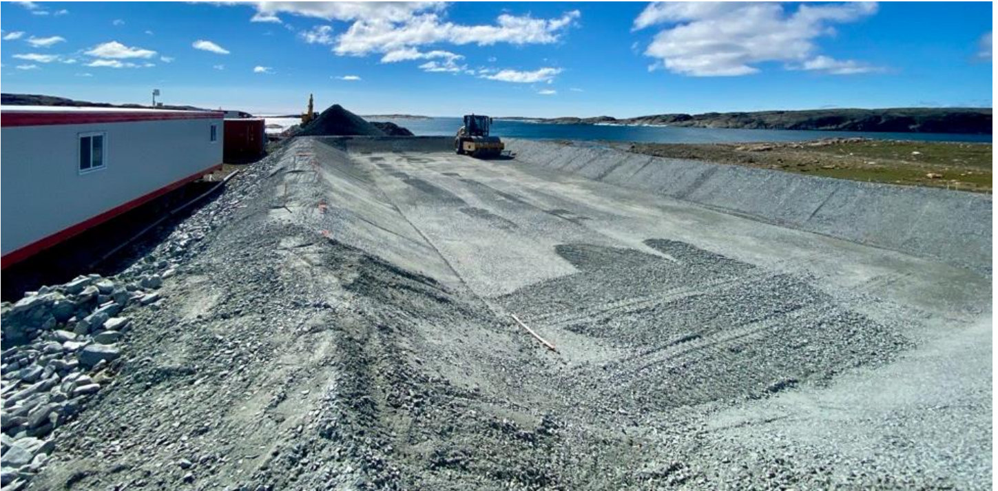
06-07-2024 Roller Packer over 30 mm minus Under Liner Material of the Lined Containment Area
