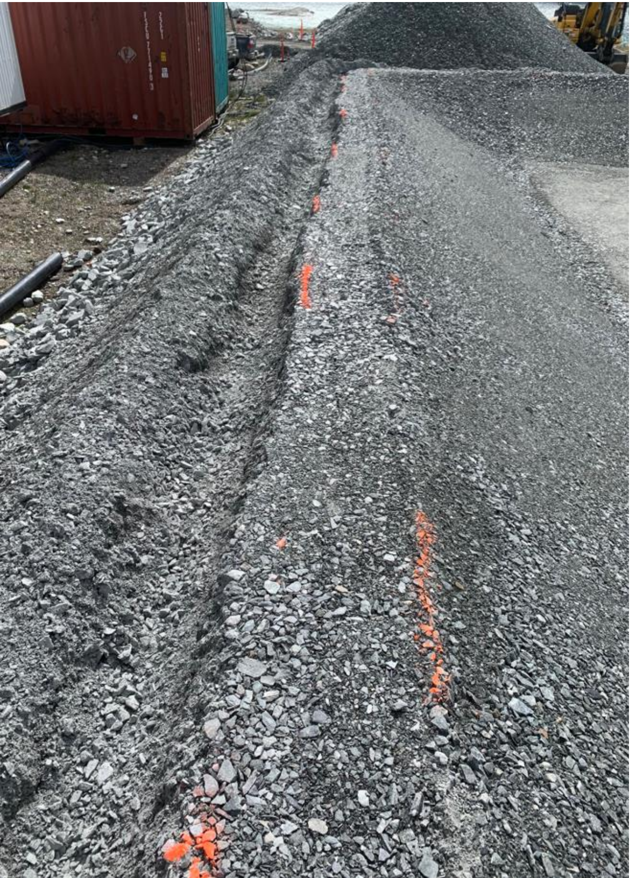
07-07-2024 Key Trench for Under Liner Material of the Lined Containment Area
