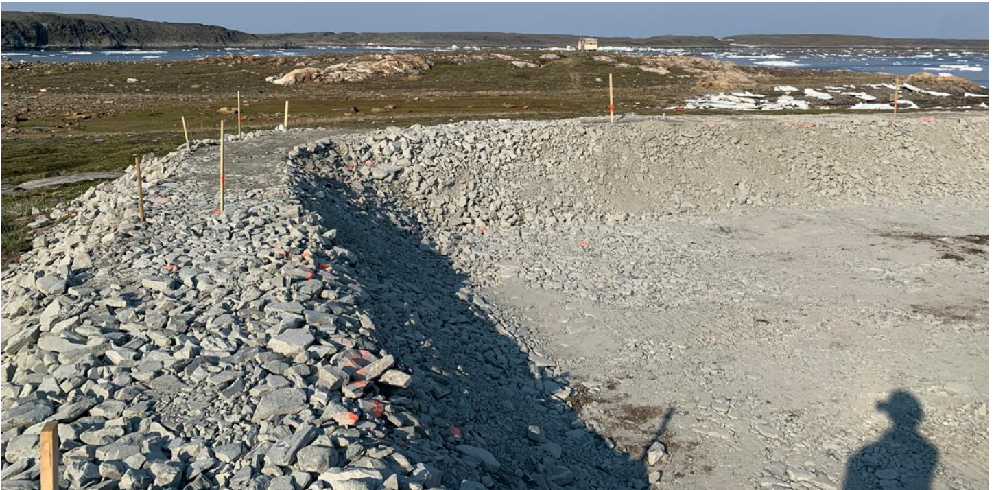
04-07-2024 150 mm minus Under Liner Material Placement of the Lined Containment Area, Southwest Corner
