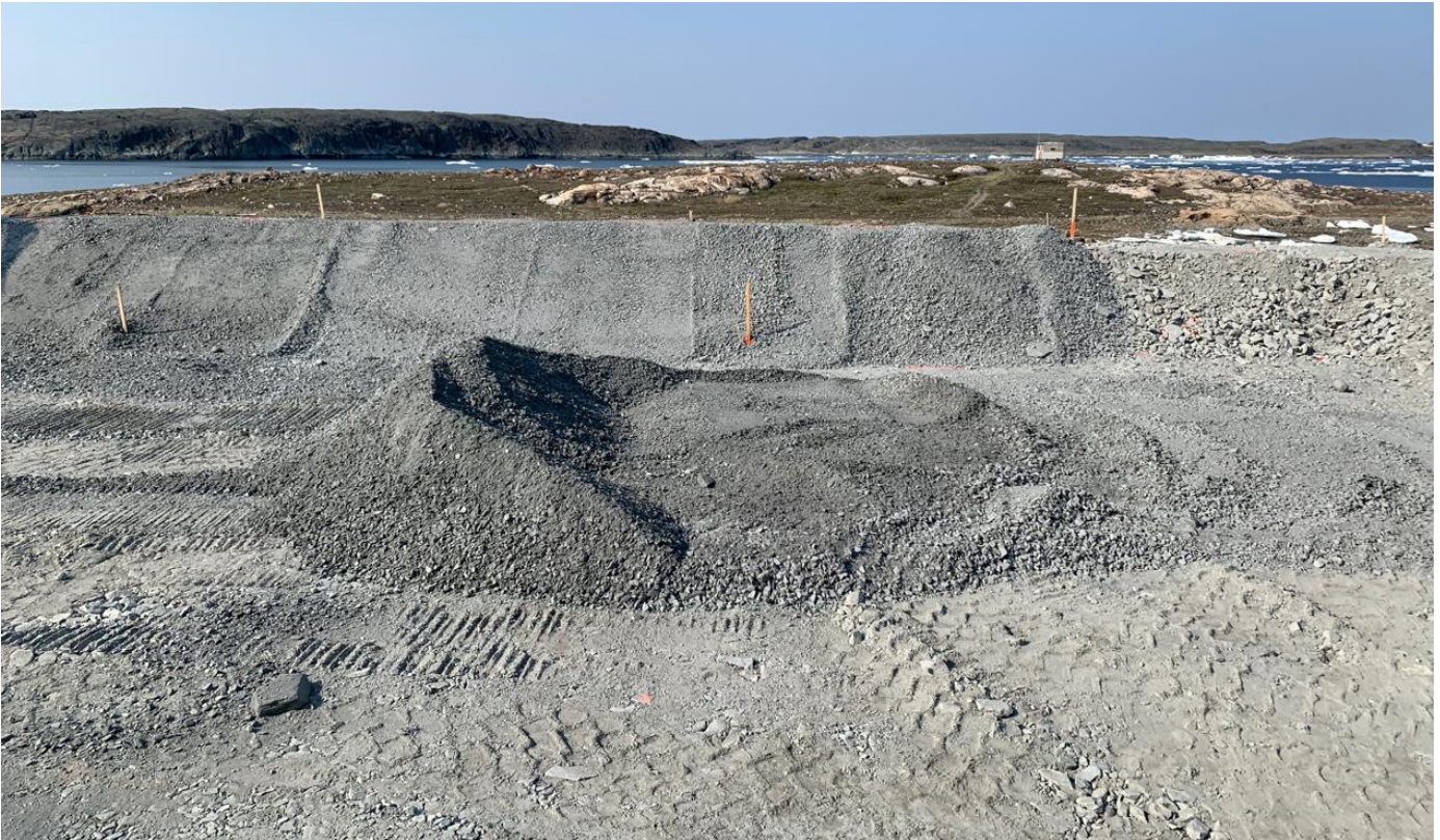
04-07-2024 30 mm minus Under Liner Material Placement of the Lined Containment Area
