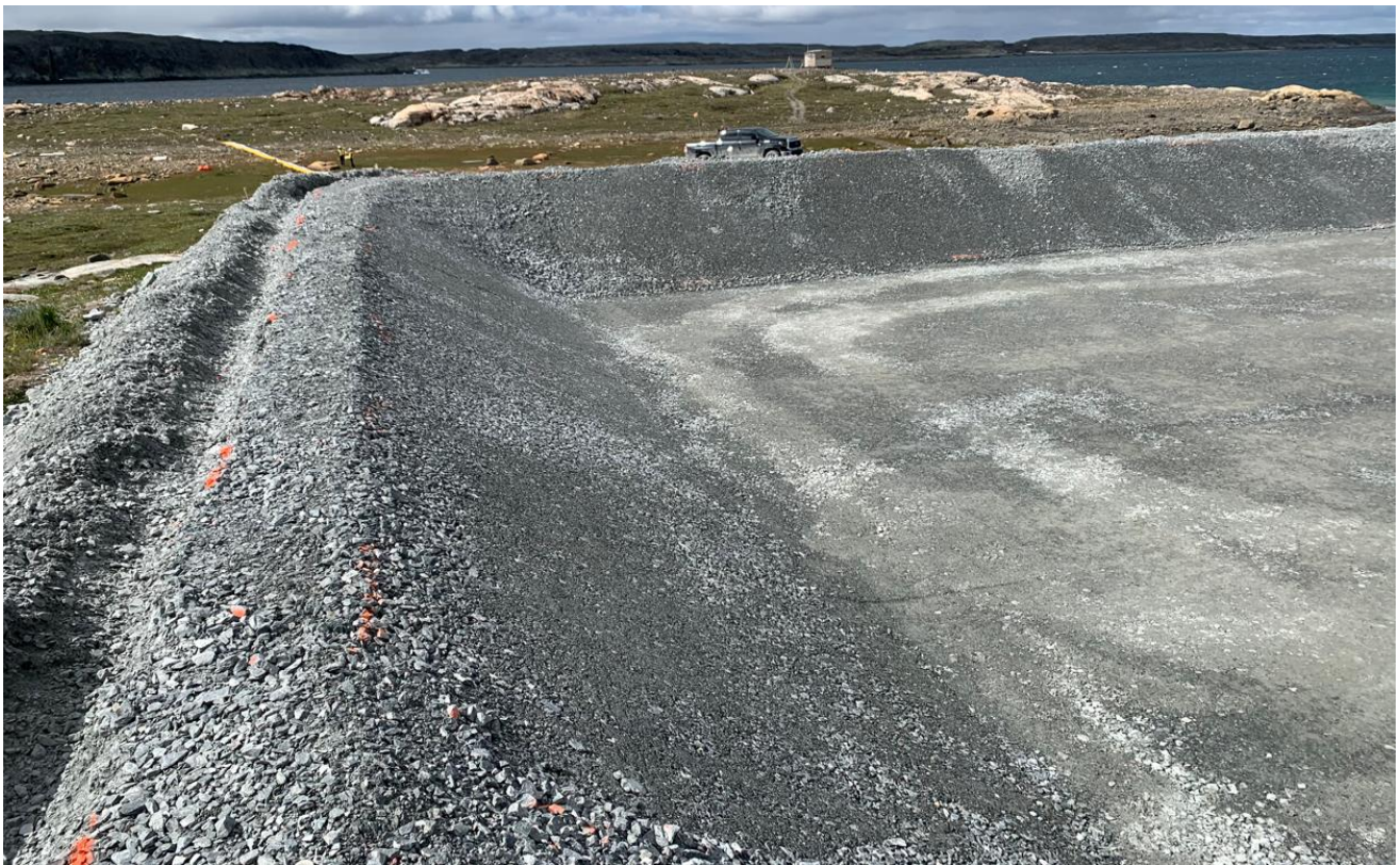
07-07-2024 Key Trench for Under Liner Material of the Lined Containment Area
