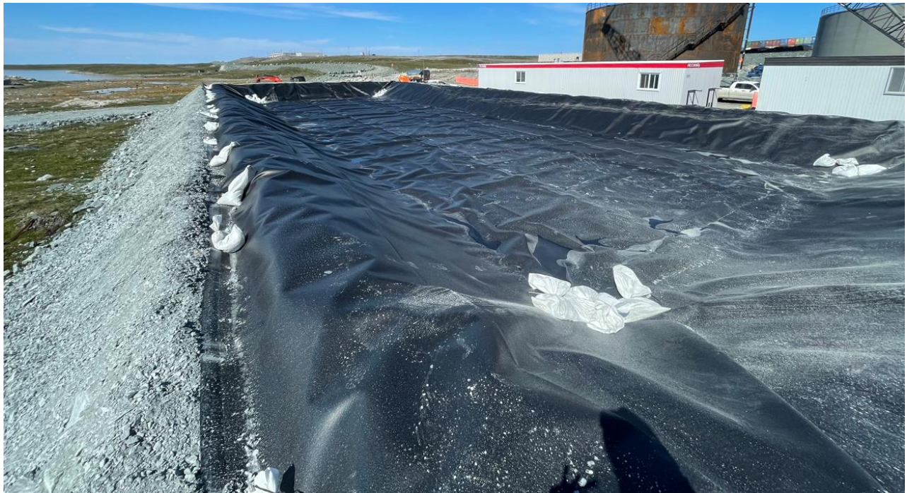
01-08-2024 Installed Liner System in the Drilling Mud Recirculation, West side
