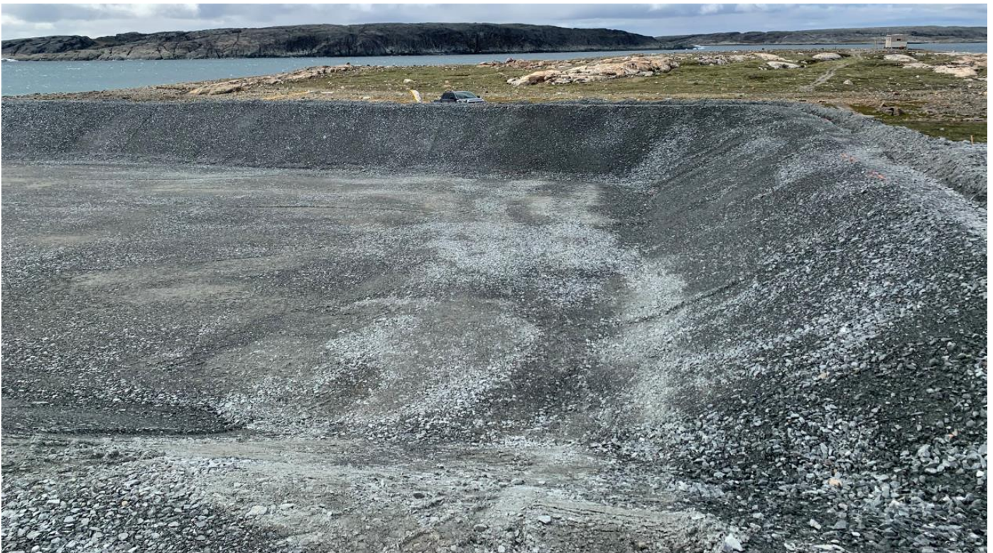
07-07-2024 Under Liner Material Placement of the Lined Containment Area
