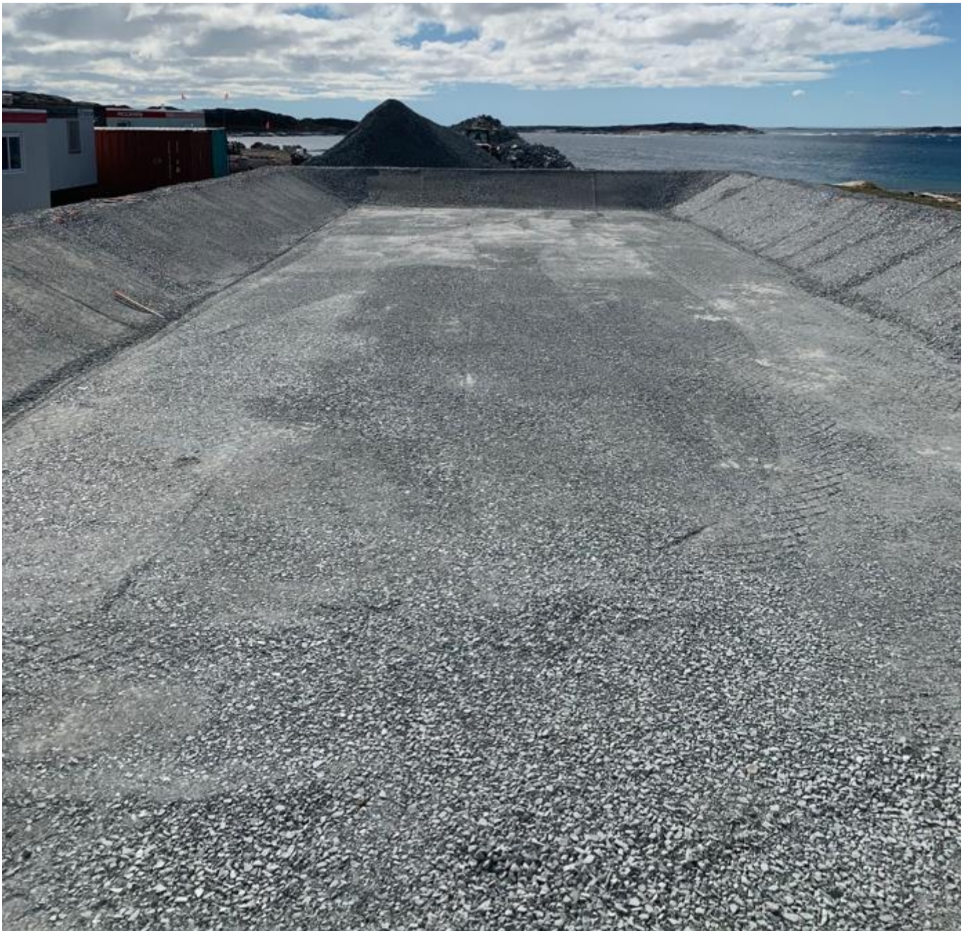
07-07-2024 Under Liner Material Placement of the Lined Containment Area
