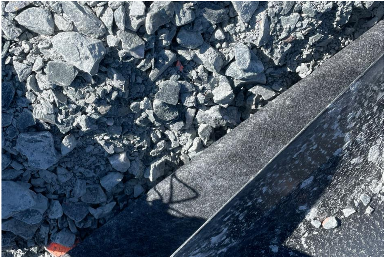
01-08-2024 Geotextile under the Membrane in the Drilling Mud Recirculation
