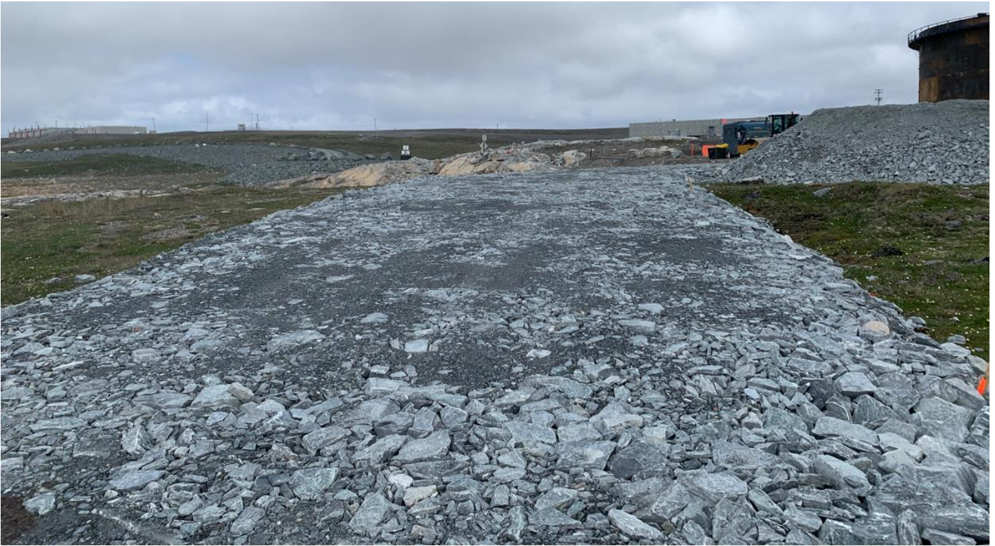
07-07-2024 600 minus of Access Road after Packing
