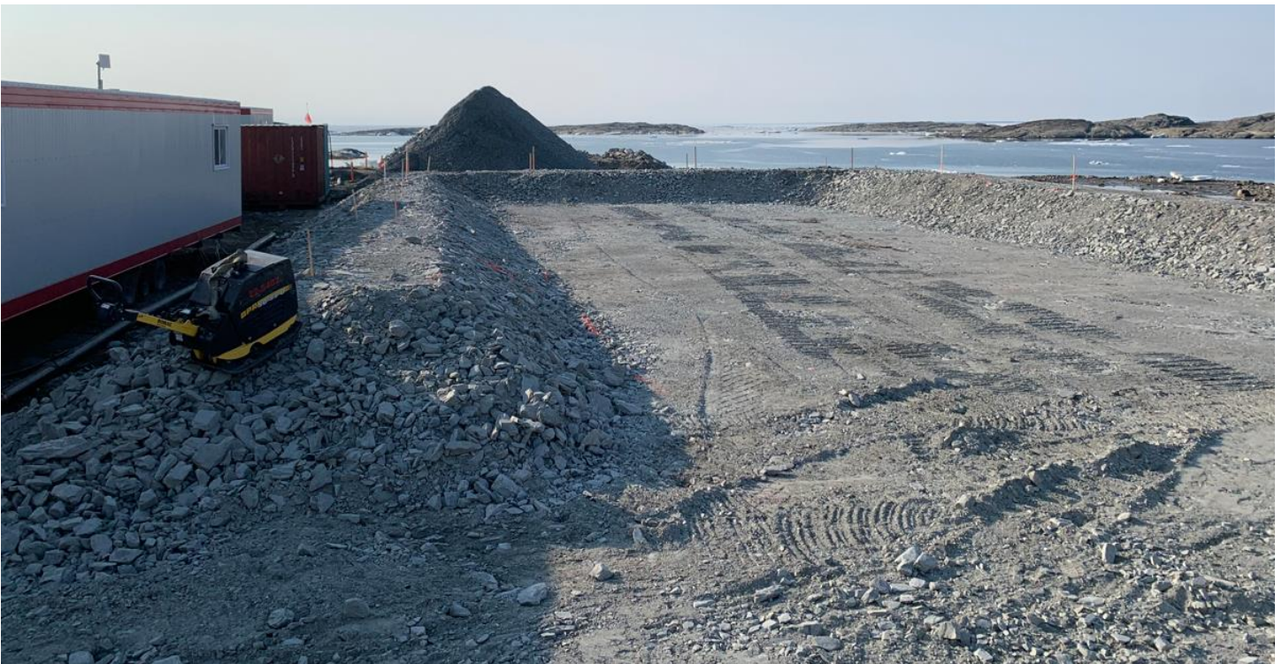
04-07-2024 150 mm minus Under Liner Material Placement of the Lined Containment Area
