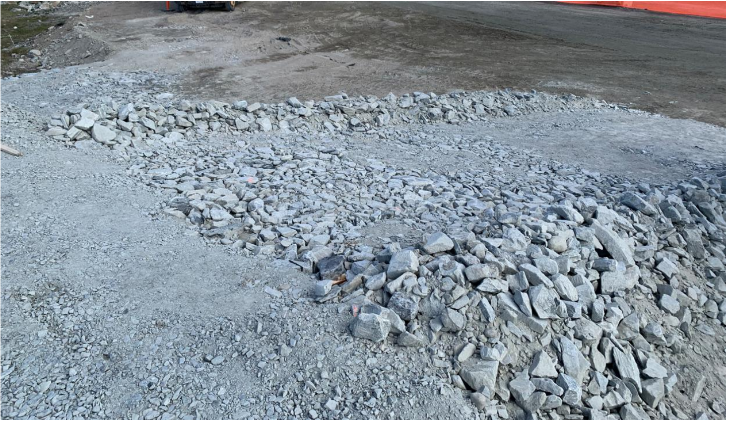
07-07-2024 Temporary Ramp to Access the Lined Containment Area, East Side
