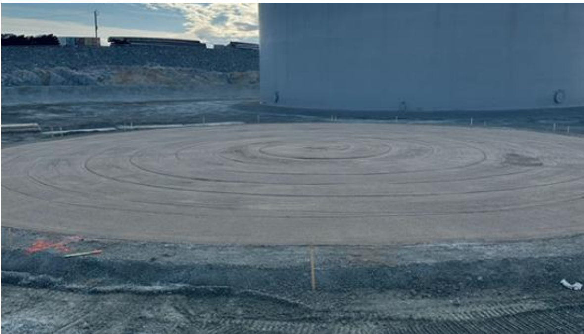
11-06-2024 Placement of Sand on the 9ML Tank Pad
