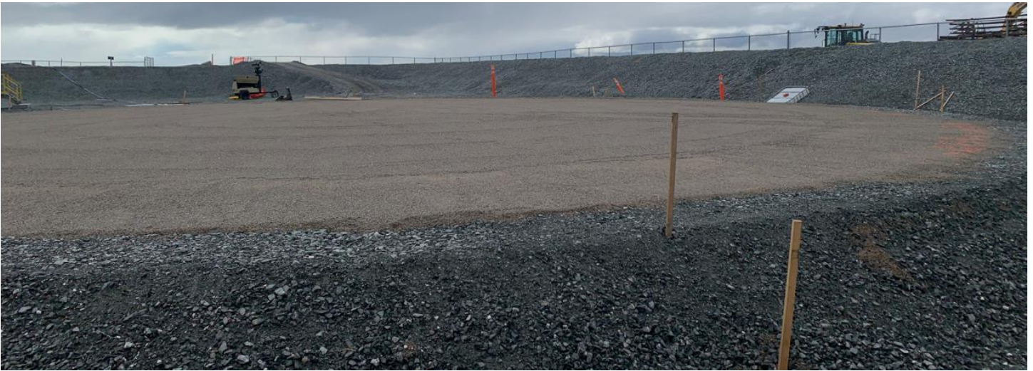
07-07-2024 4.5ML Tank Pad before Tank Erection
