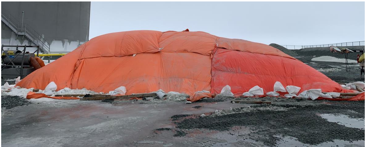
30-04-2024 Thawing Ice and Pumping out the Water at 4.5ML Tank Pad
