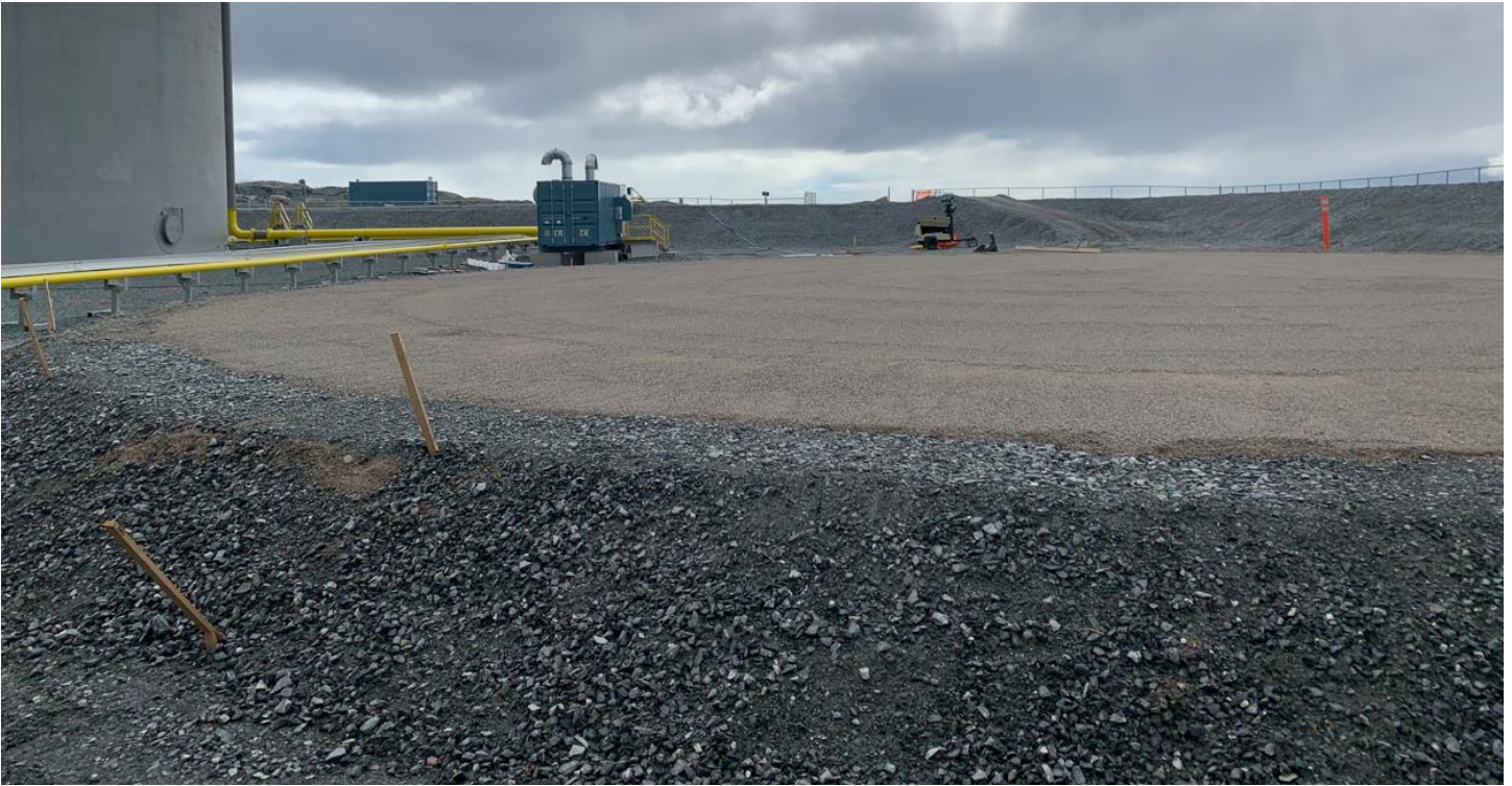
07-07-2024 4.5ML Tank Pad before Tank Erection
