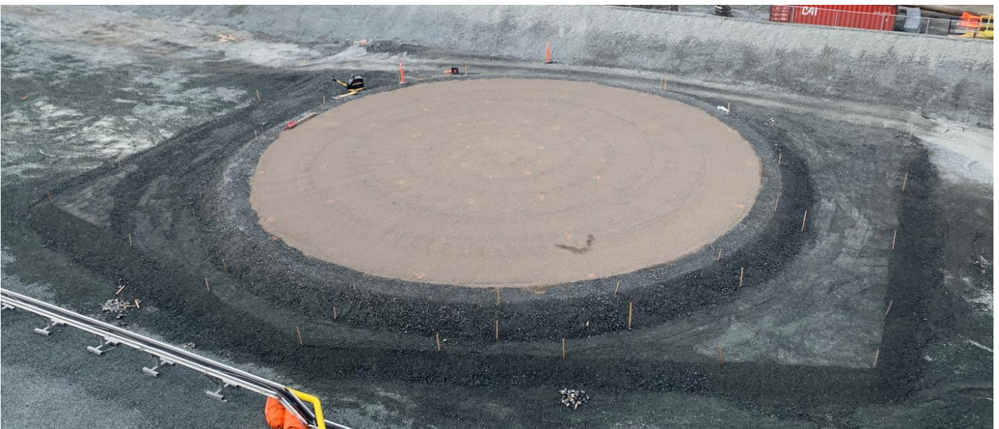
29-06-2024 4.5ML Tank Pad (fine tuning of sand not completed yet)
