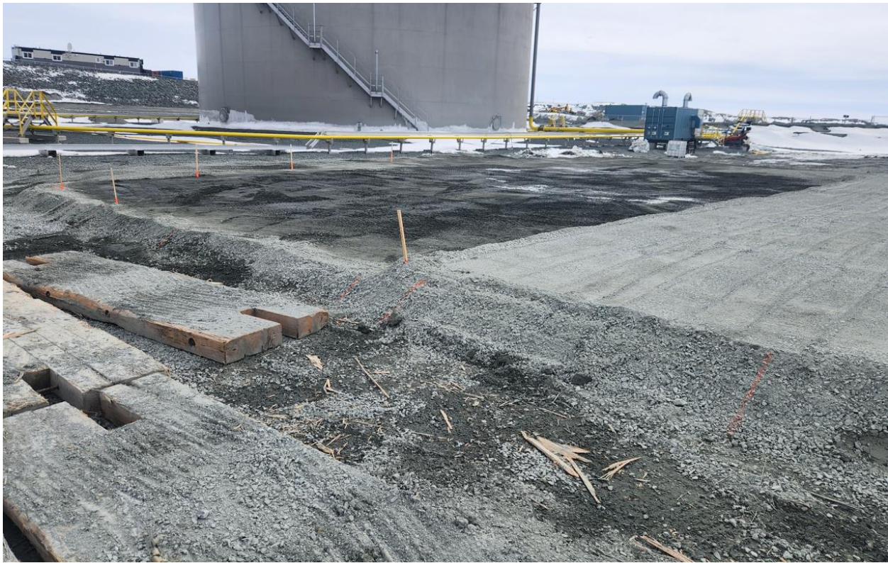
16-05-2024 First and Second Lift of 30 mm minus on 4.5ML Tank Pad
