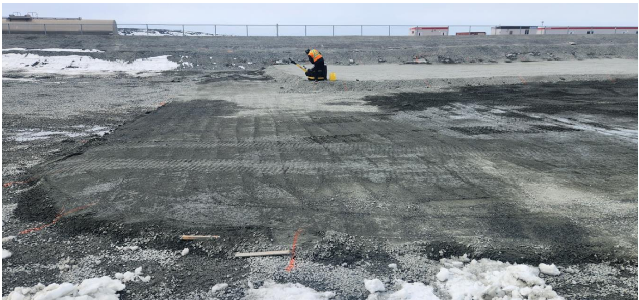
16-05-2024 First and Second Lift of 30 mm minus on 4.5ML Tank Pad
