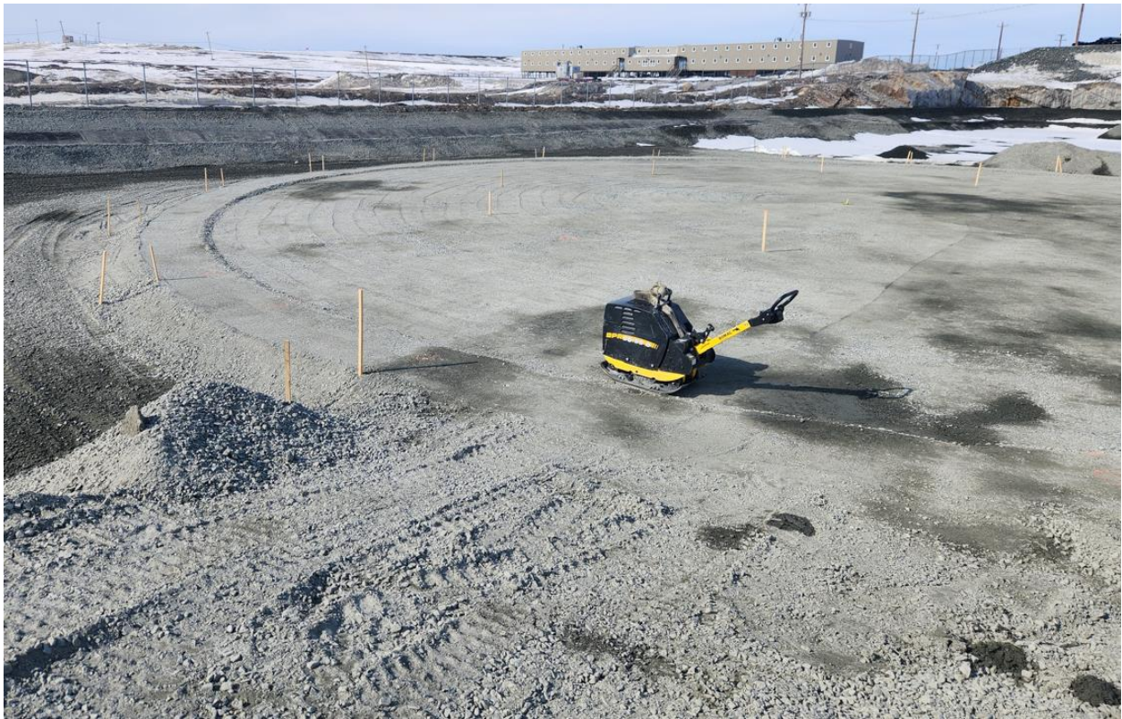
15-05-2024 Final Grade of 30 mm minus material on 9ML Tank Pad
