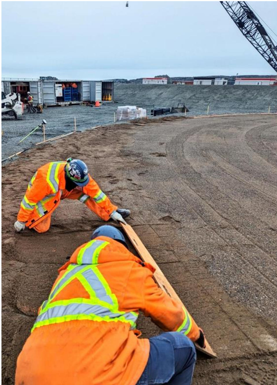
17-06-2024 Fine Tuning of Sand on 9ML Tank Pad before Tank Erection
