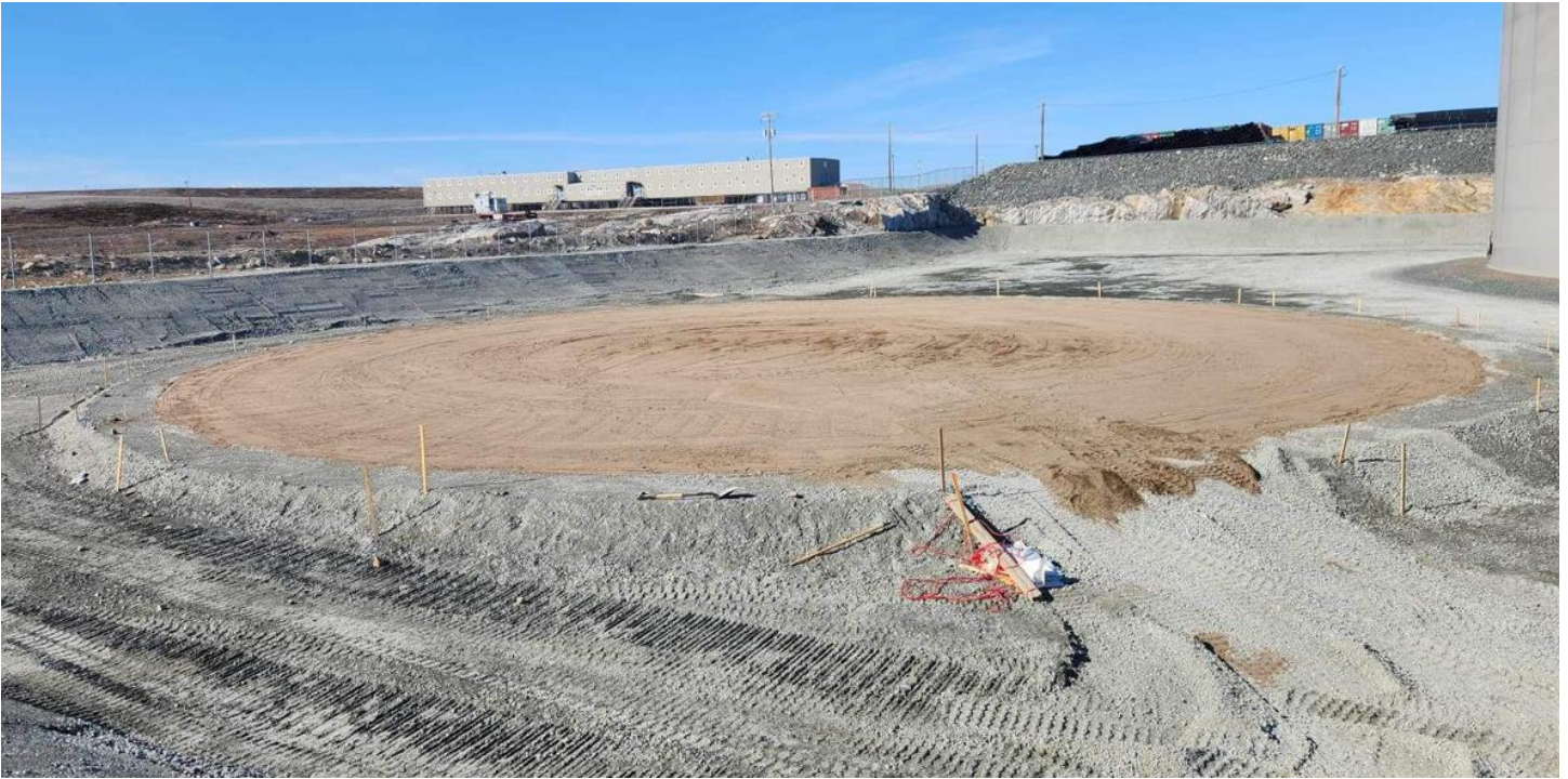
11-06-2024 Placement of Sand on the 9ML Tank Pad
