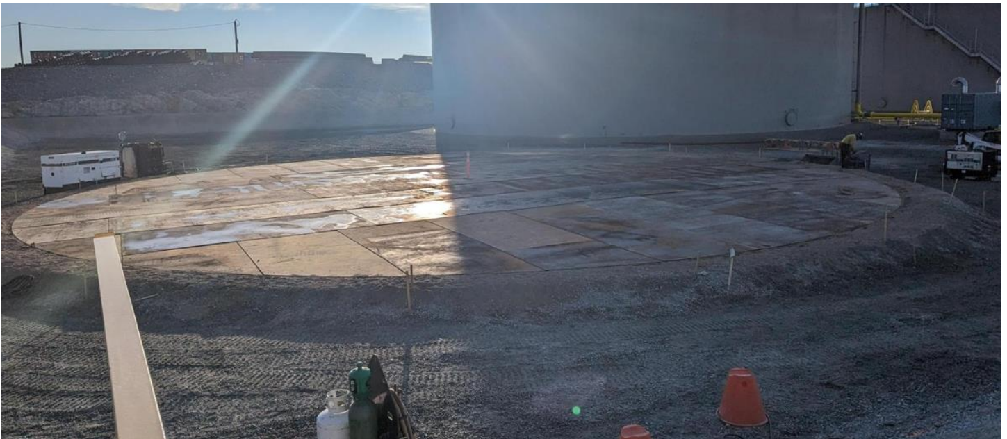
17-06-2024 Base Layer of 9ML Tank Installed
