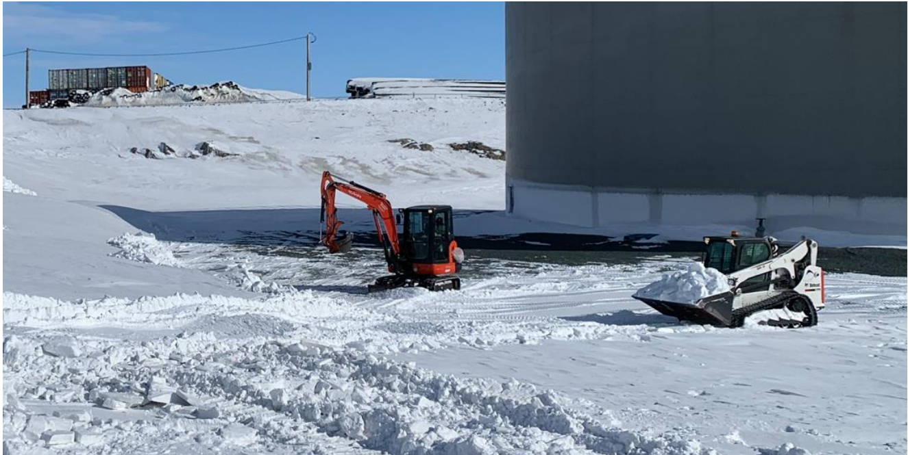
03-04-2024 Snow Removal Inside the Containment Area
