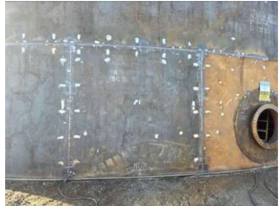
Picture 8 Door welds. Horizontal weld spot 6". Welds 1V/1V with 2V. Vertical bottom and middle welds spot 6".
