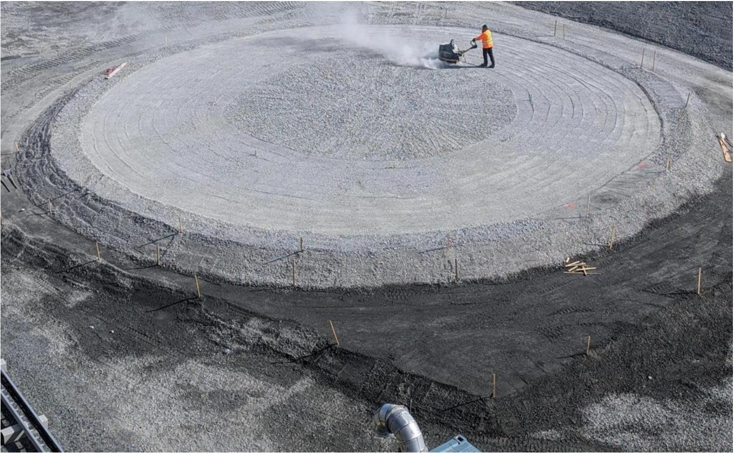
17-06-2024 Compaction of 30 mm minus on 4.5ML Tank Pad
