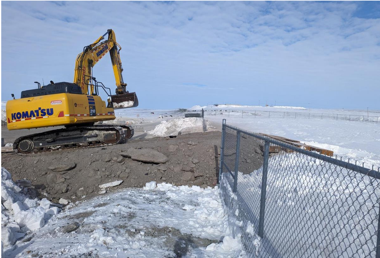
04-04-2024 Access Ramp on the West Side of the Containment, Rigmats Installed over the Dike
