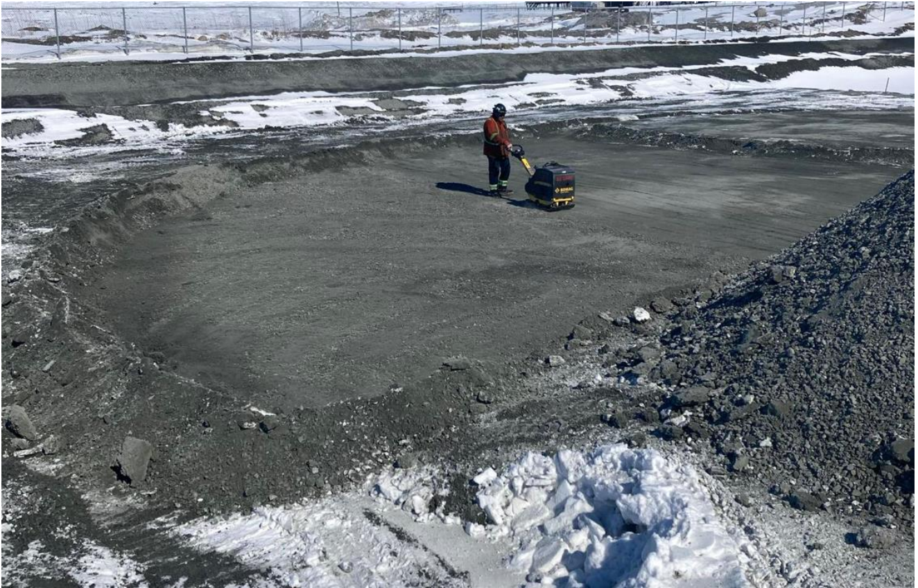
07-05-2024 Compacting 30 mm minus on 9ML Tank Pad with Vibratory Plate
