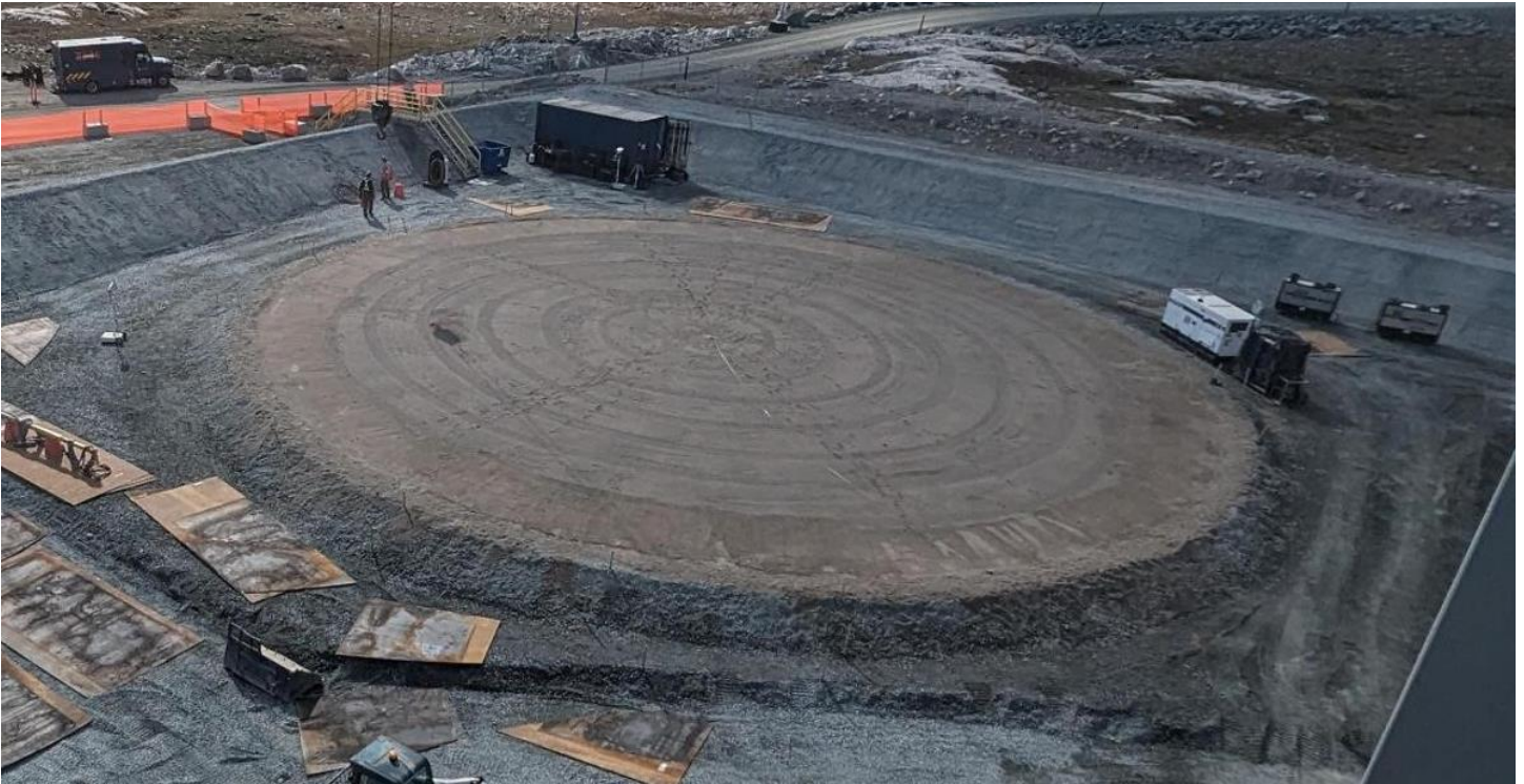
17-06-2024 9ML Tank Pad before Tank Erection
