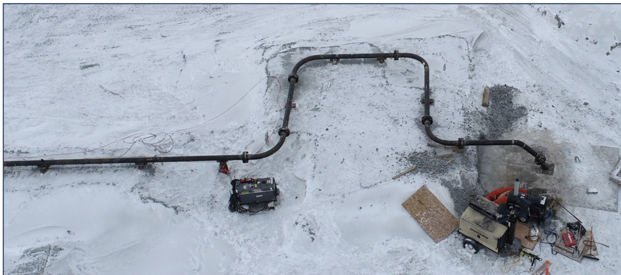
Figure 2 : Expansion loop and borehole connection
