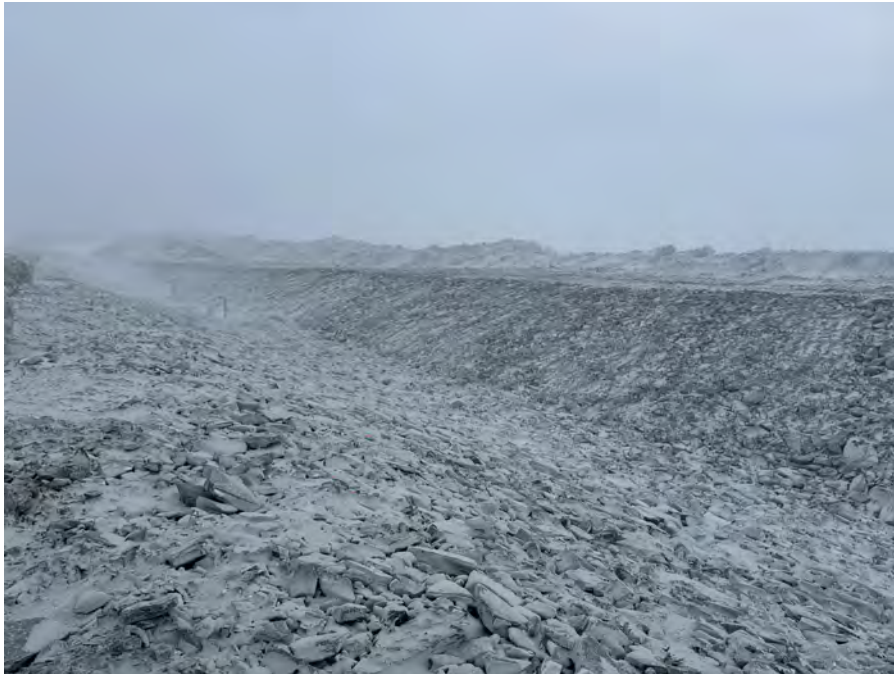
Photo 4: 2025-03-09 Channel11 — Completed Clean Rockfill Placement; Station 0+450 Facing Southwest
