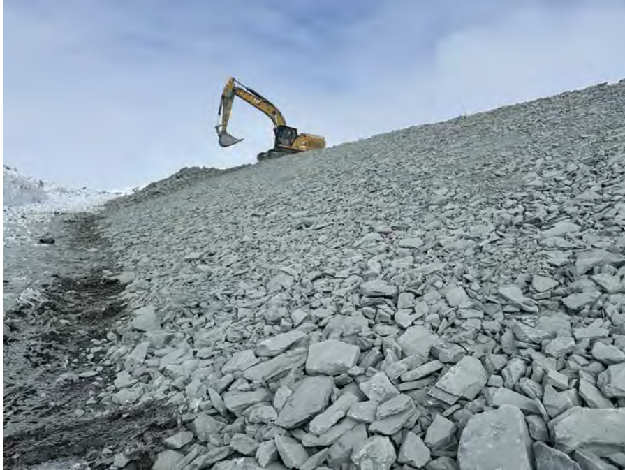
Photo 13: 2025-04-12 CP9 Thermal Berm — Clean Rockfill Sloping; Station 0+425 Facing North
