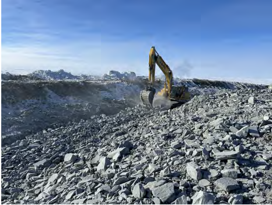
Photo 3: 2025-03-08 Channel11 — Clean Rockfill Placement Overview; Station 0+425 Facing North
