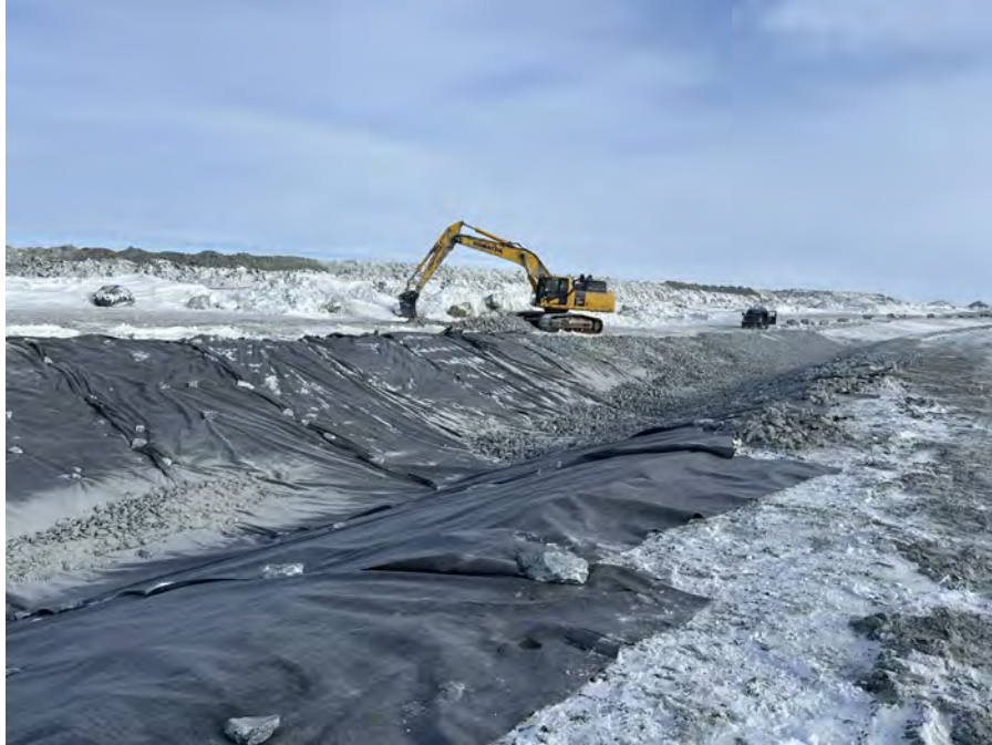
Photo 5: 2025-03-12 Channel11 — Placed Geotextile; Station 0+475 Facing Southeast
