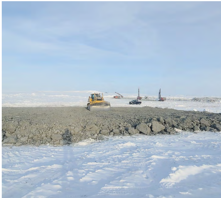
Photo 10: 2025-02-08 CP9 Thermal Berm — First Lift of Overburden Till; Facing North
