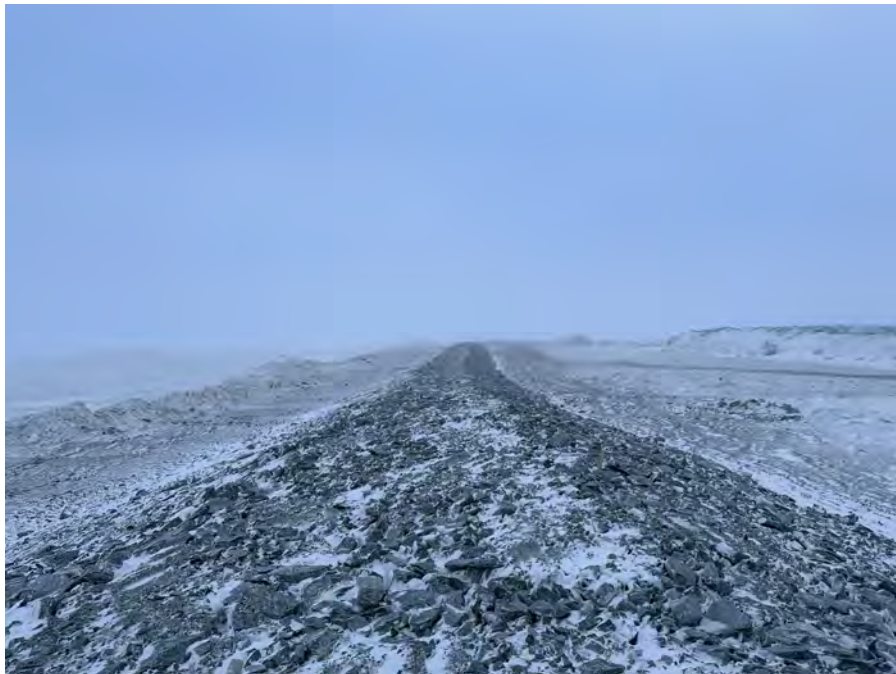
Photo 20: 2025-03-10 Berm4 — Overview of Sloped Clean Rockfill, Facing Southwest
