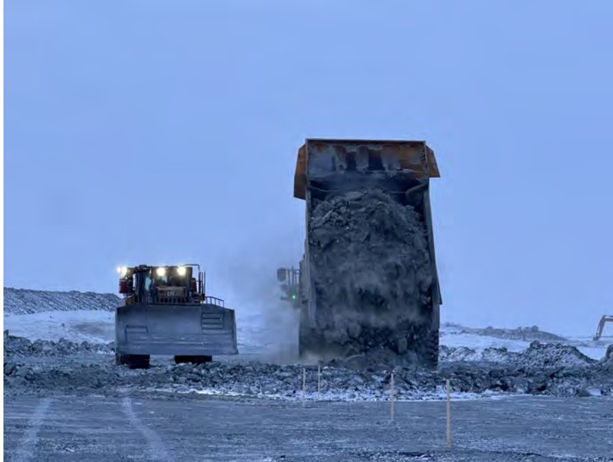
Photo 11: 2025-03-11 CP9 Thermal Berm — Overburden Till Placement Overview; Station 0+375 Facing Southwest
