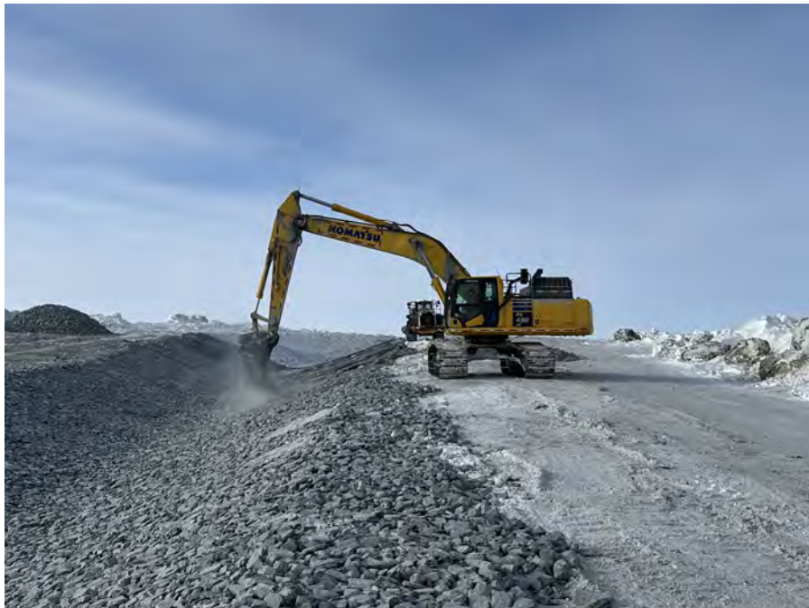
Photo 6: 2025-03-12 Channel11 — Rip-rap Placement; Station 0+415 Facing North
