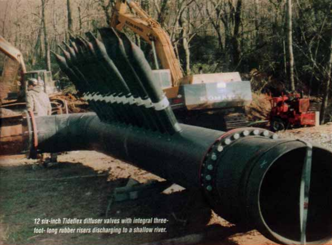
A 30° orientation from the horizontal discharge angle enhances dilution from this pulp mill diffuser.
