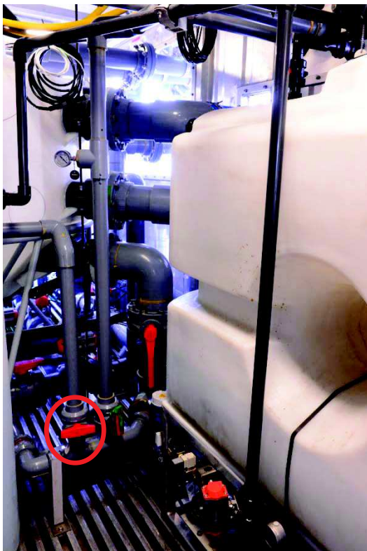
Figure B4: MBV2-224-19 Valve Location
