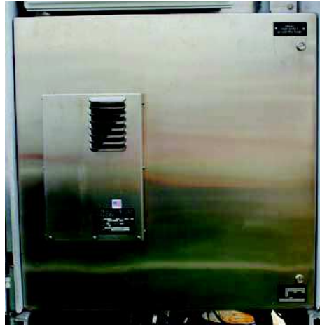
Figure 17: AC VFD Pump Panel
