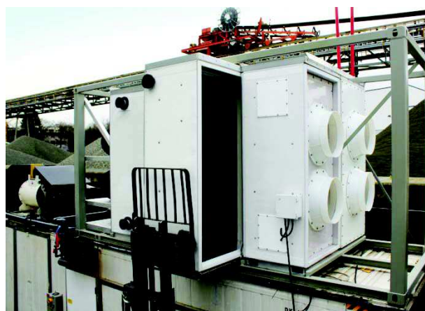
Figure 8: Module Removal by Forklift
