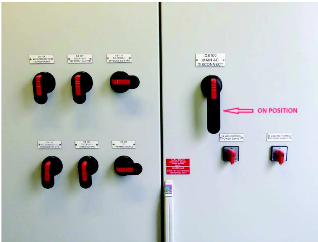
Figure 31: Main disconnect in ON Position
