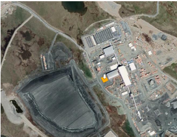
Figure 1. Temporary Storage Pad for Tailings
