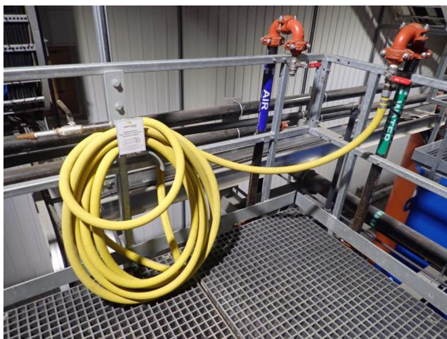
Figure 2: Zoom in image of the EWTP and photos of the MEL-14 sampling port inside the building (end of the yellow hose).
