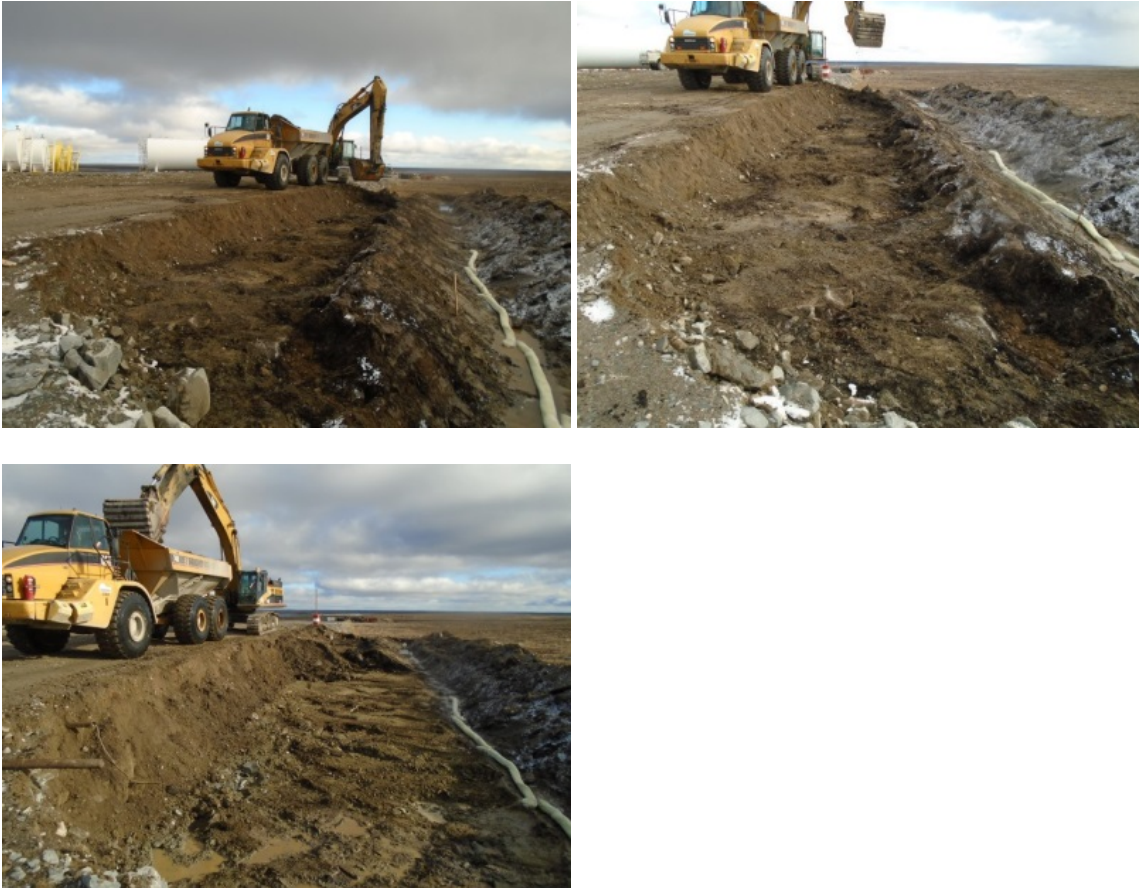
Figure 6 – Contaminated soil excavation
