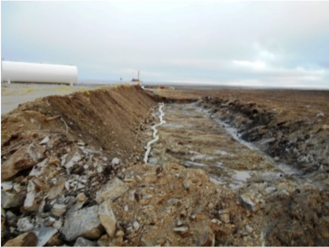
Figure 7 - All contaminated soil removed from the trench up to the road shoulder
