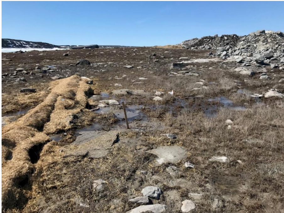
Picture 1: Straw log sediment trap between Bypass Road entrance at Itivia and Melvin Bay.
