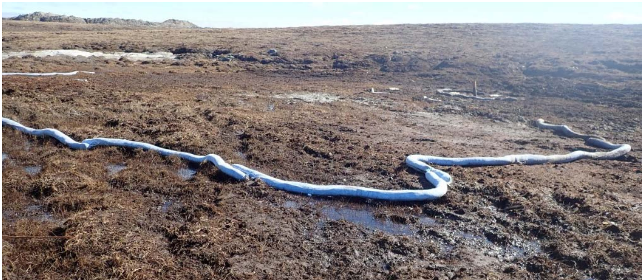
Figure 1: Booms placed downstream of spill location.
