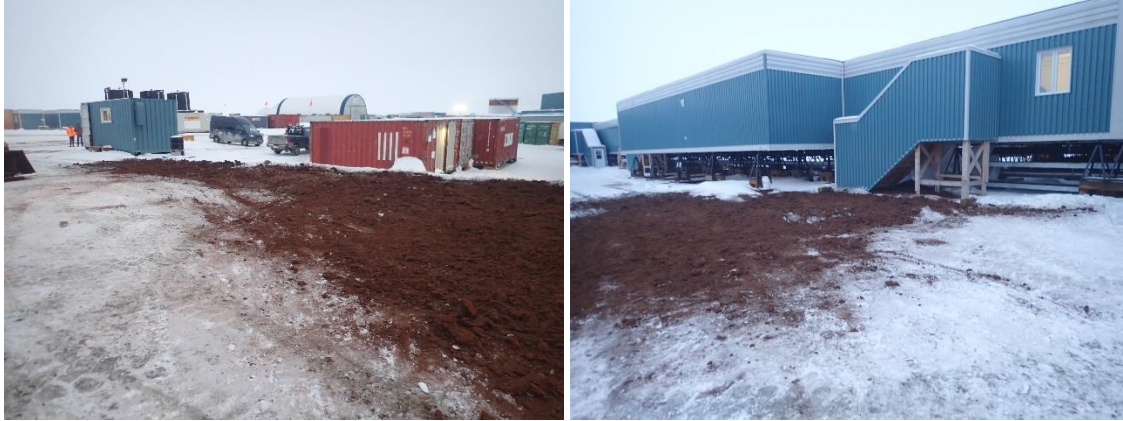
Photo 2: Peat moss applied to contaminated area to absorb material.
