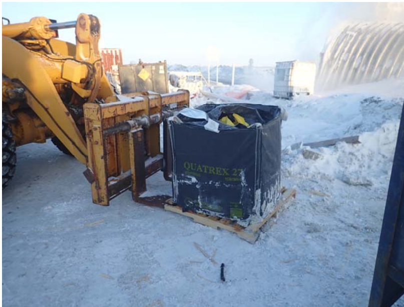
Figure 3: Snow contaminated with emulsion residue disposed of as hazmat.
