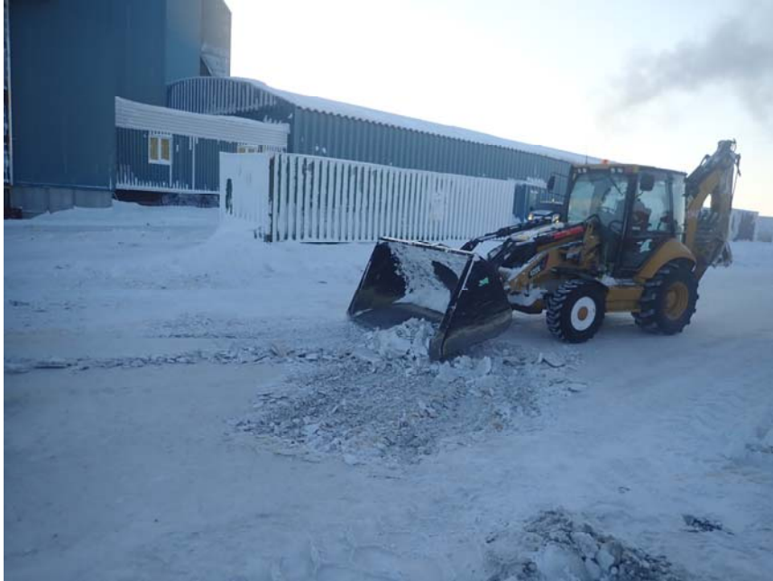
Figure 1: Water from boiler recirculation system being removed from ground.
