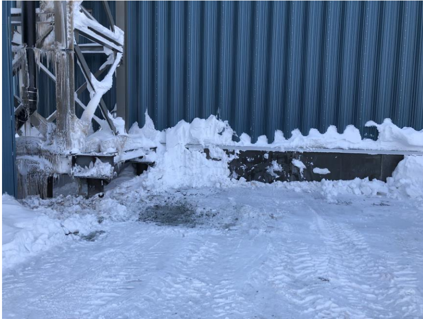
Figure 2: Area of contaminated snow removed and brought to the Meliadine Landfarm; contaminated ice will be collected when ice melts to prevent structural damage with equipment
